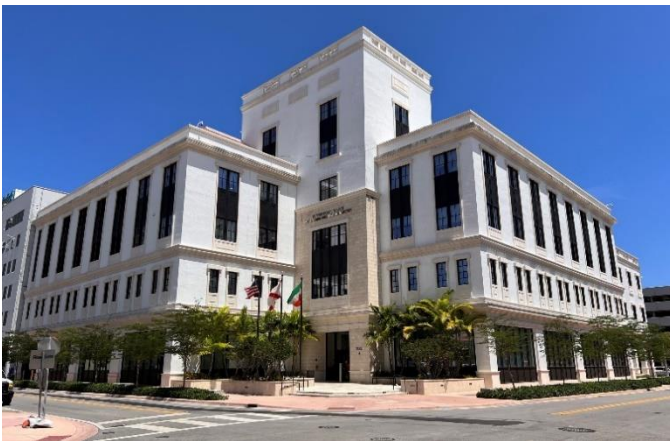
Police & Fire Headquarters
