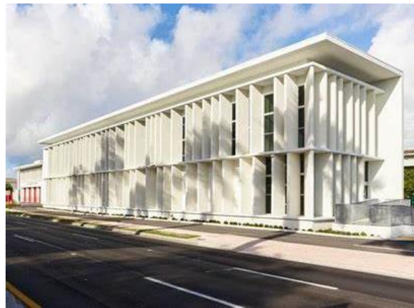
Trolley Maintenance Facility
