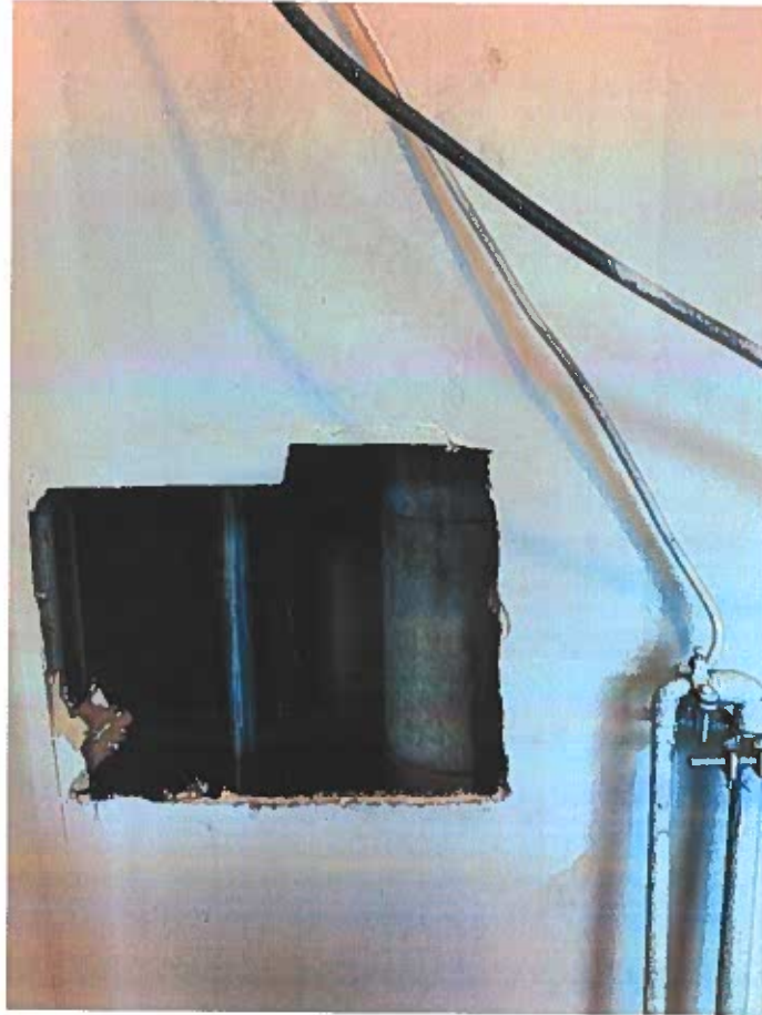
Opening in ceiling and walls inside electrical room from 2 nd -7 th floor
