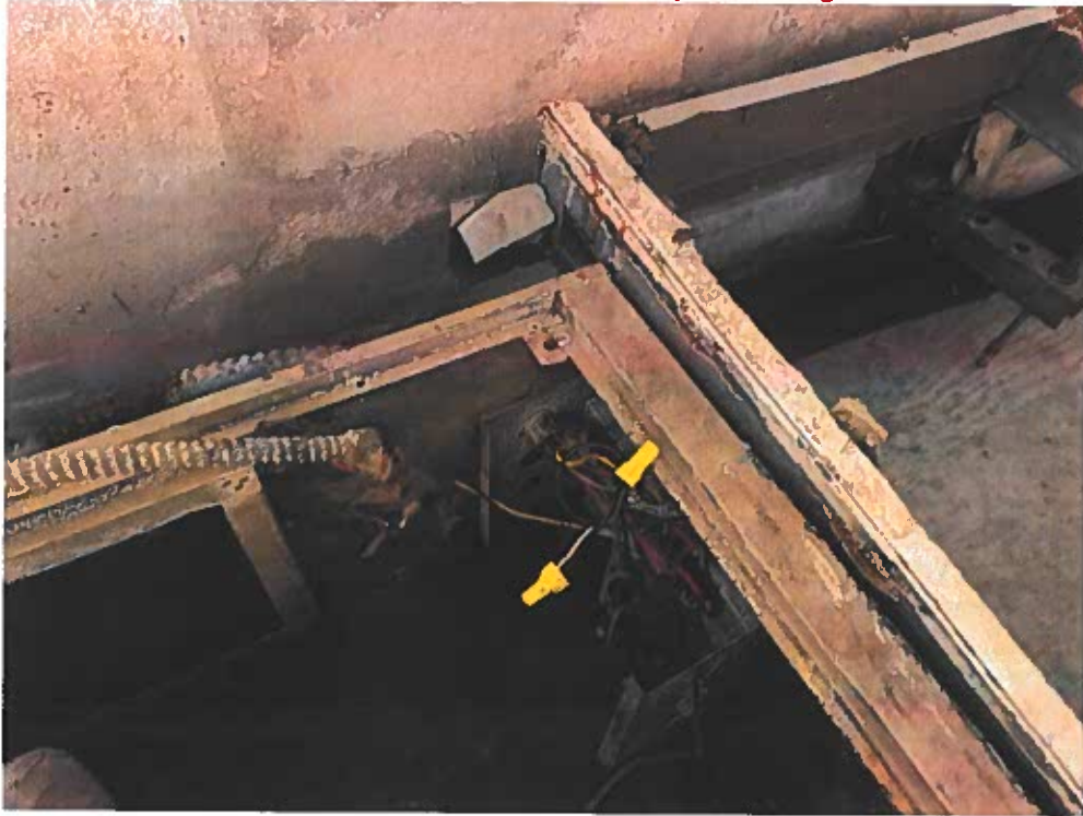
Exposed wires, missing cover in electrical boxes
