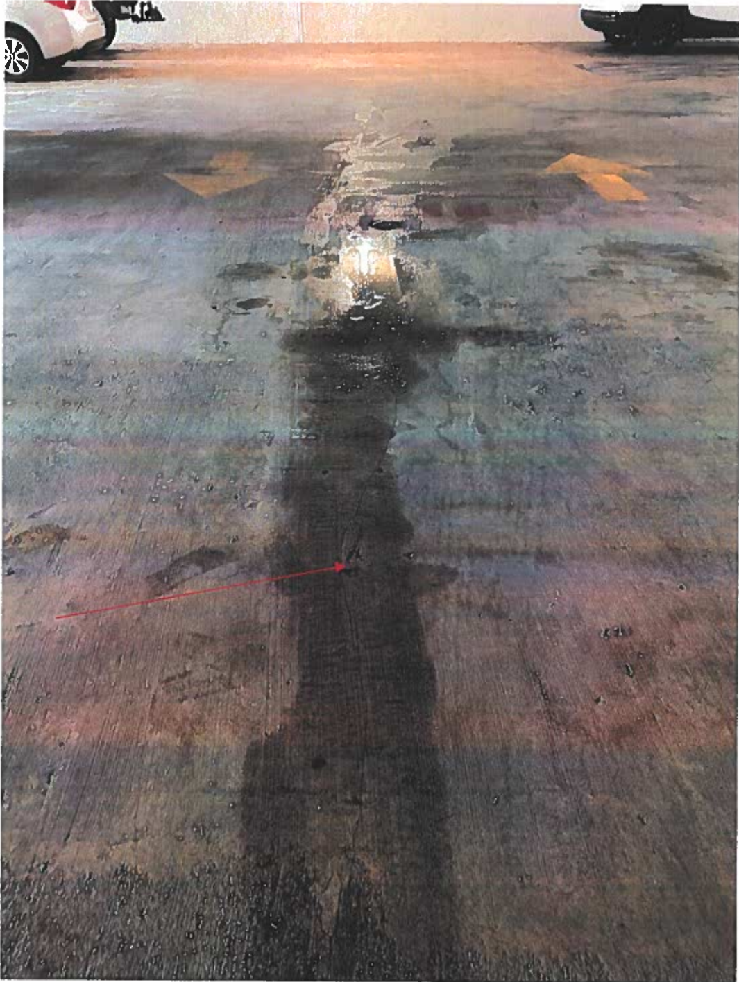
Fine crack in 2 nd floor slab with water penetration through basement
