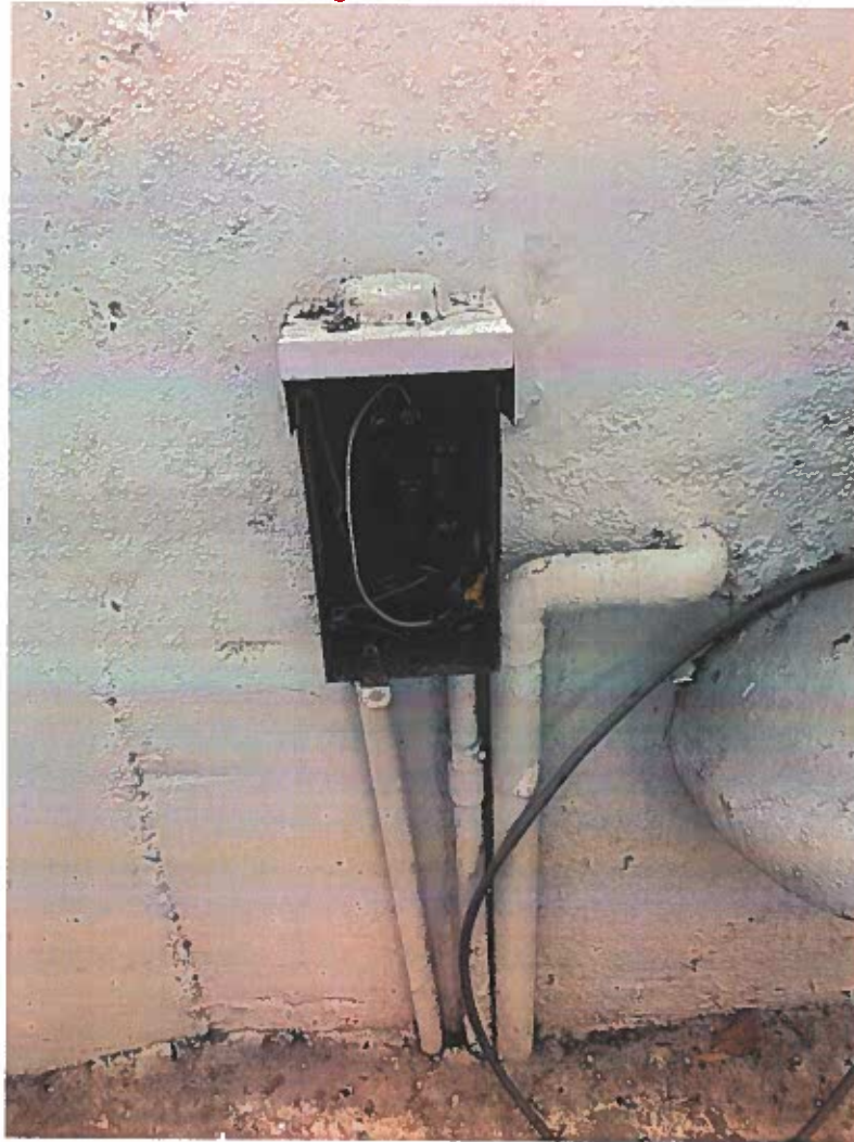
Missing cover in electrical box
