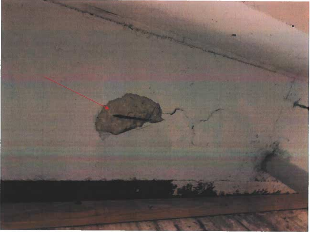
Deteriorated concrete spall
