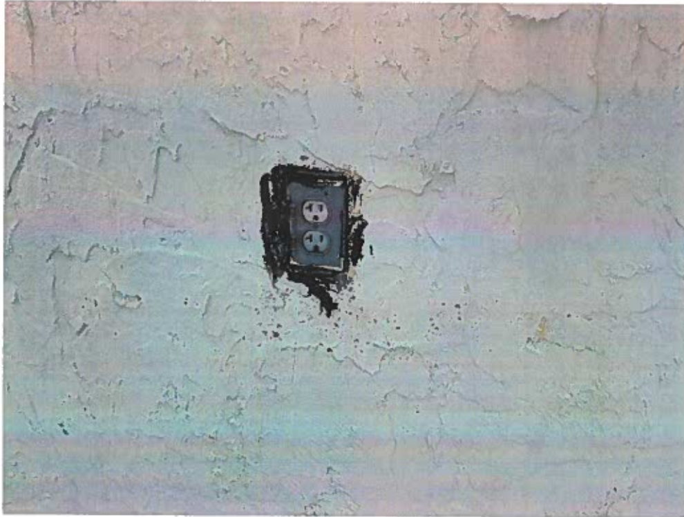
Missing waterproof cover in exterior receptacle in roof
