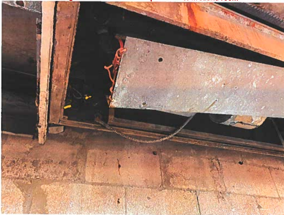
Damaged interior walls and exposed wires in sauna room
