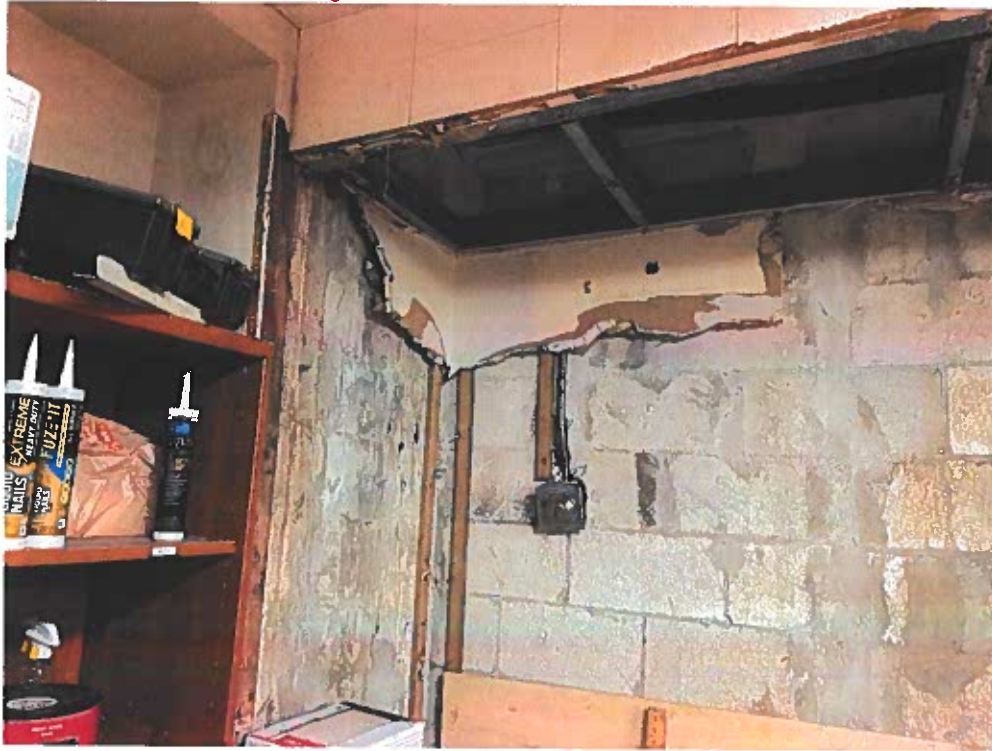
Damaged interior walls and exposed wires in sauna room
