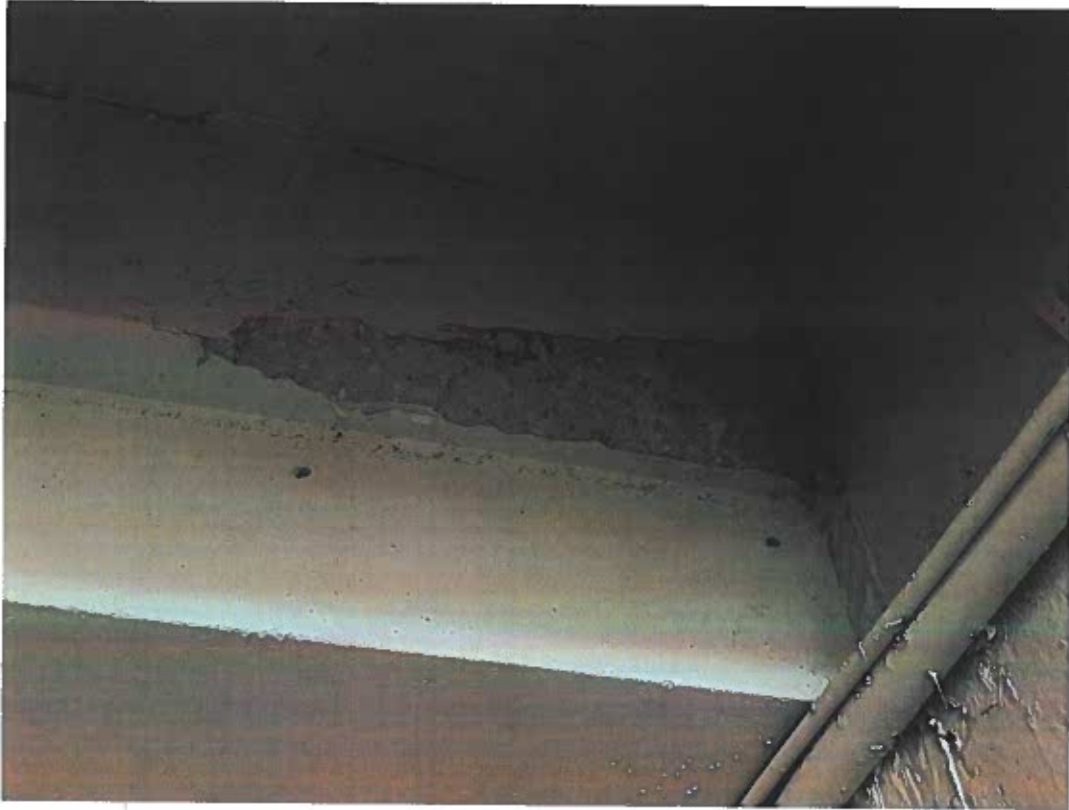
Concrete spall in many location
