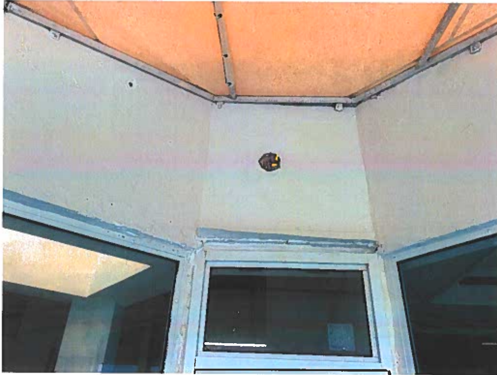
Exposed wires in management office balcony
