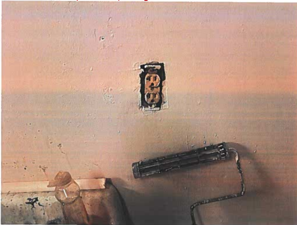
Exposed wires, missing cover in electrical boxes
