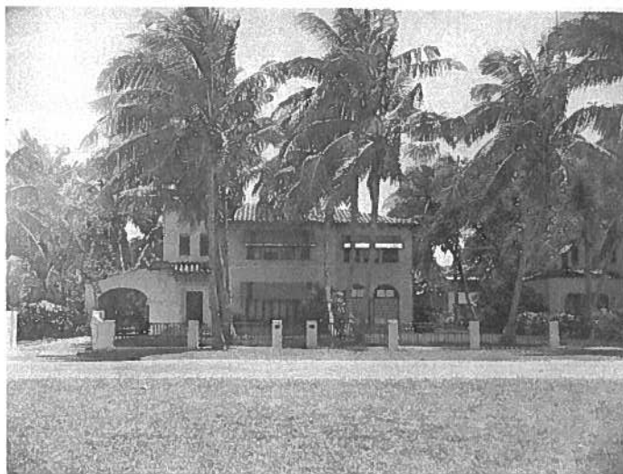
Fig. 1 1940s photograph of front facade
