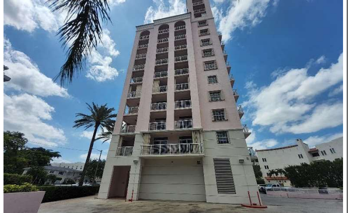
Photo # 2. East building elevation.
