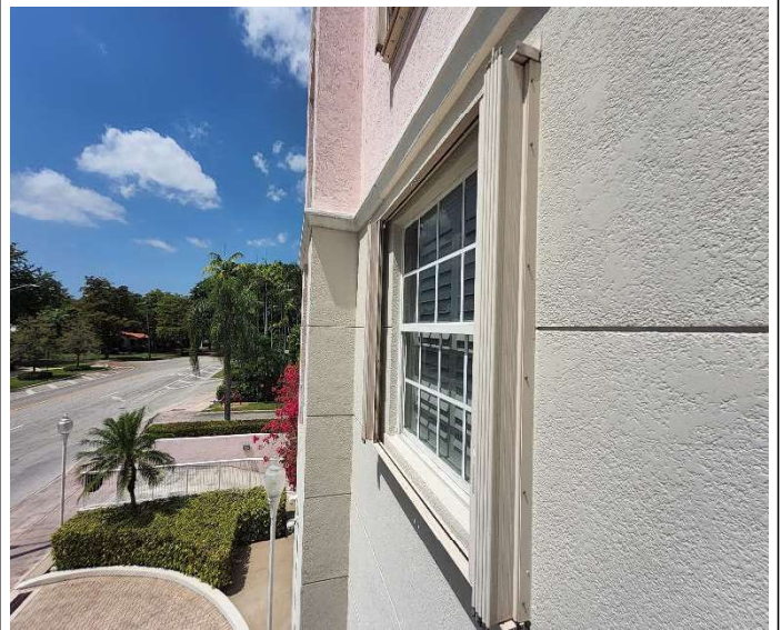
Photo # 12. Typical window.
