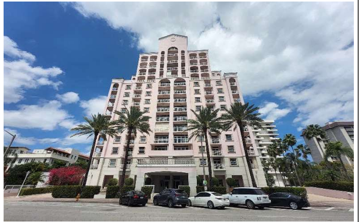
Photo # 4. South building elevation.
