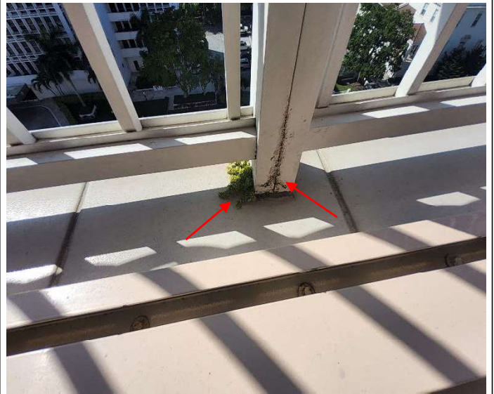
Photo # 32. Biological growth and pitting corrosion at the balcony railing post.
