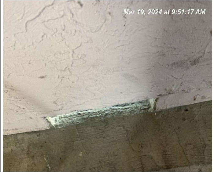
Photo # 14. Primary scupper at the lower roof.
