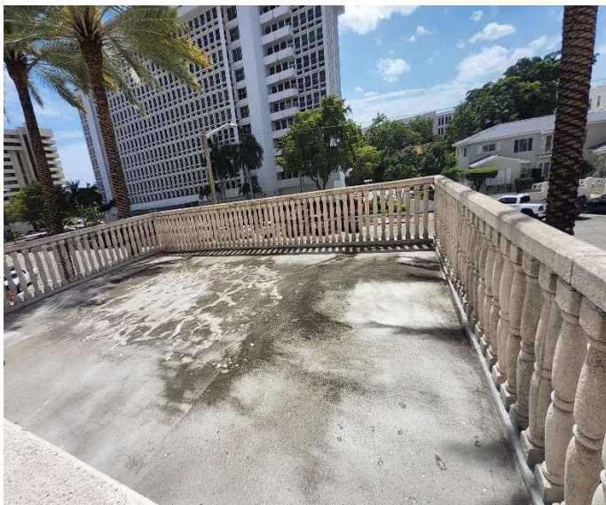
Photo # 7. Porte-cochere roof with bitumen membrane roofing system.
