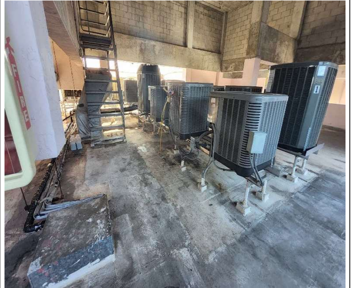
Photo # 6. Lower roof with TPO membrane roofing system.
