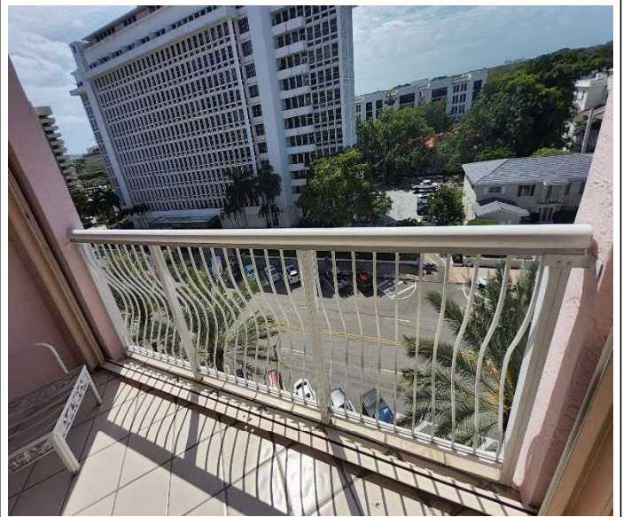
Photo # 10. Balcony railing.
