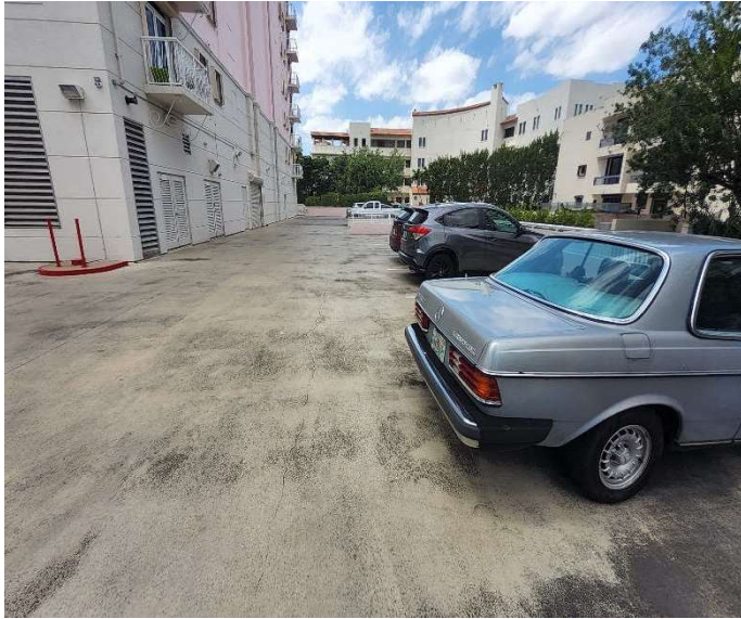
Photo # 17. Garage deck.
