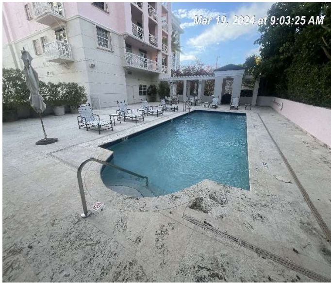
Photo # 9. Pool and pool deck.
