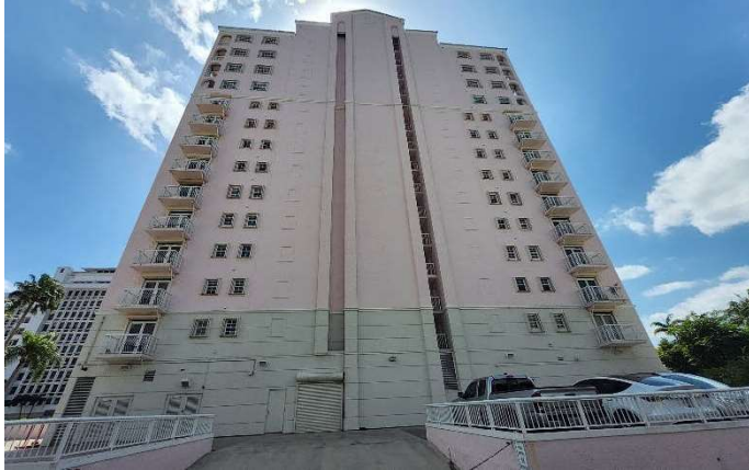
Photo # 1. North building elevation.
