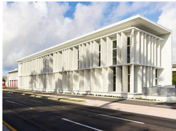
Trolley Maintenance Facility
