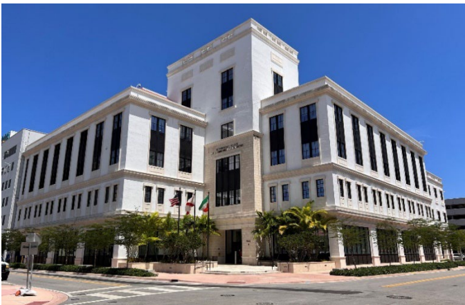
Police & Fire Headquarters
