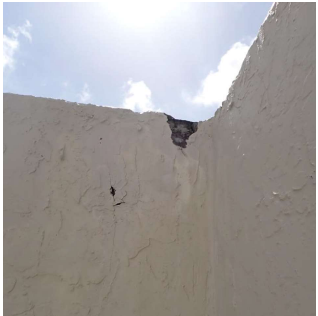
Photo # 65 Closeup of Photo # 64
