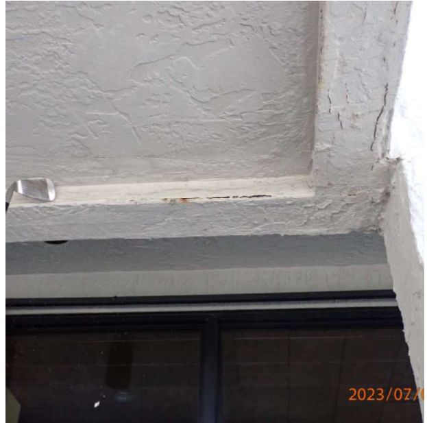
Photo # 8 Closeup of Photo # 7
