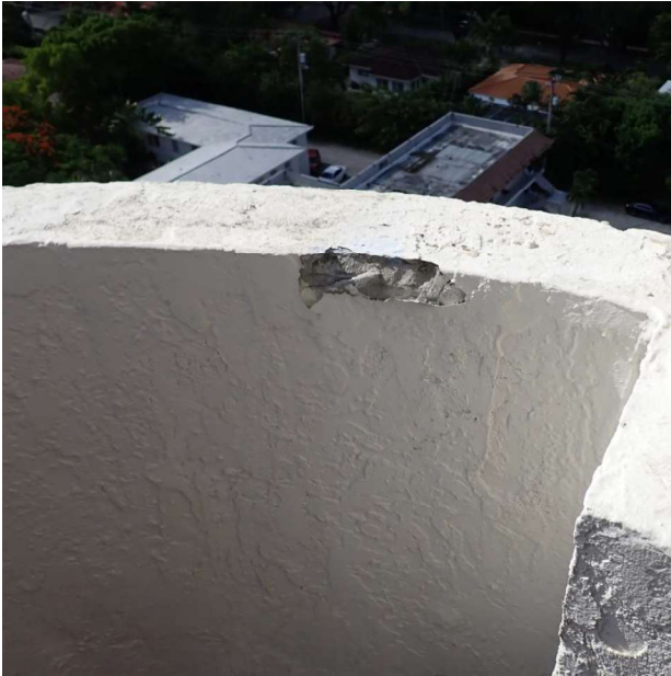
Photo # 45 Corroded column at penthouse
