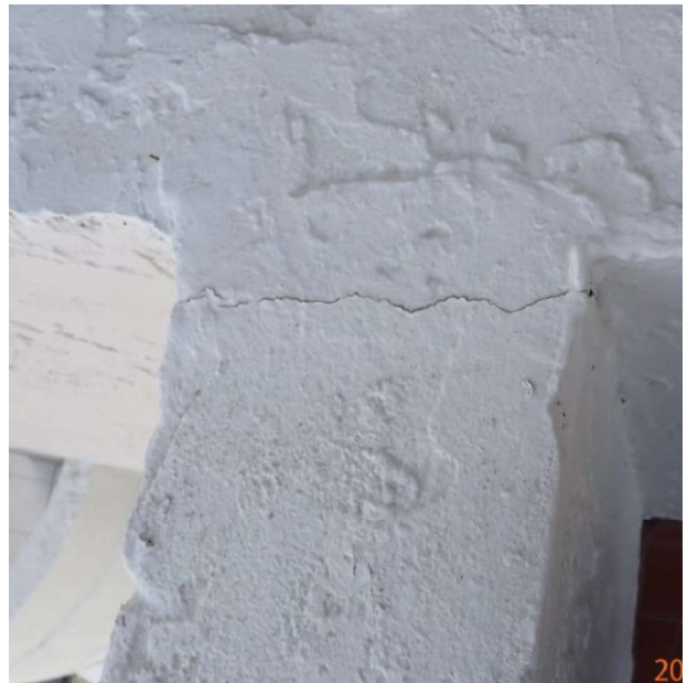
Photo # 30 Closeup of Photo # 29
