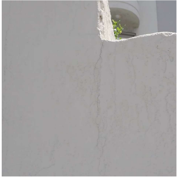
Photo # 4 Closeup of Photo # 3
