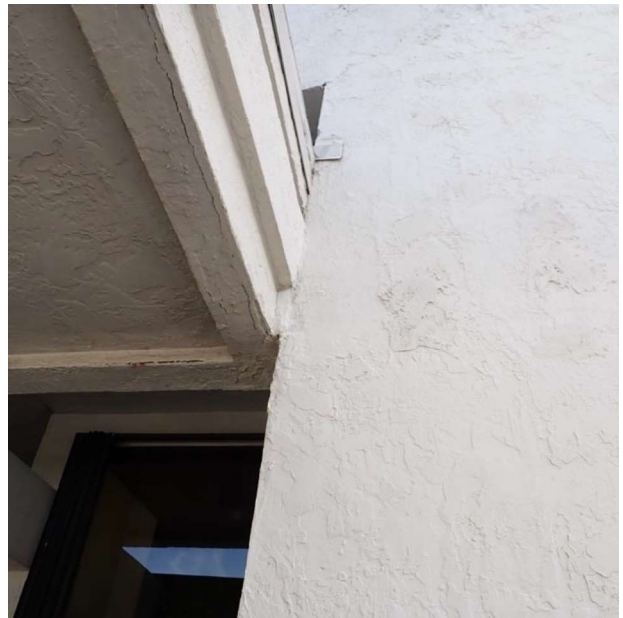
Photo # 10 Closeup of Photo # 7
