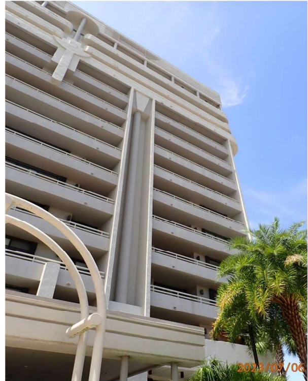
Photo # 6 South Building Elevation
