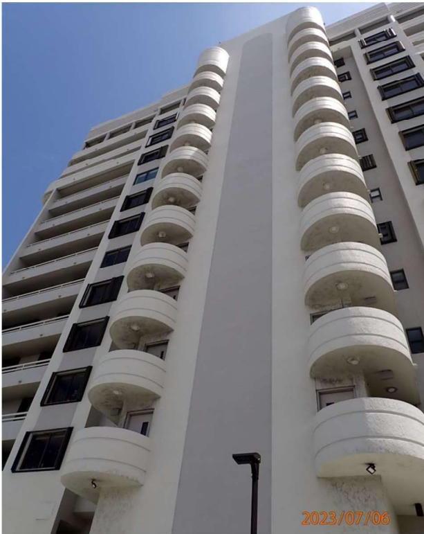
Photo # 3 North Building Elevation
