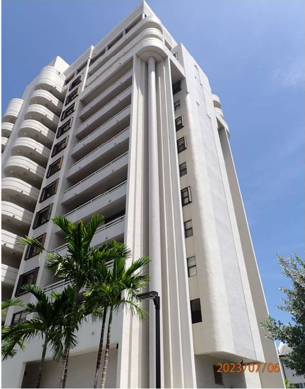
Photo # 1 NW Building Elevation
