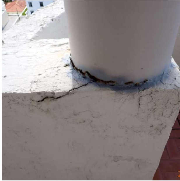
Photo # 24 Closeup of Photo # 23
