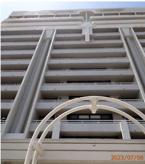
Photo # 7 South Building Elevation
