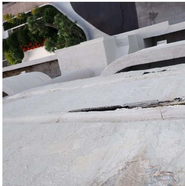
Photo # 18 Closeup of Photo # 17
