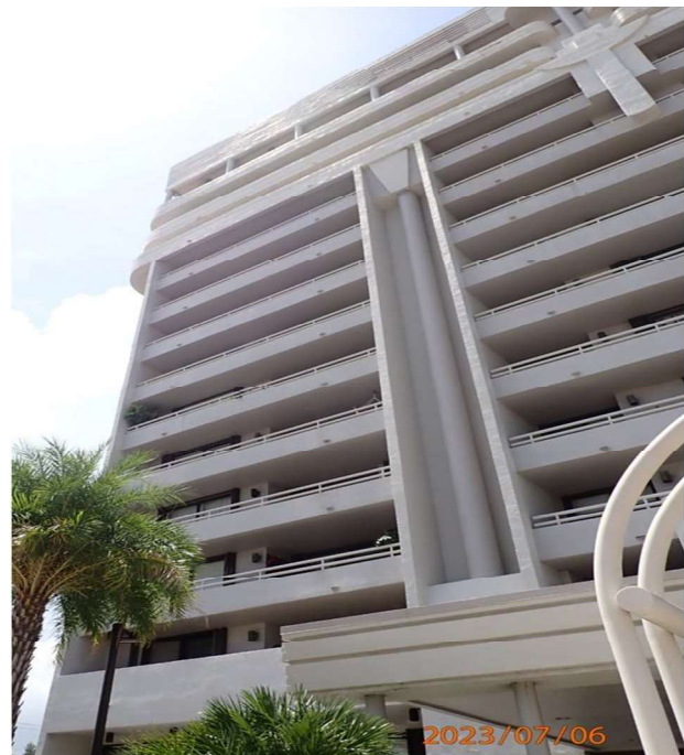
Photo # 8 South Building Elevation
