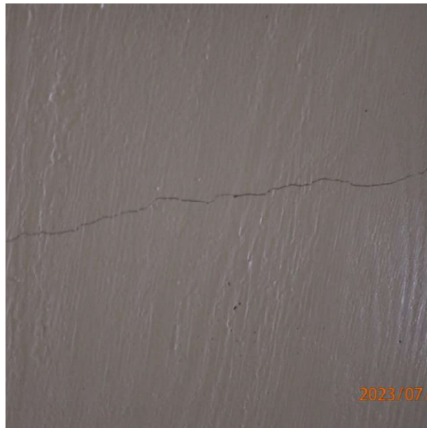
Photo # 67 Closeup of Photo # 66
