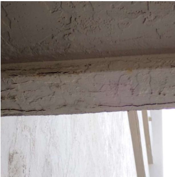
Photo # 9 Closeup of Photo # 7
