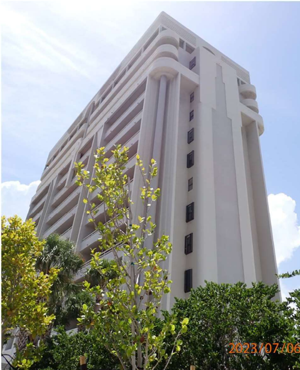
Photo # 5 SE Building Elevation
