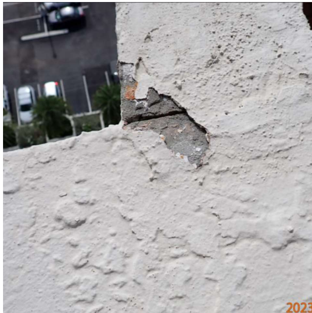
Photo # 26 Closeup of Photo # 25
