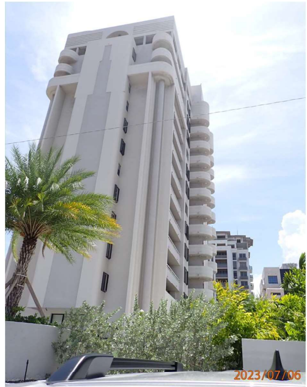
Photo # 4 East Building Elevation
