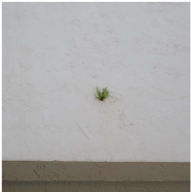
Photo # 6 Closeup of Photo # 5
