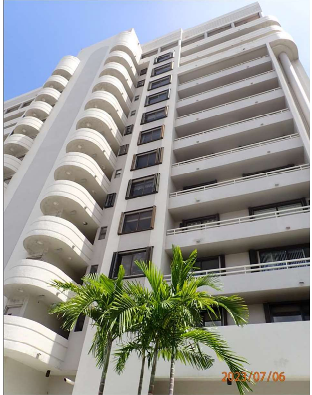
Photo # 2 North Building Elevation
