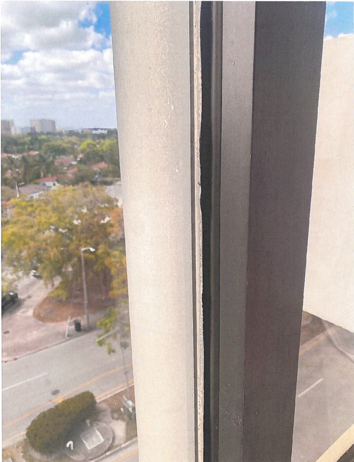
Typical interior seals at window system
