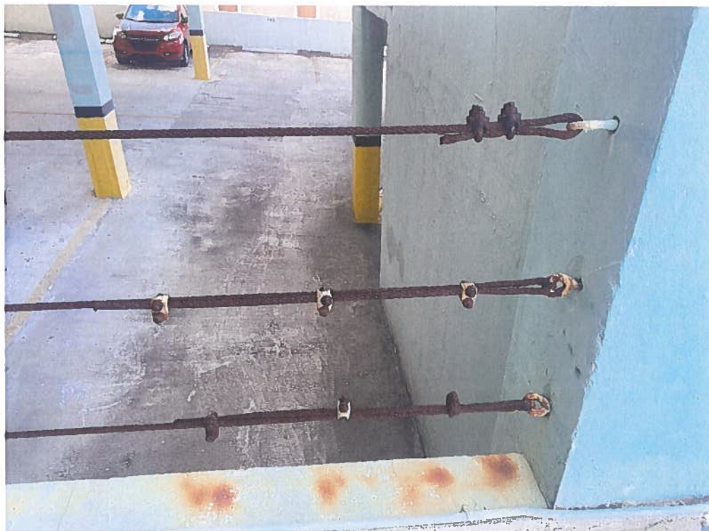
Excessive corrosion observed on barrier cables
