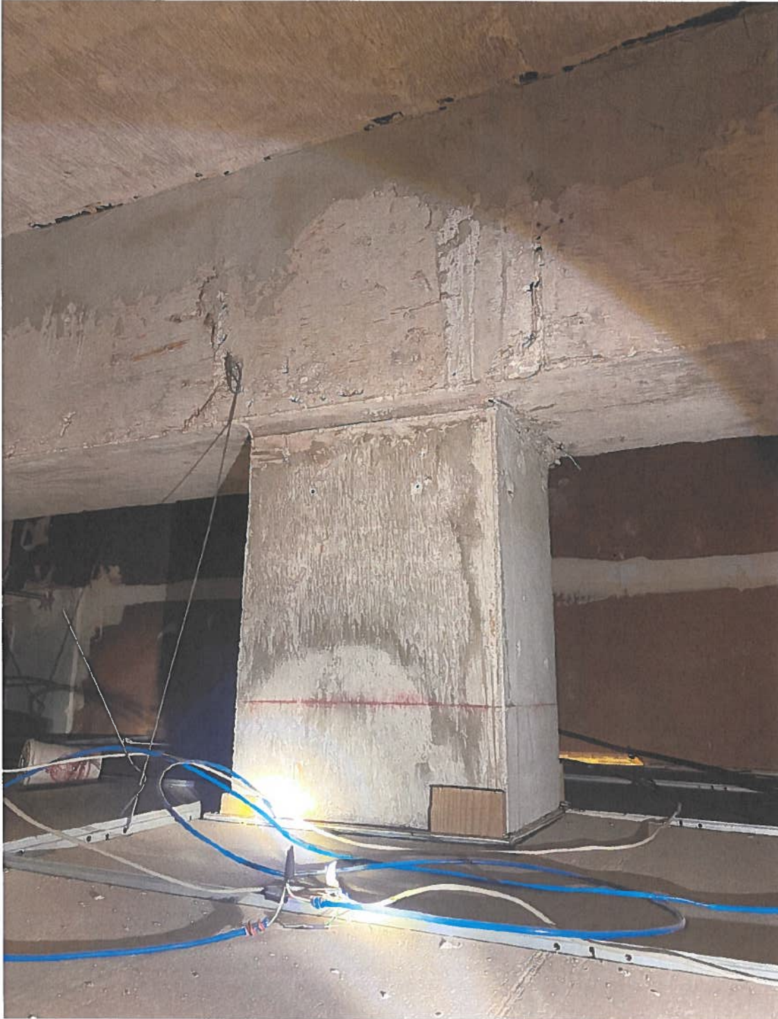
Typical interior concrete column/beam connection
