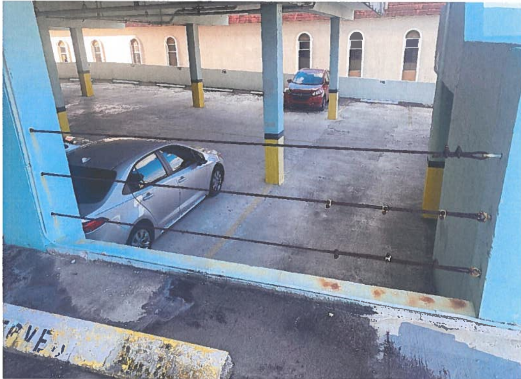
The steel barrier cables at Parking Garage needs replacement
