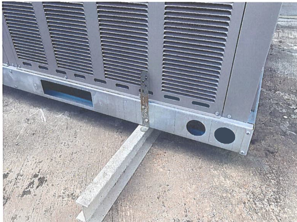
RTU attachment to aluminum frames
