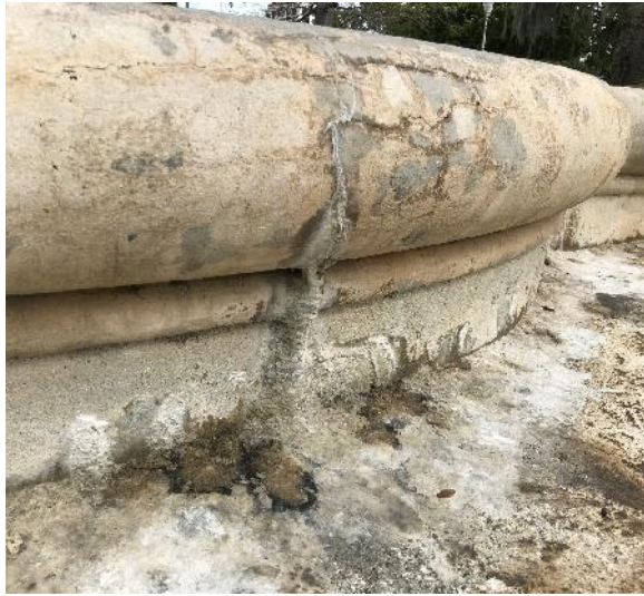
Figure 4. Detail of the typical mineral accretions on the outside of the concrete basin (photo by EverGreene, February 2021).
