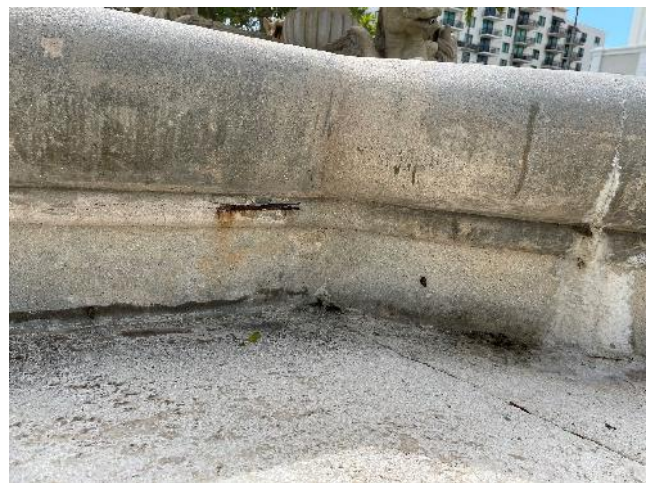
Figure 7. Corroded ferrous metal resulted in damage and loss in concrete (photo by EverGreene, February 2021).
