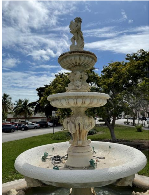
Figure 13. Lighting hardware in lower basin, no water has collected in the lower basin (photo by EverGreene, February 2021).
