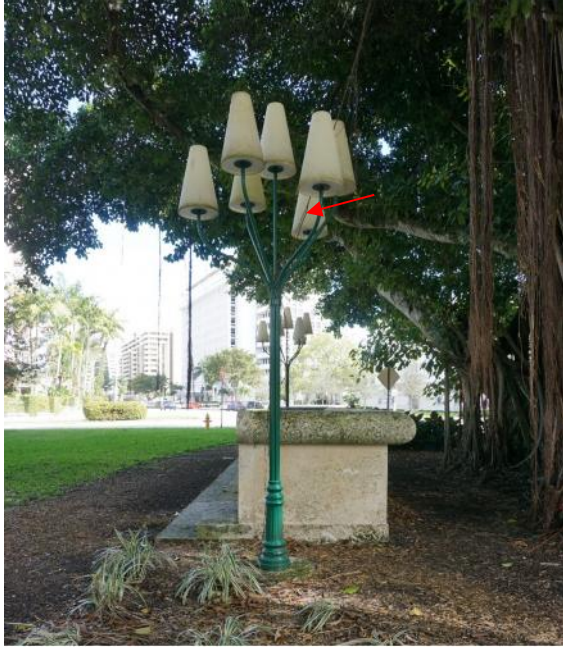
Figure 1. Northwest lamp and northwest side of bench; red arrow points to the vine that has entered the lamp structure (photo by EverGreene, February 2021).
