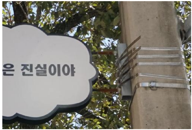
Figure 3. T: The Truth is I Remember You, two corroded threaded rods (photo by EverGreene, February 2021).
