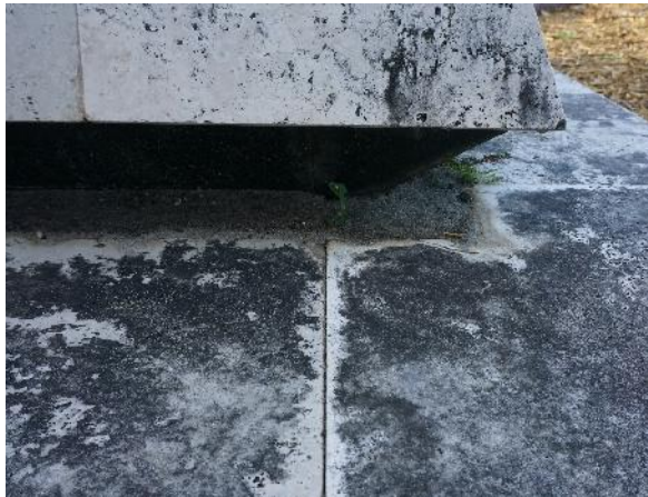
Figure 7. Soiling accumulation under pyramid with plant growth; soiling on marble pavers (photo by EverGreene, February 2021).
