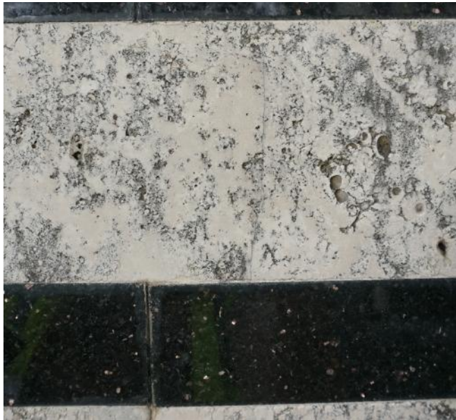
Figure 5. Mortar loss in granite joint, crack in marble (photo by EverGreene, February 2021).
