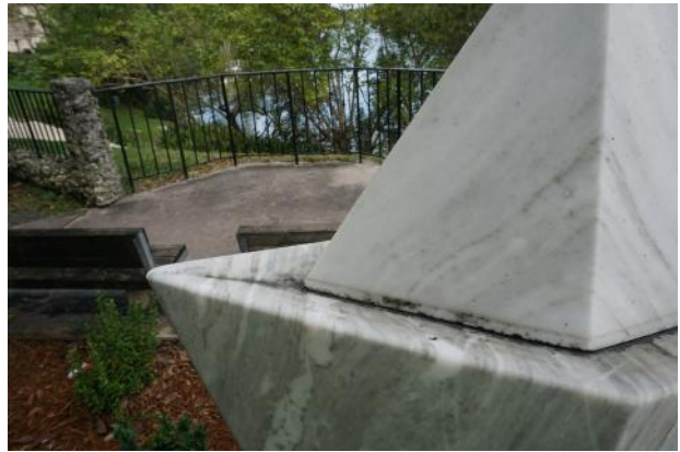
Figure 4. Detail of soiling accumulation on top of marble sculpture where rainwater pools (photo by EverGreene, February 2021).
