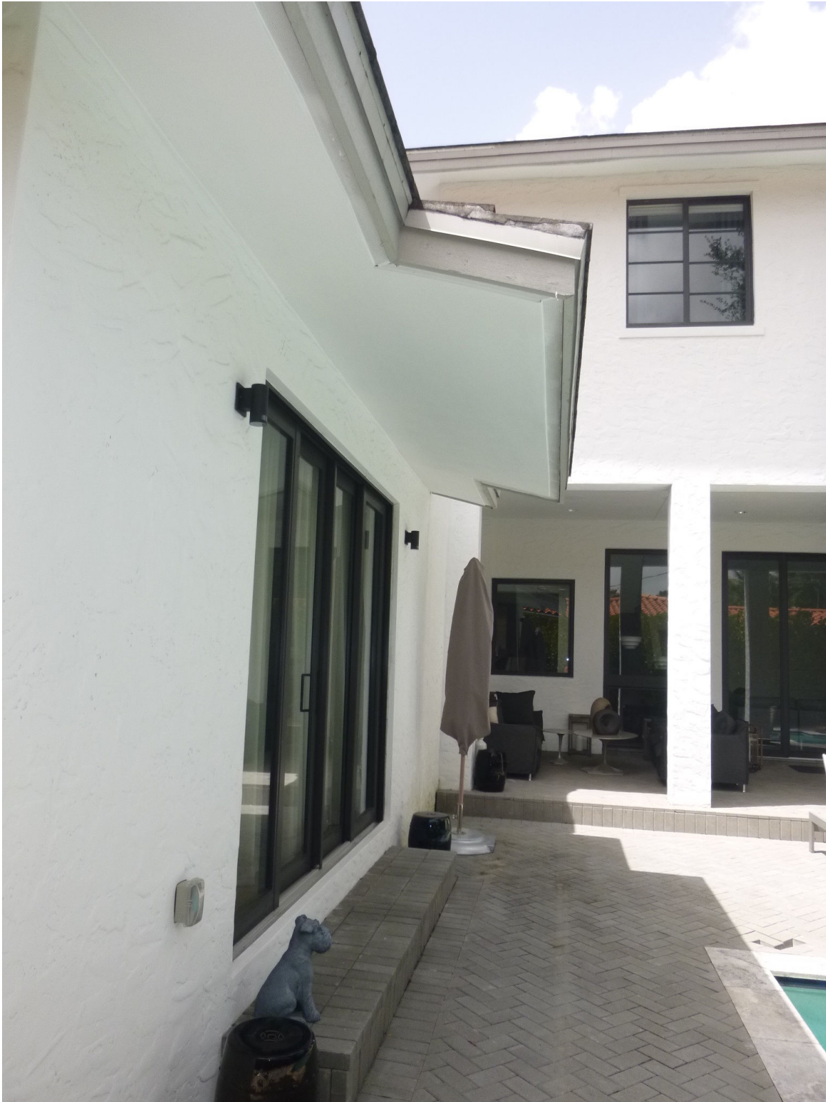
#10 - Existing Extended overhang North Elev. at pool area Extended overhang to be trimmed back in line with main o.h.
