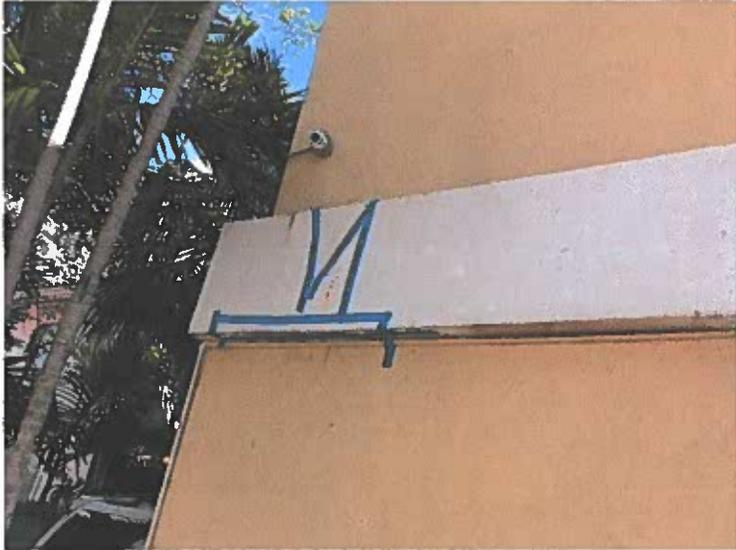
**Beam Spall at 2<sup>nd</sup> Floor West Main Elevation**
