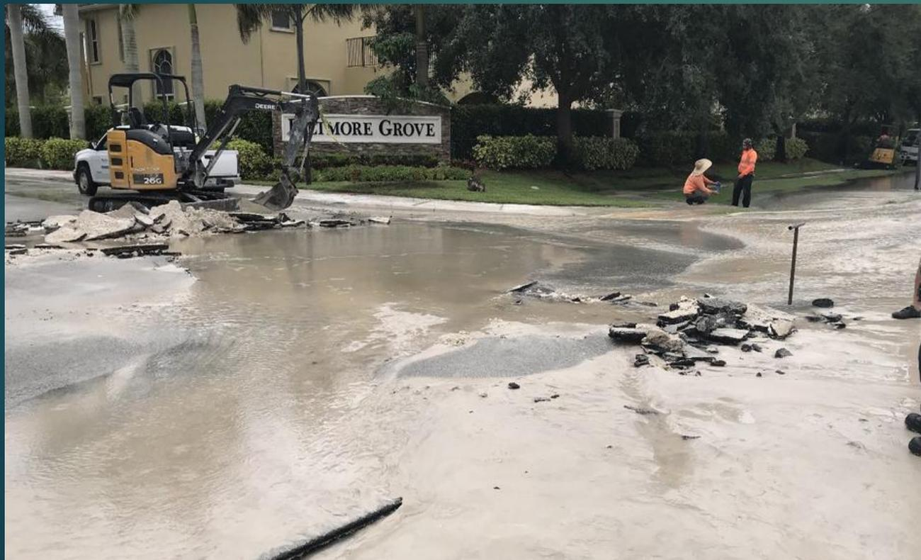
May 12, 2018, contractor for a wireless carrier installing fiber via directional bore struck a water main, which caused a flood and the road collapsed, creating a sink hole which blocked the entrance to a neighborhood in Cooper City. (Sun Sentinel picture)
