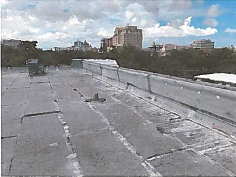
Roof & Parapet Wall
