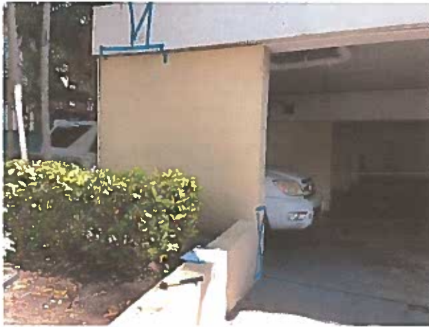
West Ground Floor Garage Entrance Beam Repair
