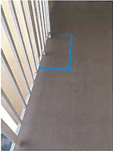
4 th Floor catwalk Spalls
