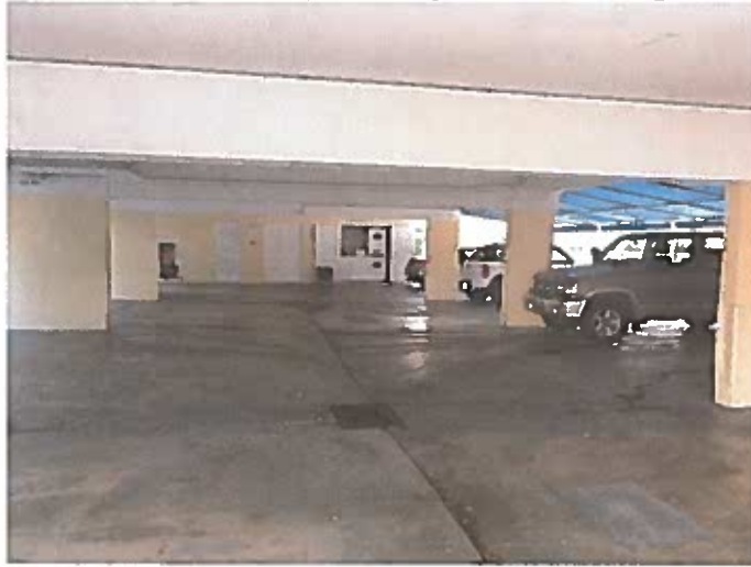
Garage at Ground Floor
