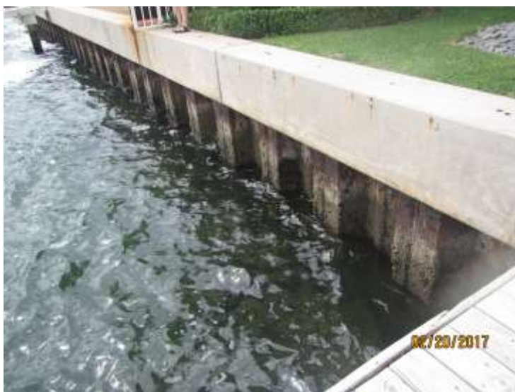
View of sheetpile seawall
