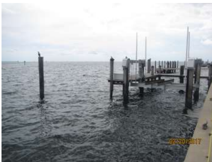
View of wood dock, boatlift, and mooring piles.
