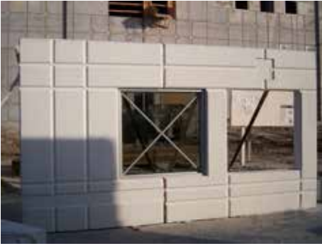
Weitz built and water-tested this mock-up before installing the window system in the South County Courthouse Expansion project in Delray Beach, Florida.
