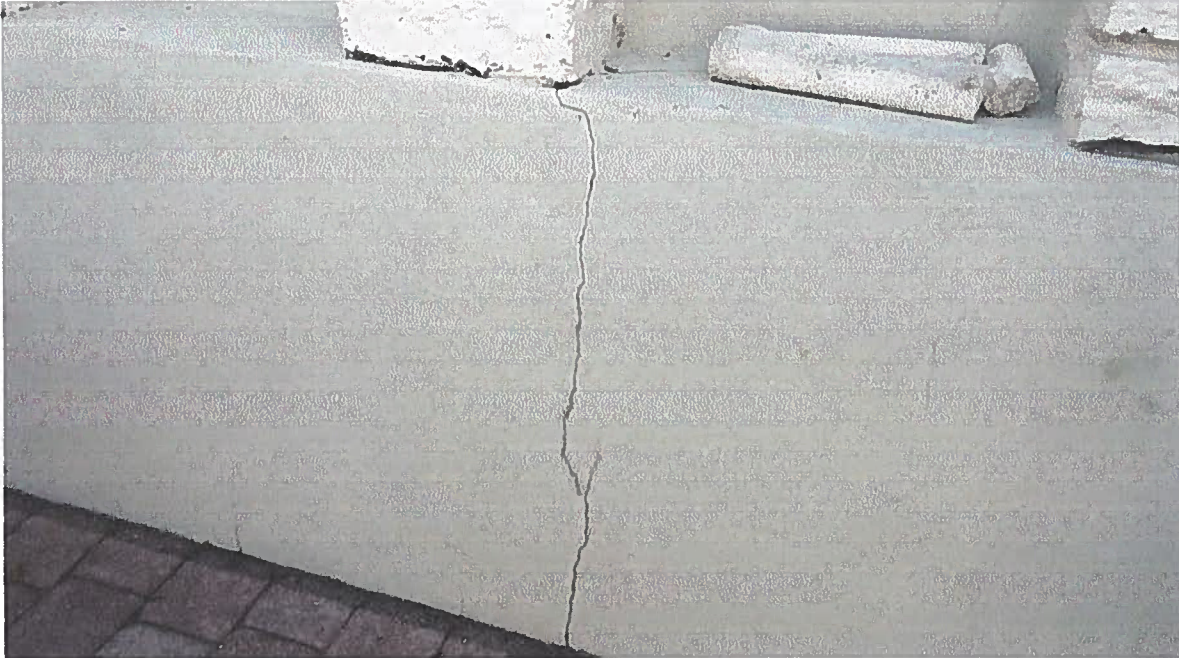
TYPICAL CRACKS FOUND IN EXTERIOR WALLS (SEVERAL WERE VISIBLE).
