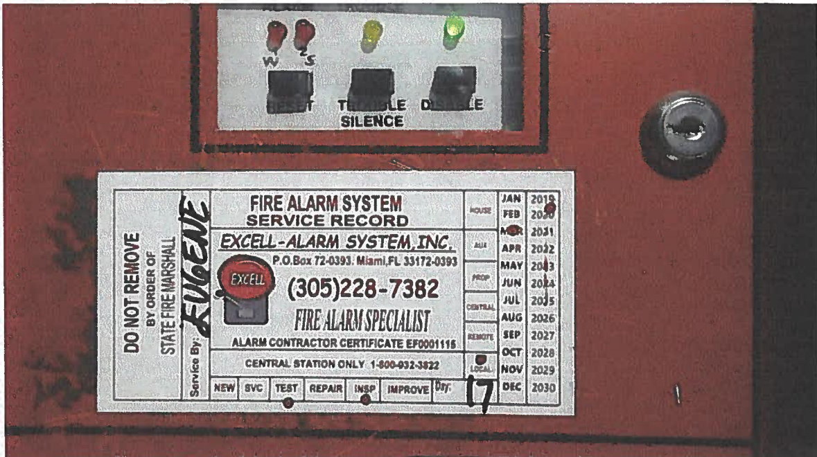
FIRE ALARM PANEL WITH ANNUAL INSPECTION PAST DUE (AS PER TAG, LAST INSPECTION WAS PERFORMED ON MARCH, 2020).
