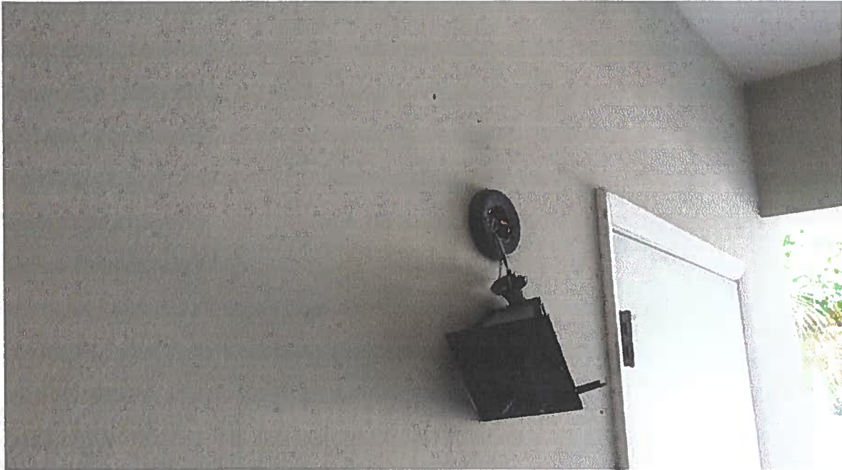
EXPOSED WIRES DUE TO BROKEN LAMP.
