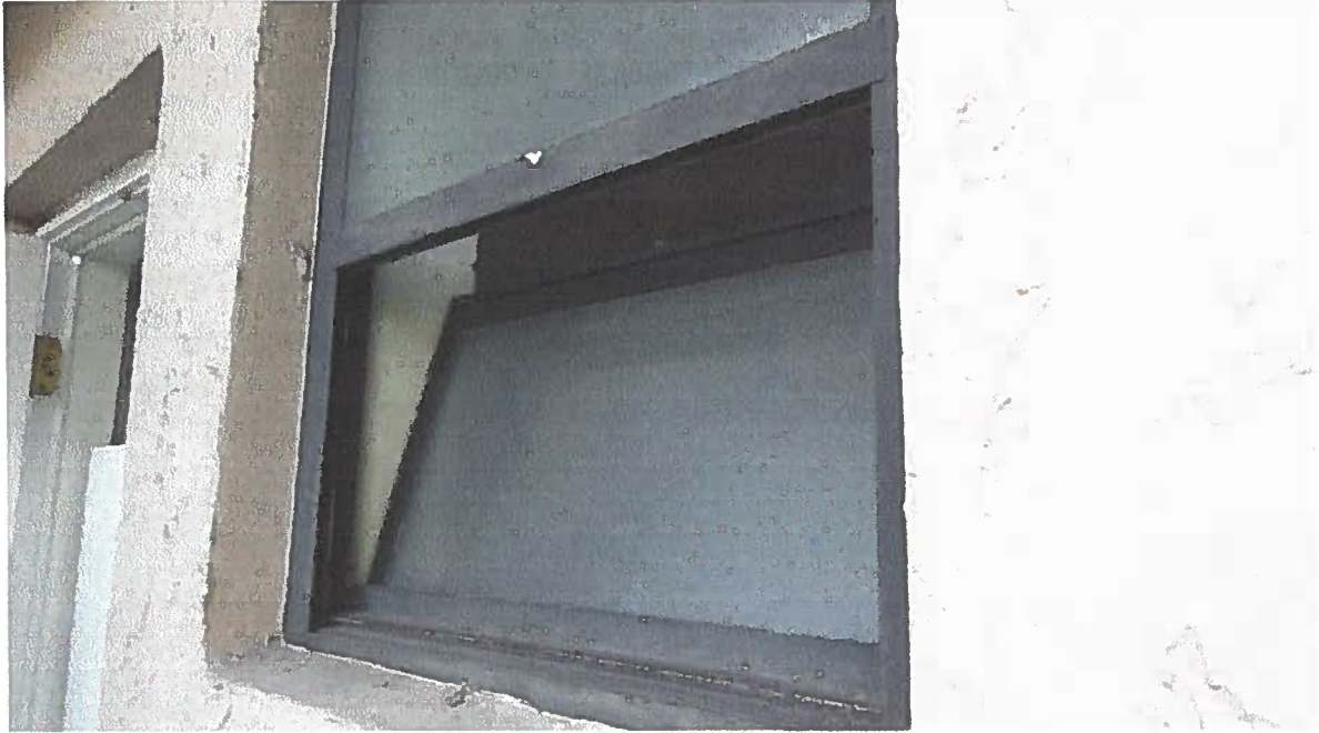
LOOSE WINDOW OF STORAGE MUST BE RE-INSTALLED.
