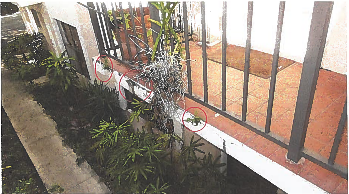
PLANTS GROWING IN SLAB MUST BE REMOVED AND CRACK MUST BE REPAIRED.
