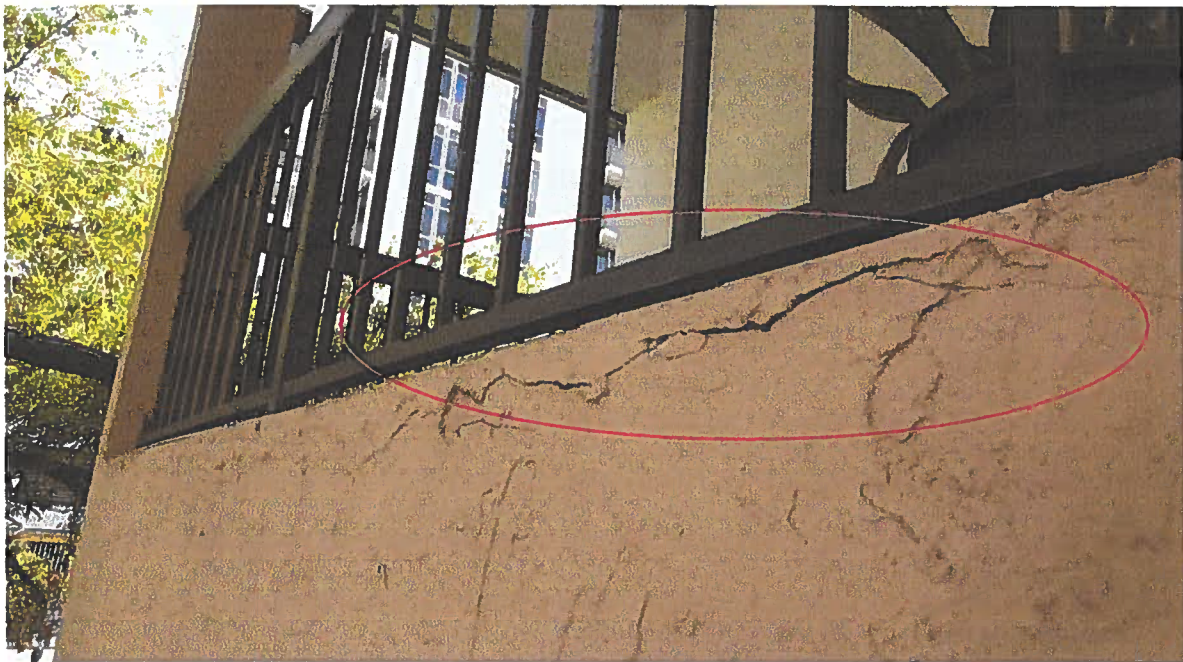
SPALLED CONCRETE IN BALCONY AT WEST SIDE MUST BE FIXED.
