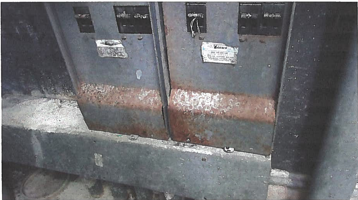
SIGNS OF CORROSION IN EQUIPMENT OF ELECTRICAL ROOM MUST BE REMOVED AND EQUIPMENT MUST BE SANDED AND PAINTED.
