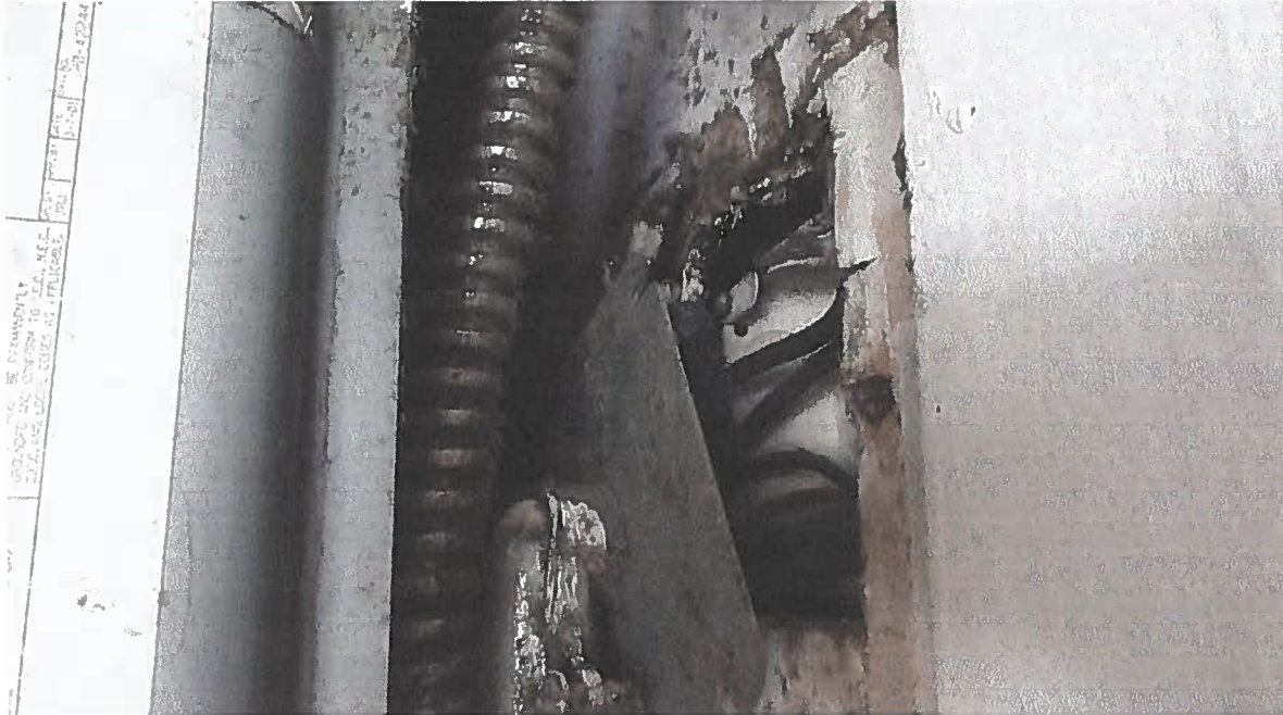
UNIT #4: EXPOSED WIRES IN AIR HANLDER CONNECTION.
