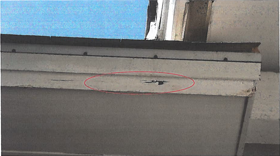
ROTTEN FASCIA MUST BE REPLACED.
