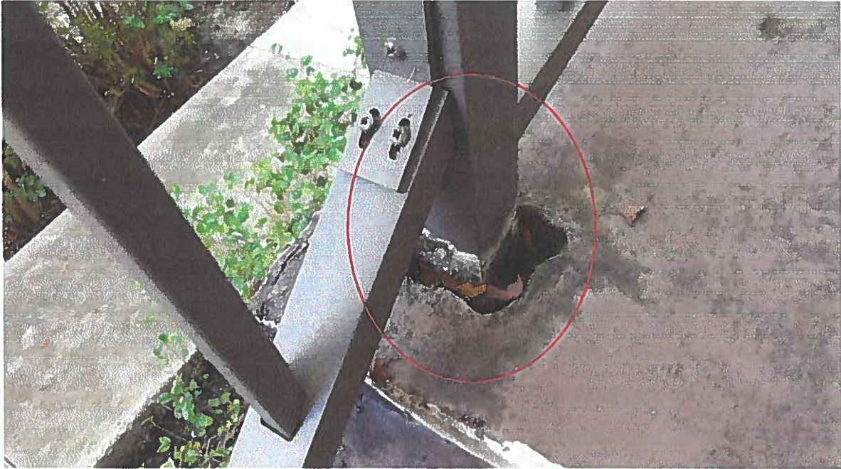
GAP AROUND RAILING POST POCKETS MUST BE RE-FILLED.
