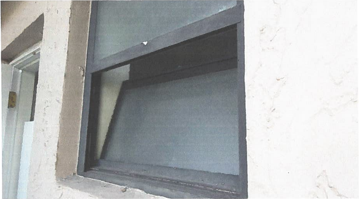
LOOSE WINDOW OF STORAGE MUST BE RE-INSTALLED.
