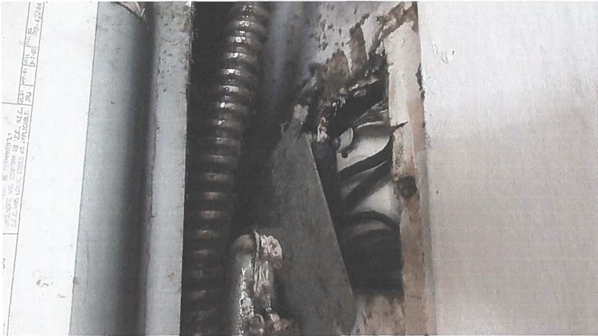
UNIT #4: EXPOSED WIRES IN AIR HANLDER CONNECTION.
