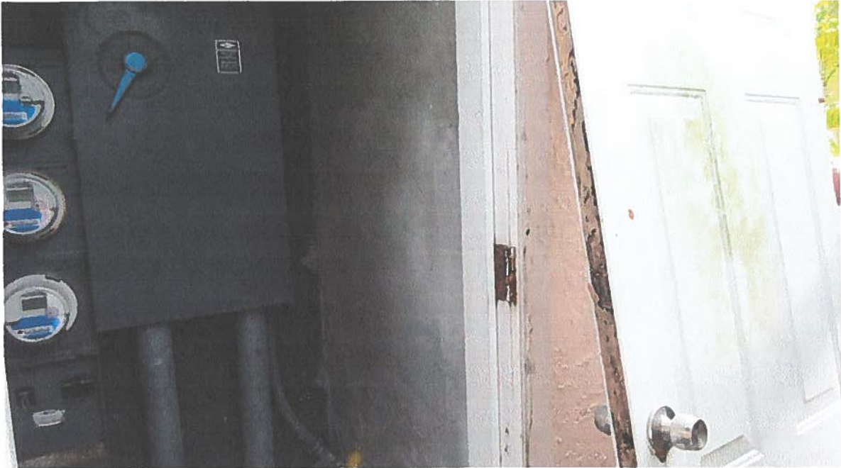
DAMAGED DOOR AND FRAME DOOR OF ELECTRICAL ROOM.
