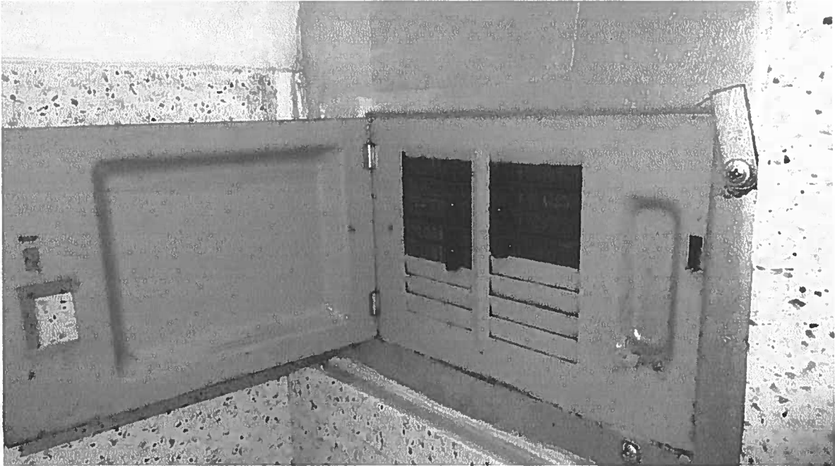
BREAKERS IN ALL PANELS MUST BE IDENTIFIED.
