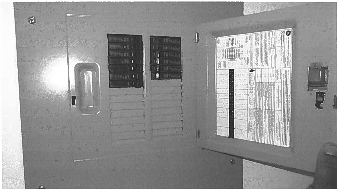
BREAKERS IN ALL PANELS MUST BE IDENTIFIED.
