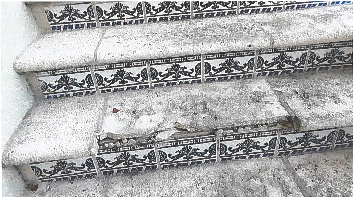
DAMAGED STEP OF STAIR (TRIP HAZARD) MUST BE REPAIRED.
