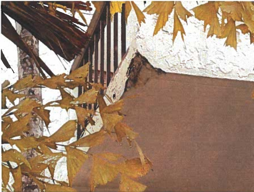
Edge "spalling" (exposed rebar) at the East balcony (South corner) of unit #6.
