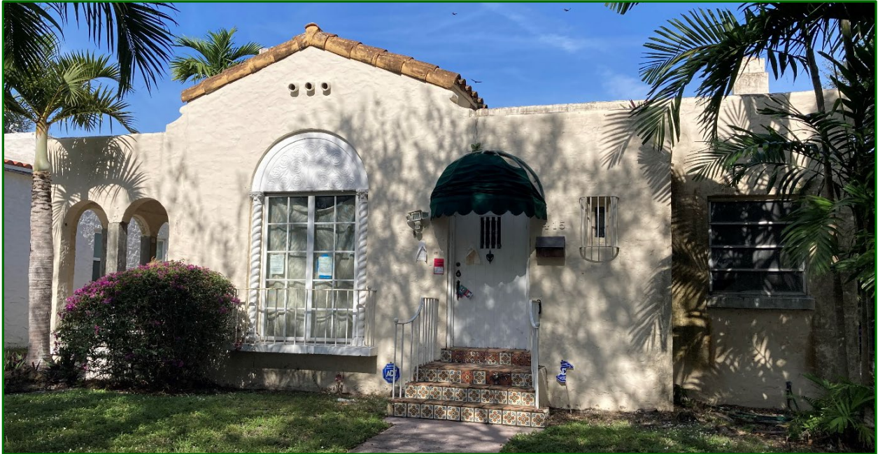
Figure 13: Front (South) Façade, 2023
