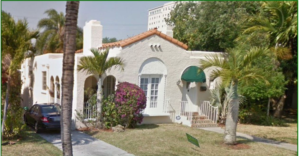
Figure 11: Front (South) & Side (West) Facades, 2011 Courtesy Google Streetview
