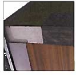
ANCHORED STEEL PLATE
