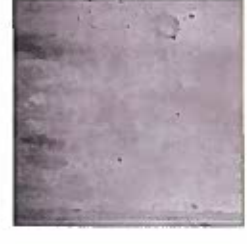
ROUGH STUCCO FINISH
