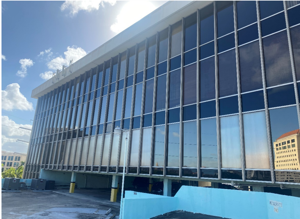
Typical glazing system around building perimeter
