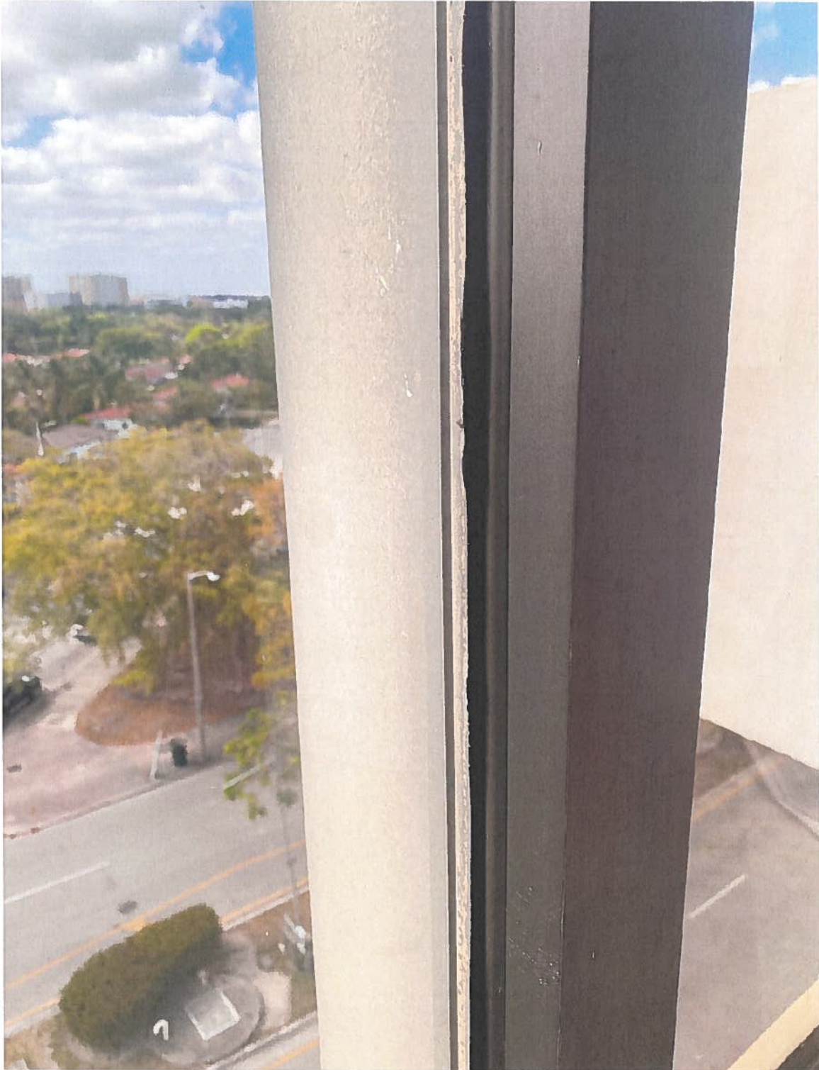
Typical interior seals at window system
