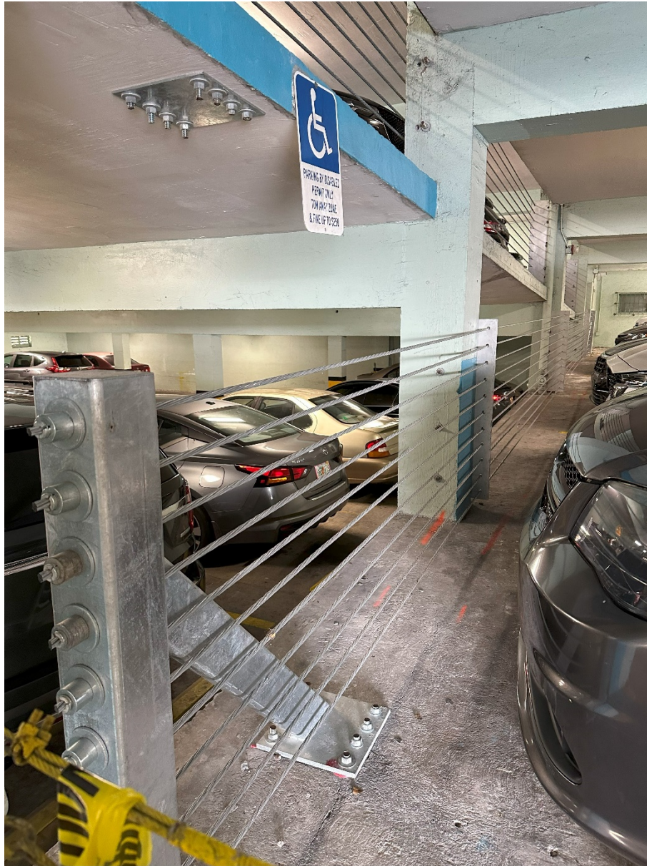
UPDATE 10-27-23: New cable railings final inspection
