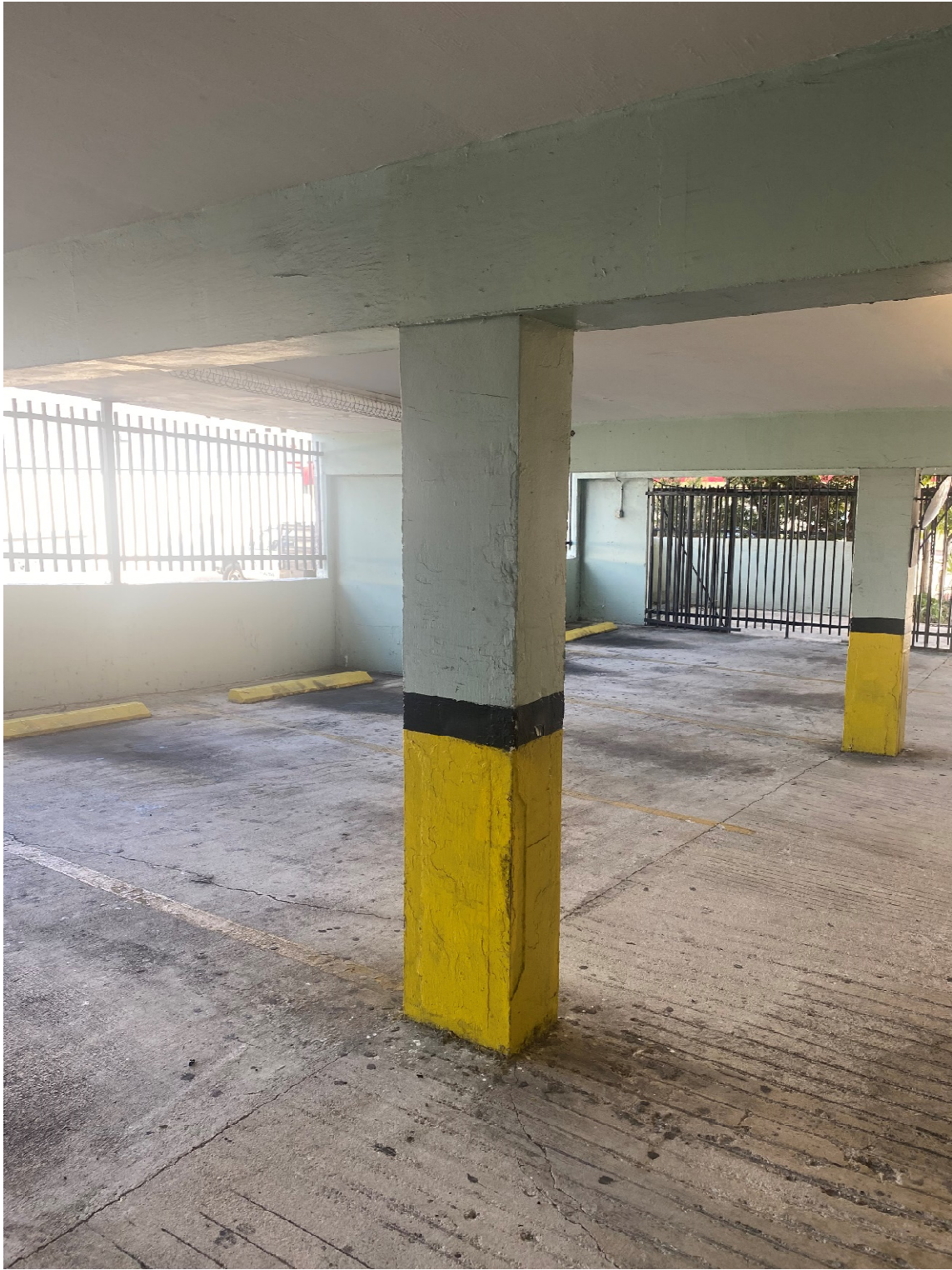
Parking Garage ground level typical column/beam
