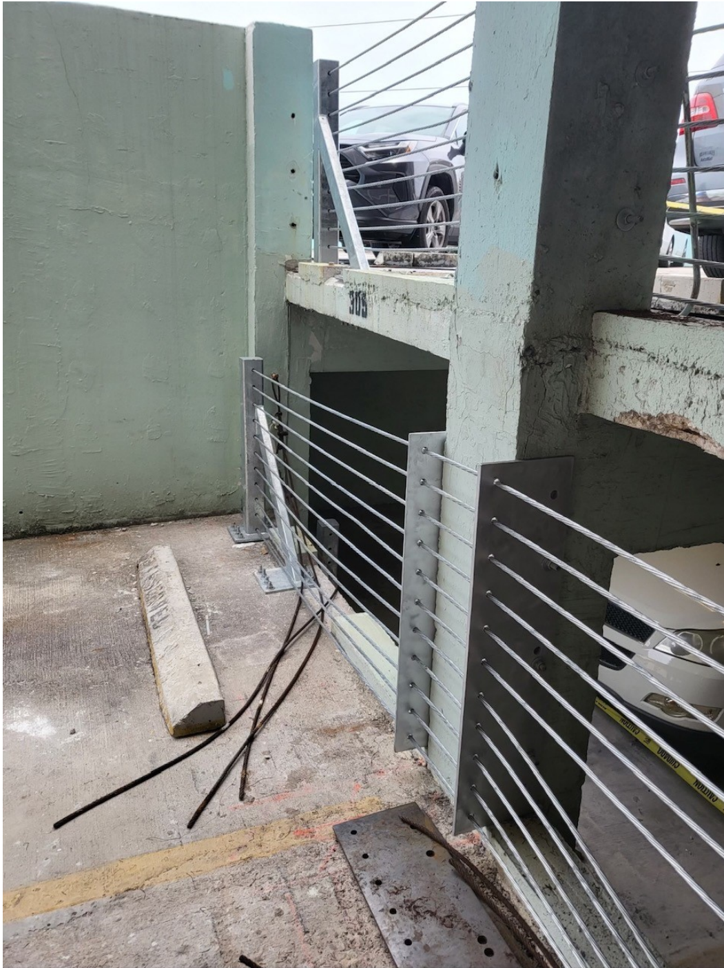
UPDATE 6-7-23: New cable railings installed
