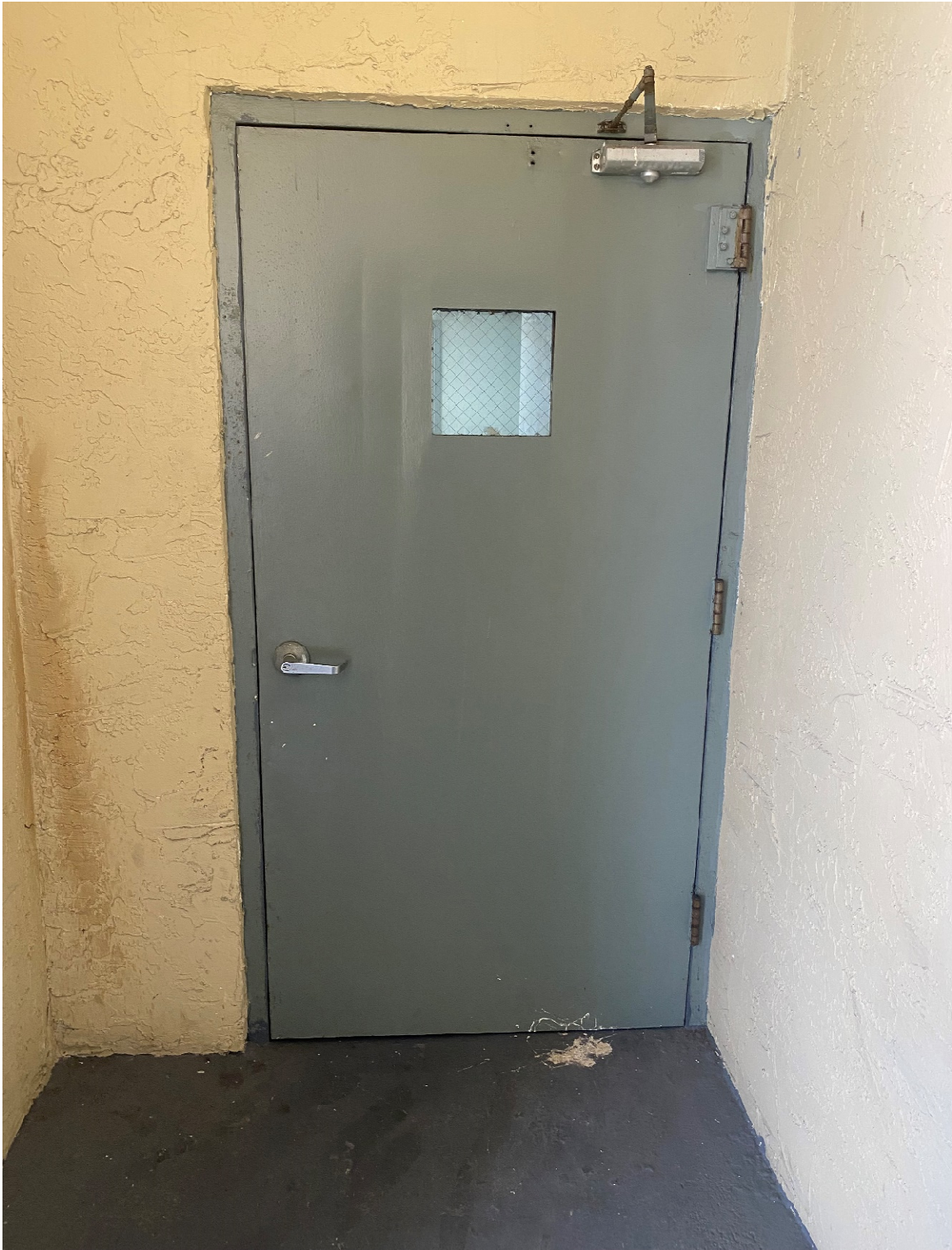
Typical exterior steel egress door at Main Building
