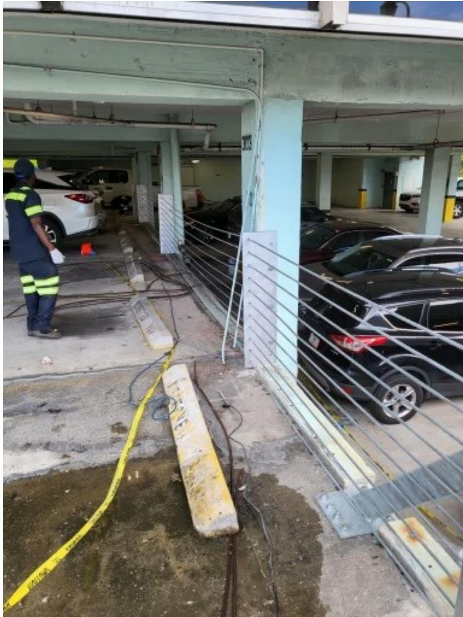
UPDATE 6-7-23: New cable railings installed
