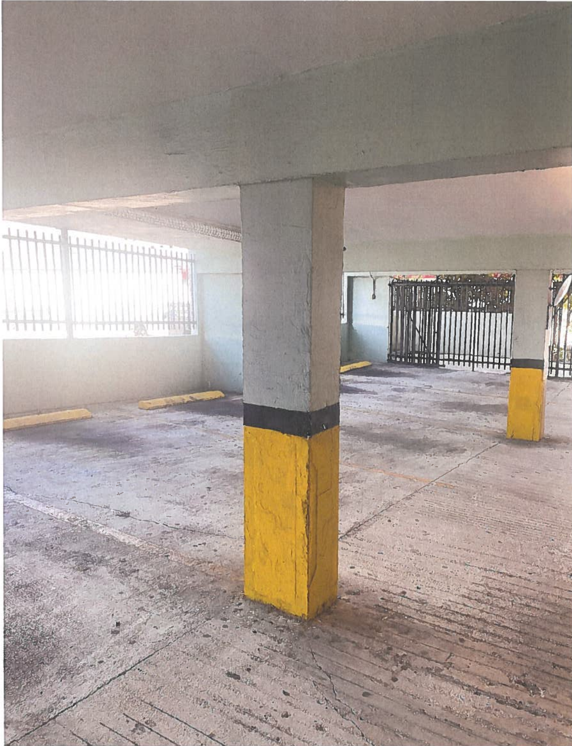
Parking Garage ground level typical column/beam
