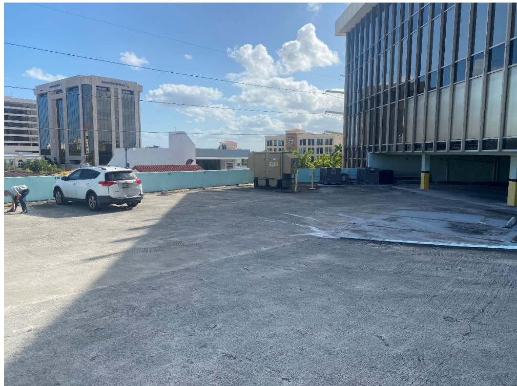
Top level of Parking Garage
