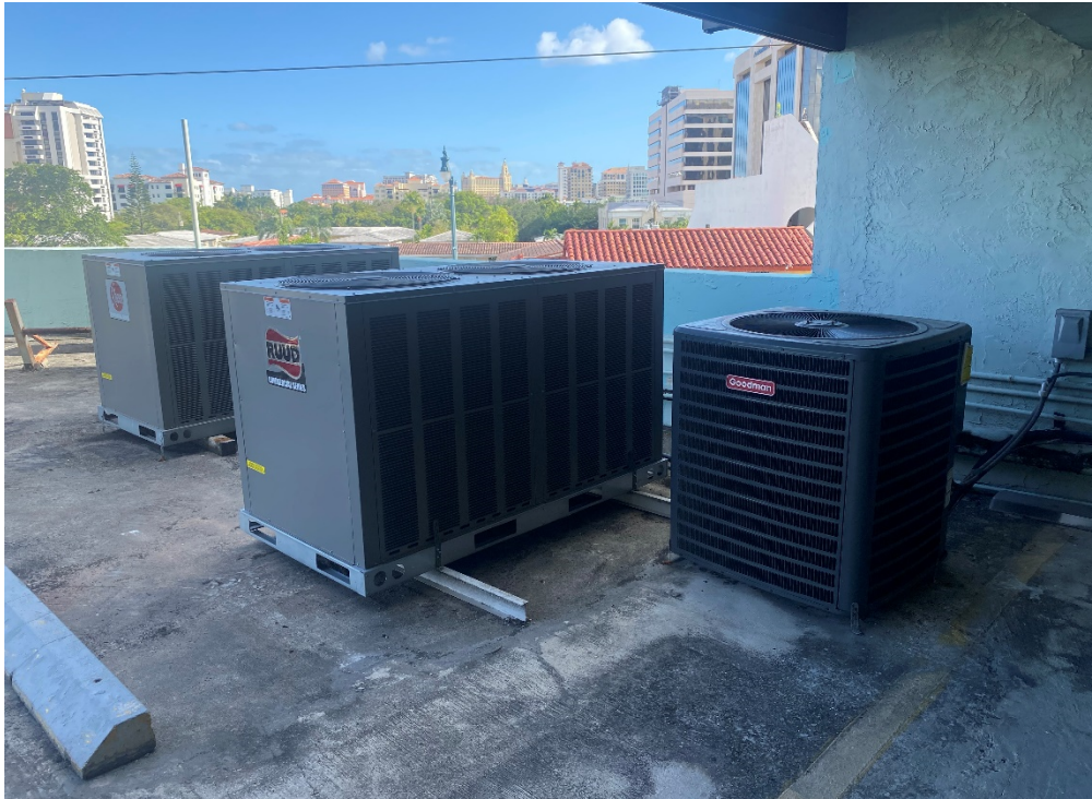
RTUs located at top of the Parking Garage
