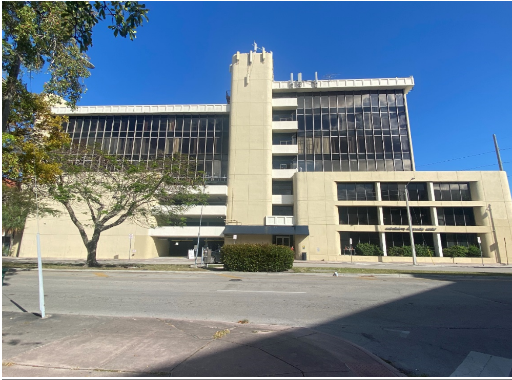
Front elevation along Ponce de Leon Blvd.
