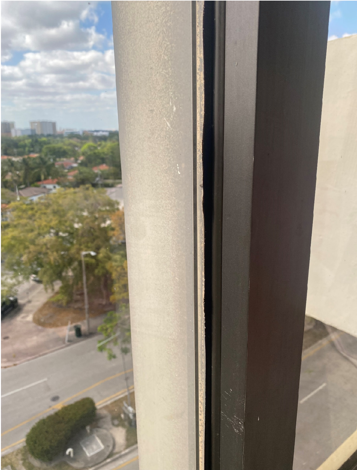
Typical interior seals at window system
