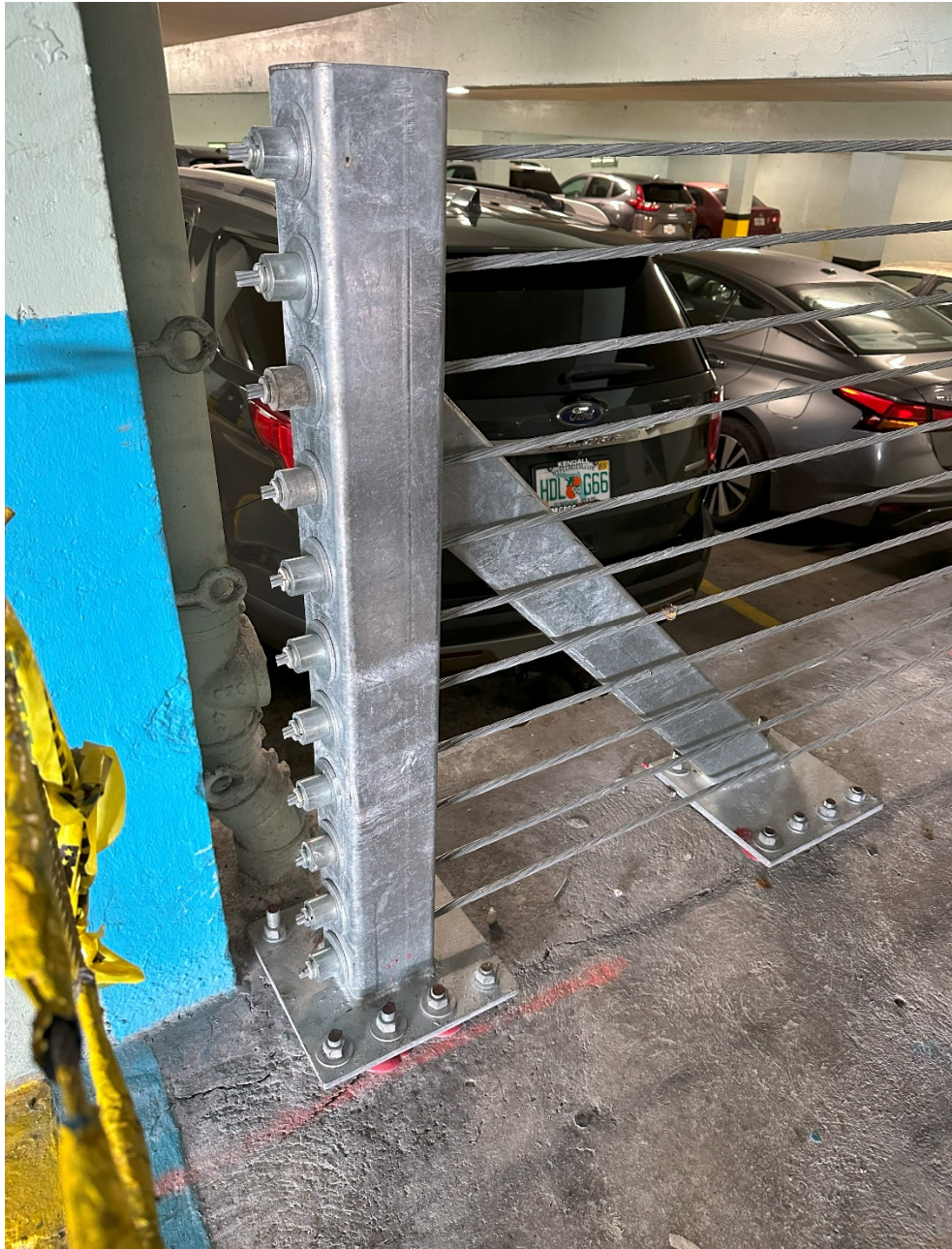
UPDATE 10-27-23: New cable railings final inspection
