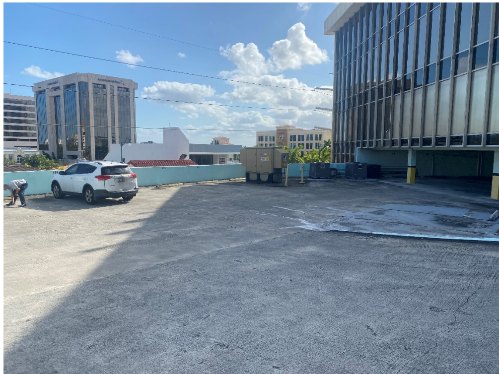
Top level of Parking Garage
