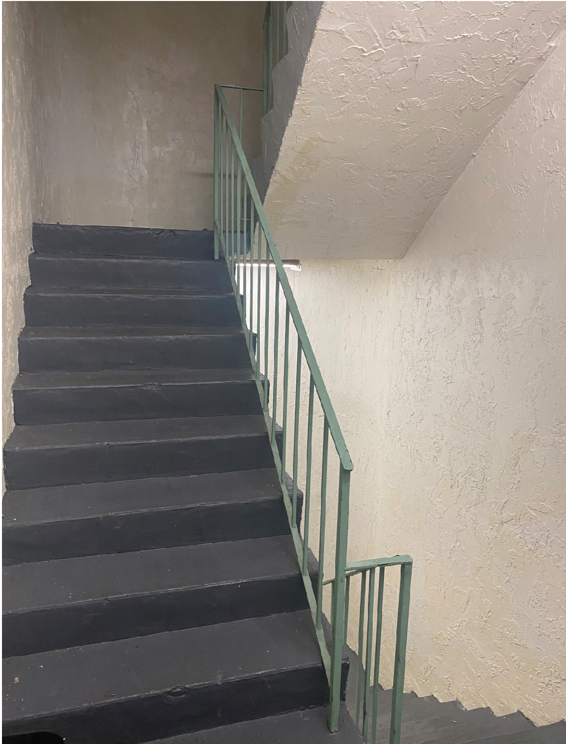
Typical framing at egress stairs
