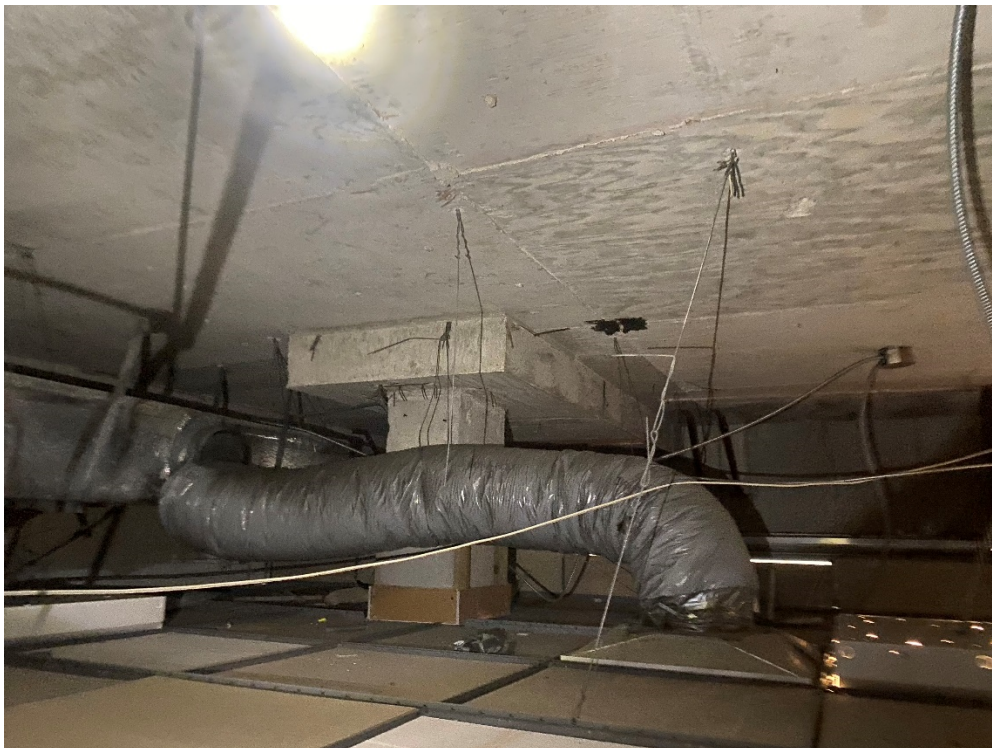
Typical concrete drop panel at interior column supports
