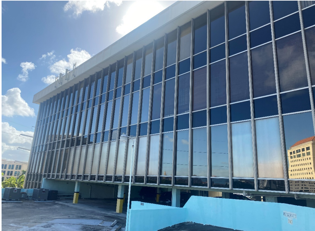
Typical glazing system around building perimeter
