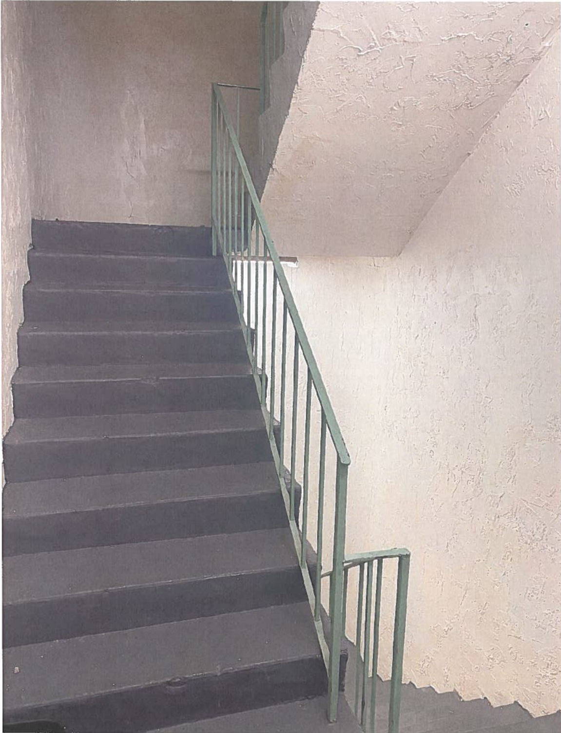
Typical framing at egress stairs
