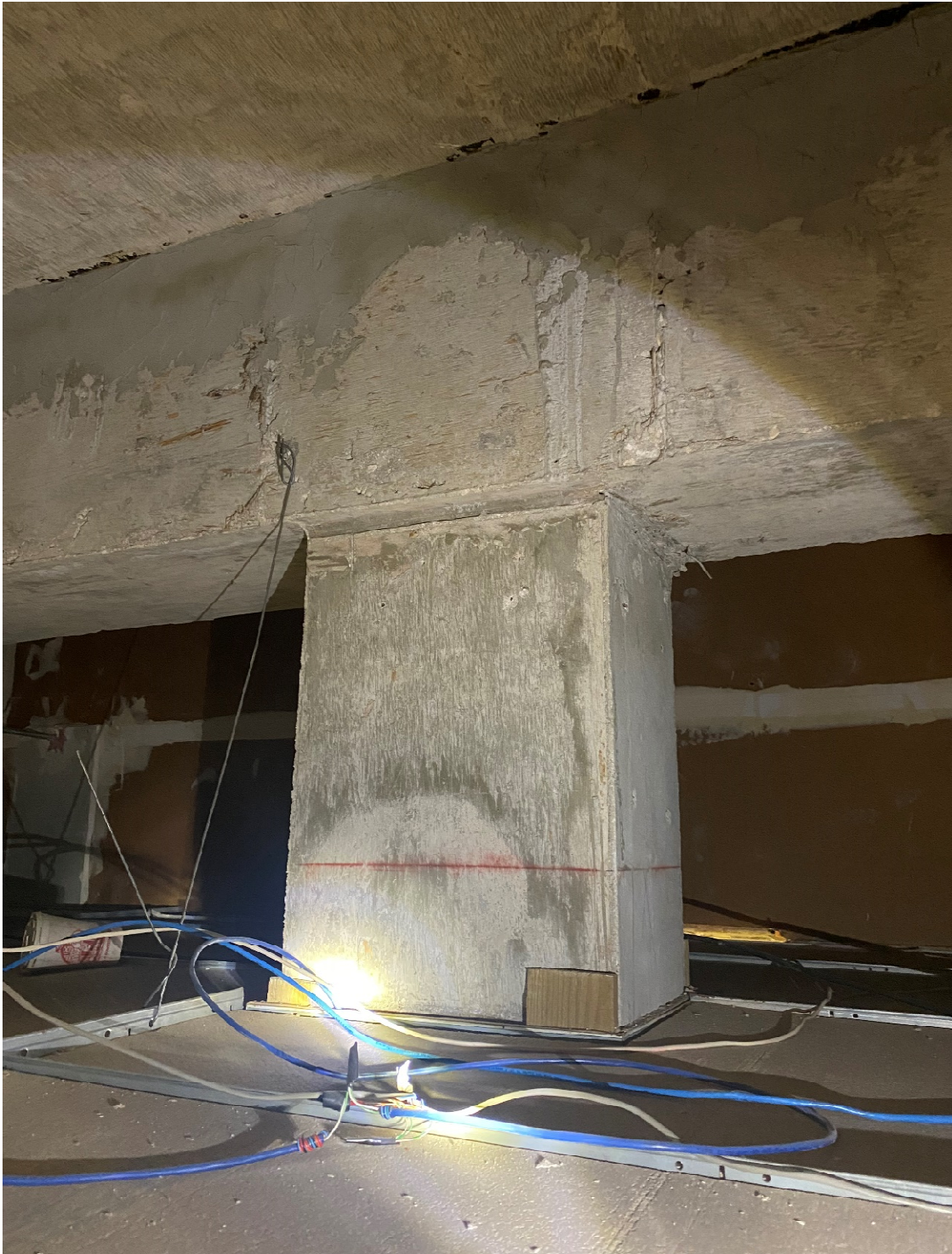
Typical interior concrete column/beam connection
