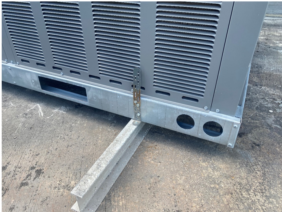
RTU attachment to aluminum frames
