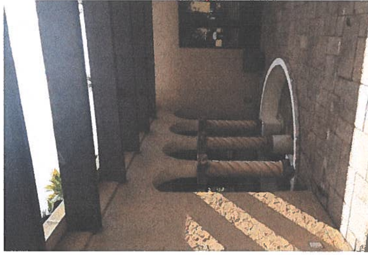
Existing Courtyard Fountain
