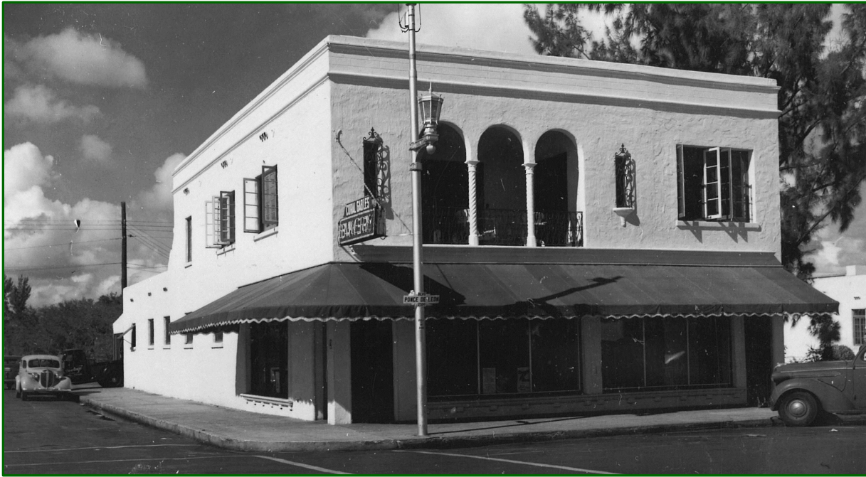
Figure 11: Peacock's Coral Gables Bakery Building with Paist Expansion, c.1940
