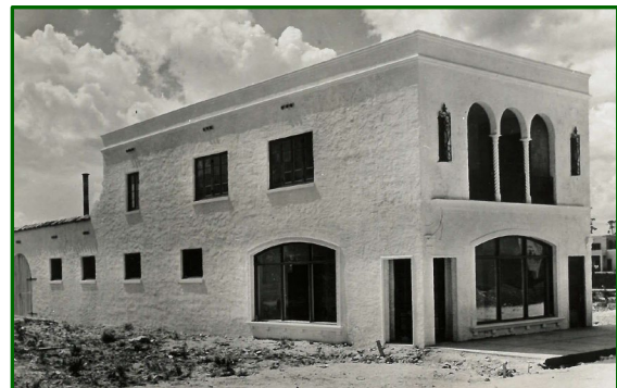
Figure 34: Side (South) Façade, 1925
