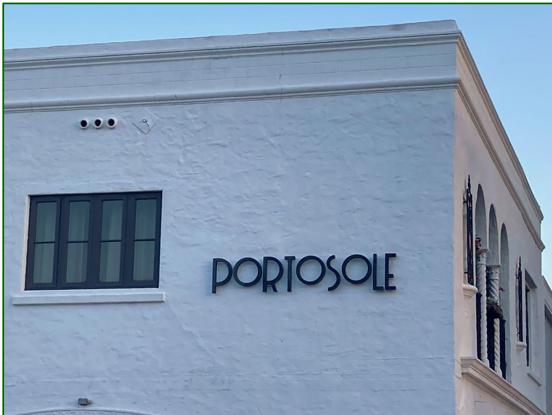
Figures 28: Ornamental Features, 2024 First Story: String Course, Bas Relief, Bracket and Door Frames [top] Cornice Feature: Moldings and Scored Stucco [bottom]
