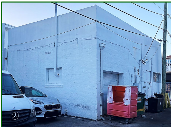
Figures 36: Raised Parapet Alteration at Rear Current Photos, 2024 South Façade [top] Northwest Corner [bottom right] Note: smooth stucco of infill and parapet additions Alteration Drawings Permit #24498, 1977 [bottom left]
