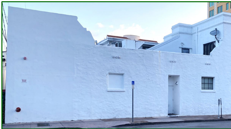
Figures 36: Raised Parapet Alteration at Rear Current Photos, 2024 South Façade [top] Northwest Corner [bottom right] Note: smooth stucco of infill and parapet additions Alteration Drawings Permit #24498, 1977 [bottom left]
