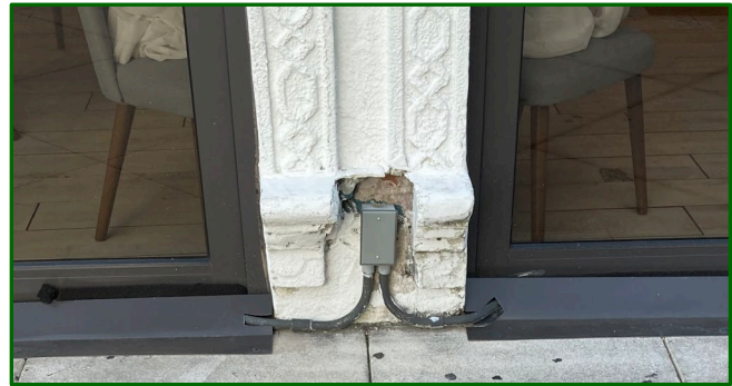
Figure 32: Unpermitted Exterior Electrical Installation on Historic Fabric, 2024
