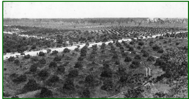
Figure 1: Streets in Coral Gables under Construction, July 22, 1922
