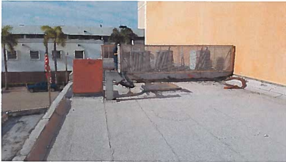
Another view of the rusty steel beam, both beams needs to be replace
