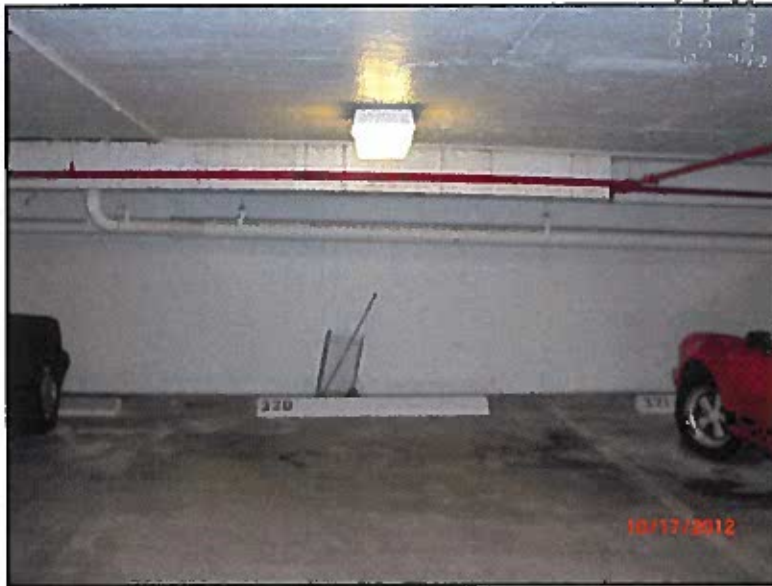
PHOTO # 21: trench drain drop ceiling between Parking Spaces 314 & 327
