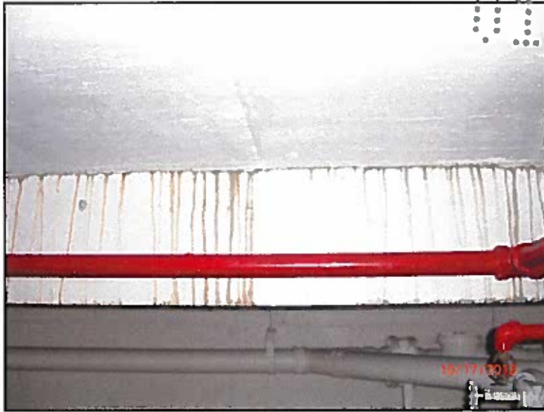
PHOTO # 25: trench drain drop ceiling between Parking Spaces 52 & 61
