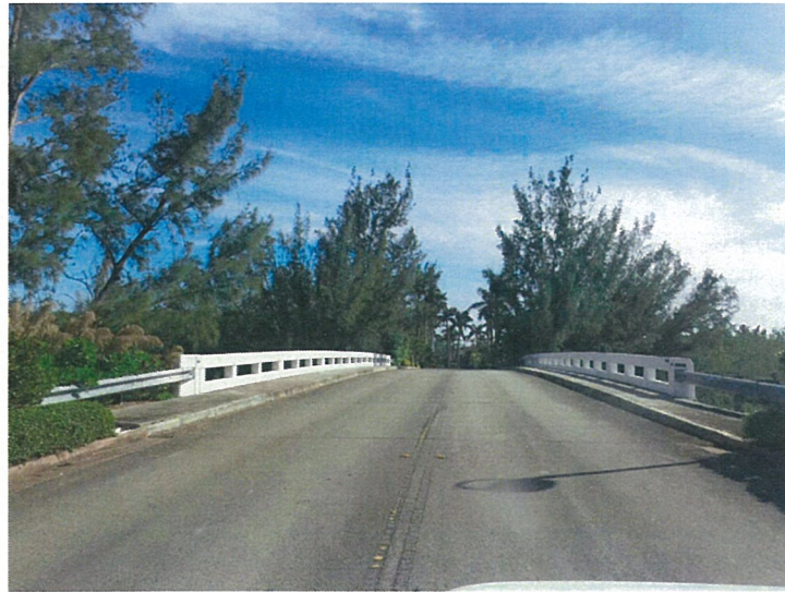
ISLA DORADA BRIDGE EXISTING CONDITIONS NTS
