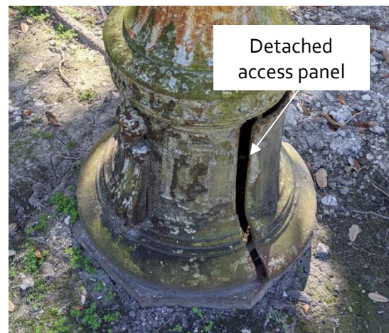
Figure 10. Detached access panel (photo by EverGreene, January 2020).
