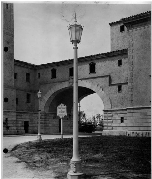
Figure 1. Fully intact original “White Way” lamppost (GE publicity department, July 1927).
