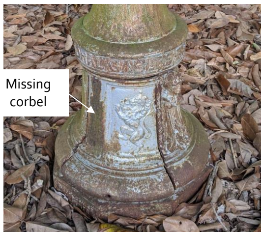
Figure 9. Missing figurative corbel (photo by EverGreene, January 2020).
