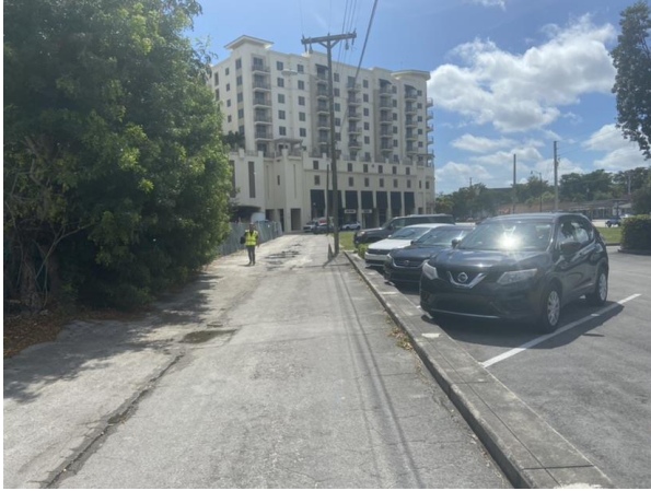
Looking south along east alleyway. Subject property is to the right.
