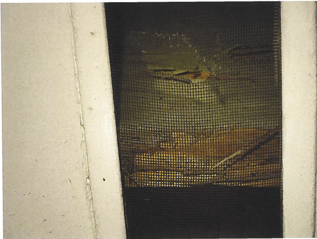
Photograph 15 – Termite damage at the east roof overhang wood framing.
