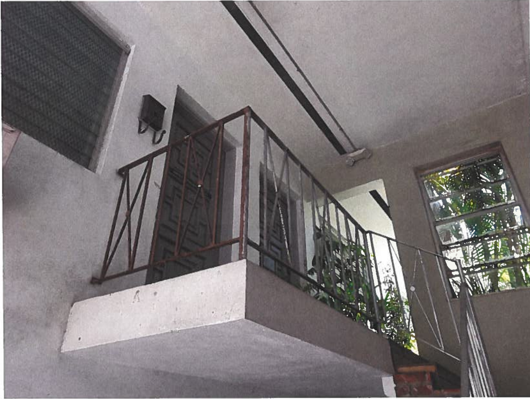
Photograph 6 – Steel guardrails with surface corrosion at south end of second-floor corridor.
