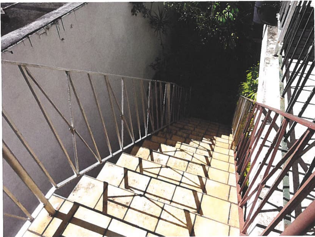
Photograph 19 – Wrought iron guardrails at staircase.
