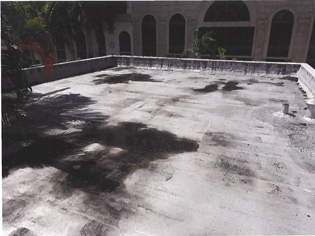
Photograph 12 – Ponding water spots at the south end of the roof.
