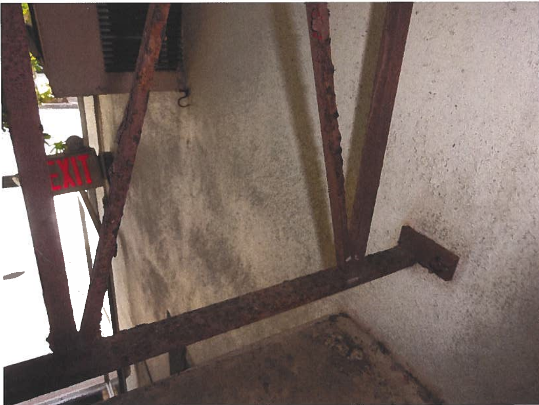
Photograph 7 – Surface corrosion shall be sanded and repainted with anti-corrosive metal paint.
