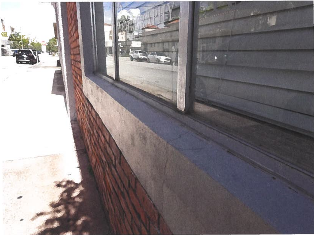
Photograph 23 – Cracked sealant caulking at exterior storefront.
