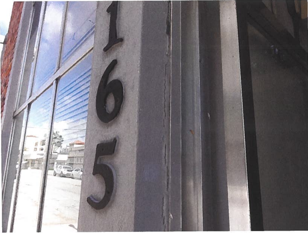
Photograph 24 – Cracked sealant caulking at exterior storefront.
