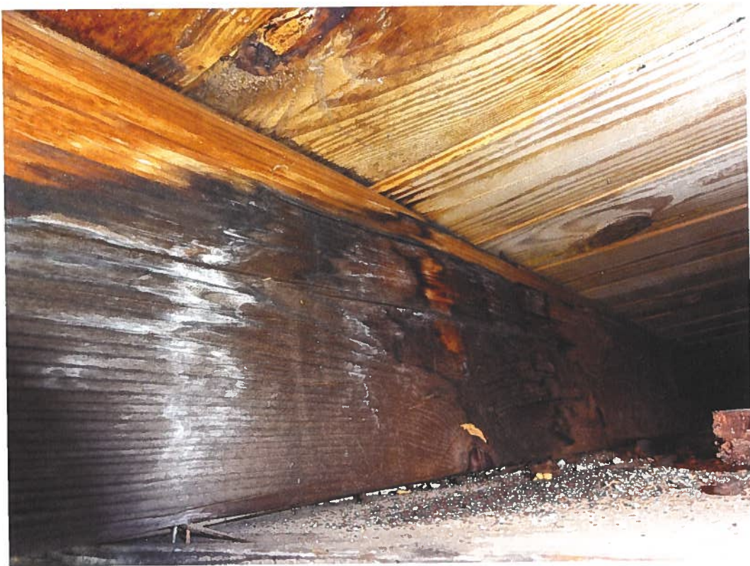
Photograph 29 – Water and termite damage on wood joists at second-floor overhang soffit.
