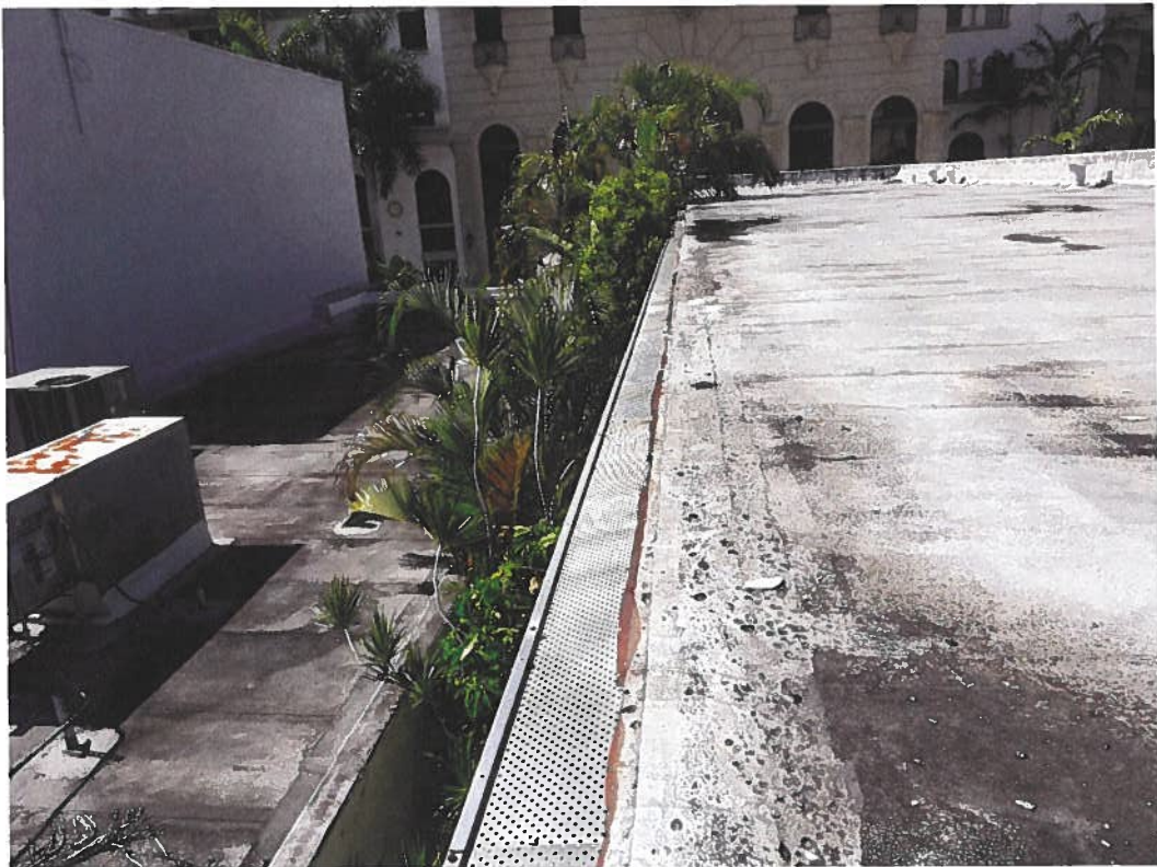
Photograph 13 – The membranes along the east end of the roof need to be restored.
