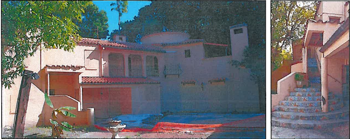
Figures 19 and 20: Rear (West) Façade, 2017 [left] and Stair Detail, 2016 [right]
