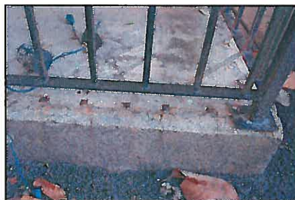
Figure 12: Wrought Iron Railing Detail, 2017
