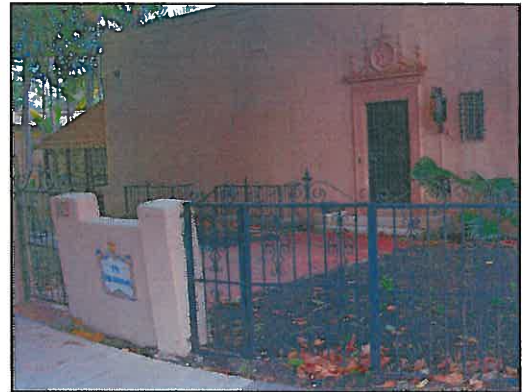
Figure 7: Front (South) Façade, 2017
