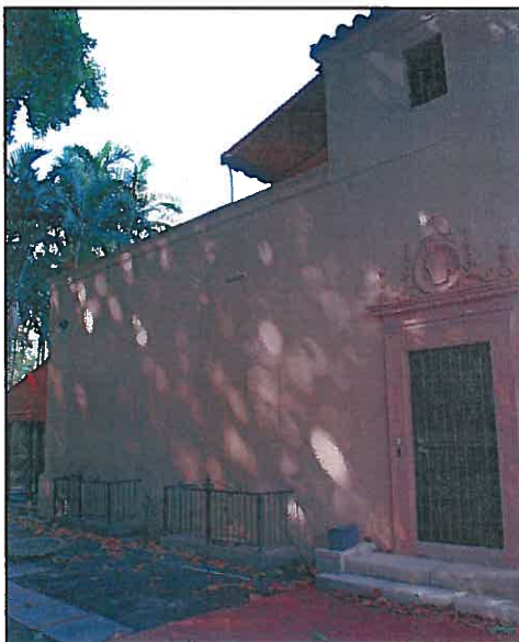
Figure 11: Front (South) Façade, 2017
