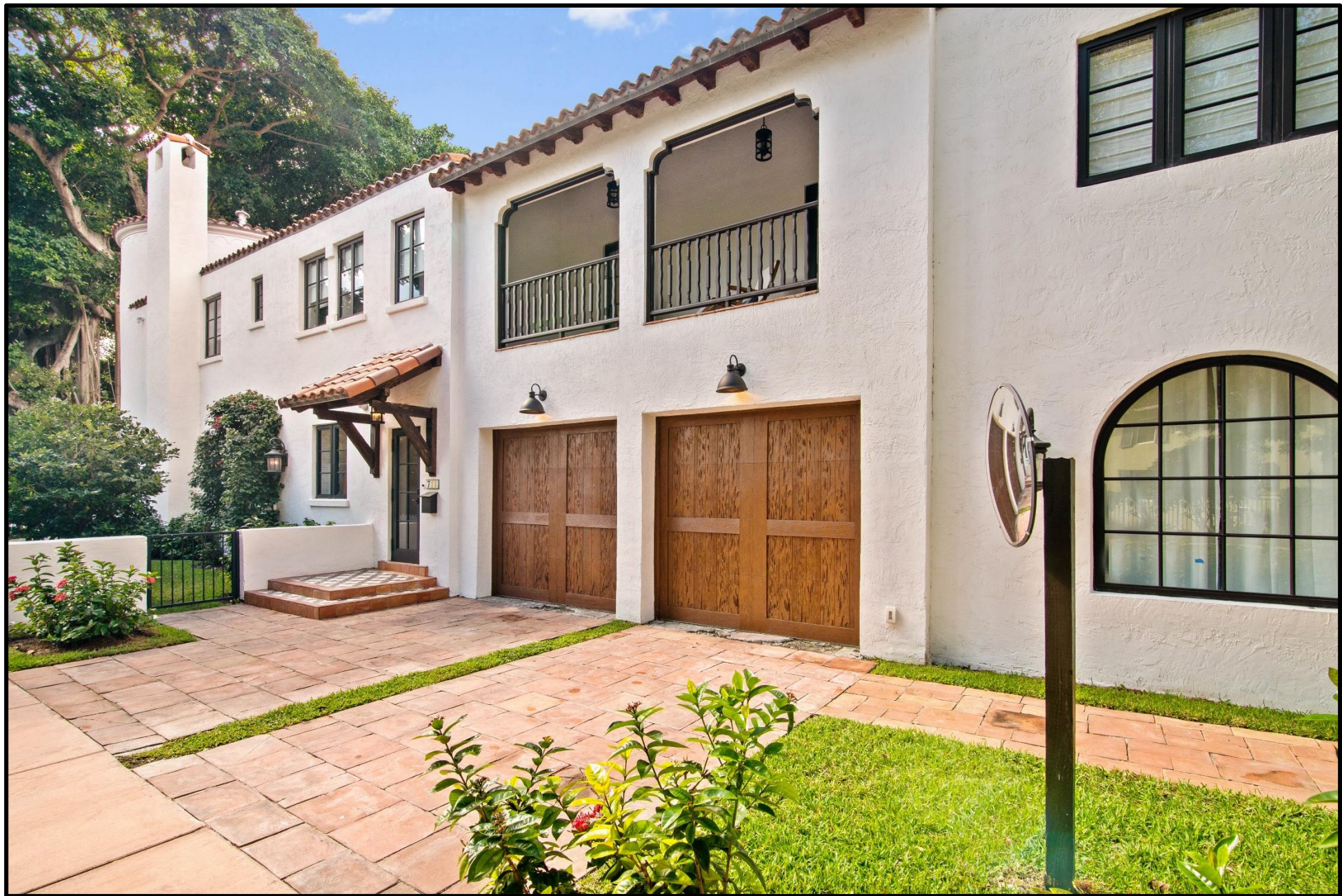
East Façade – After
