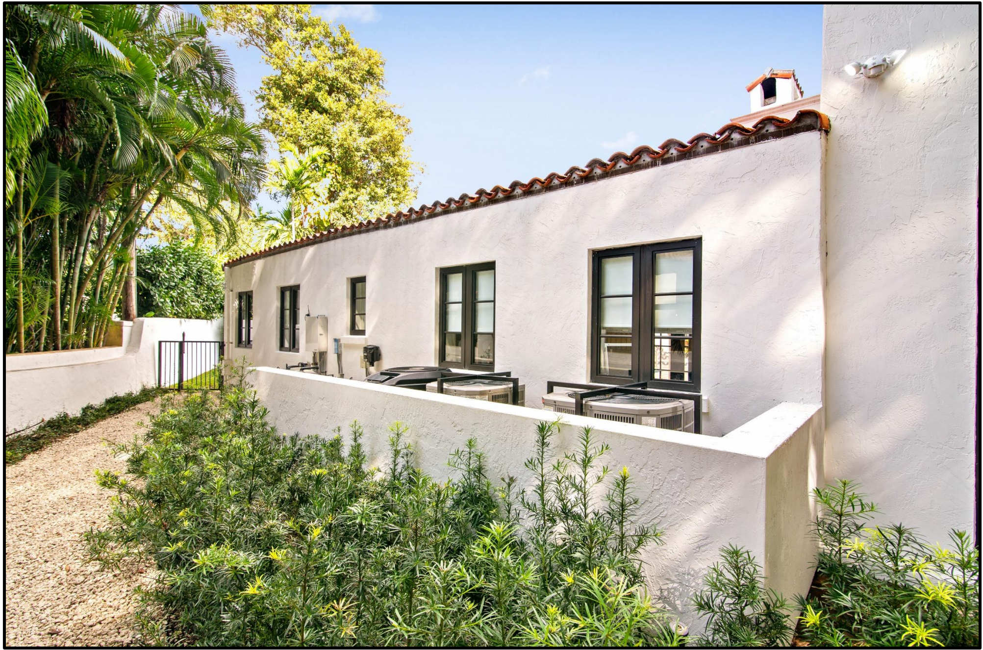
West Façade – After
