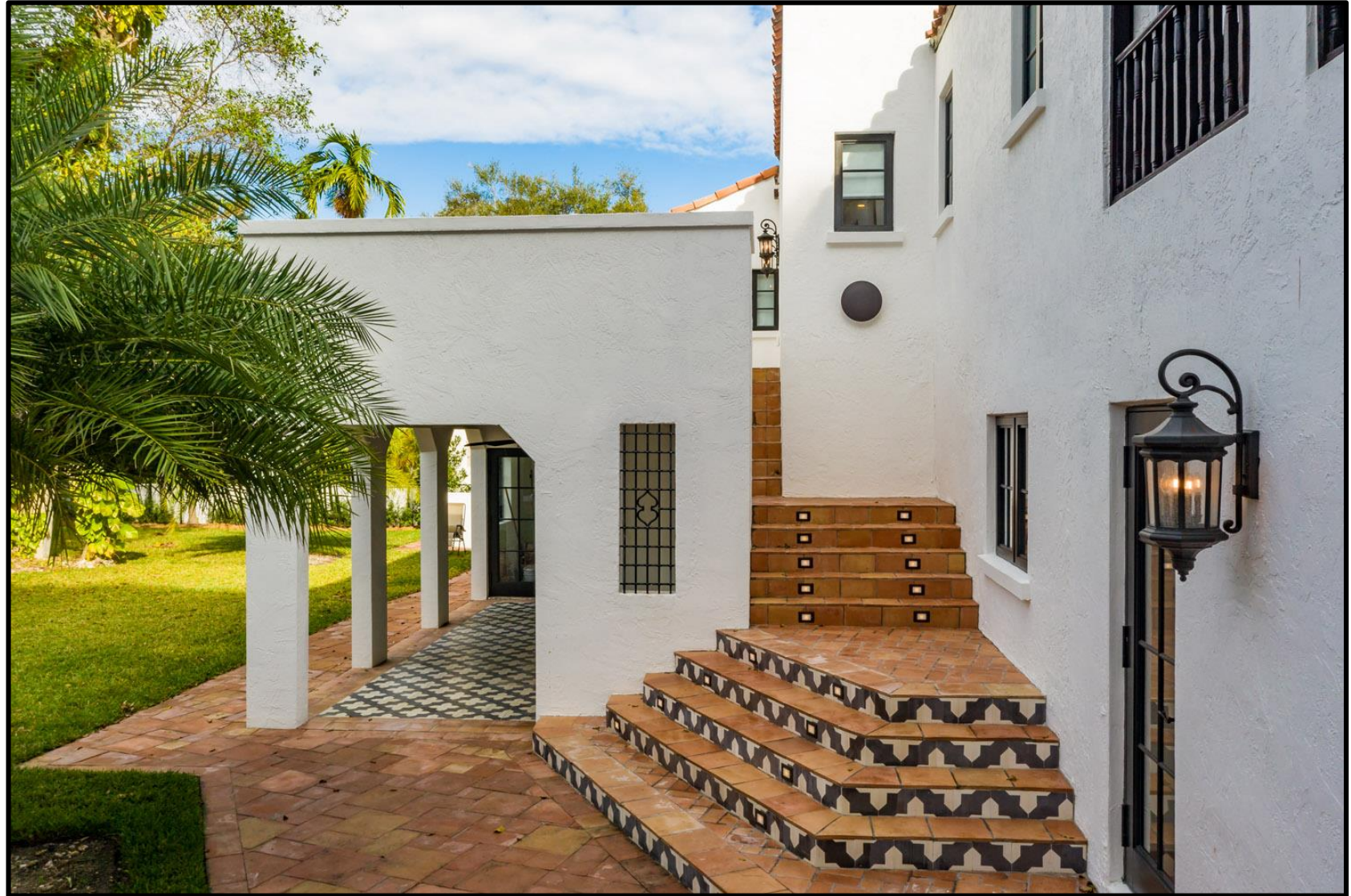
West Façade (looking north) – Before & After
