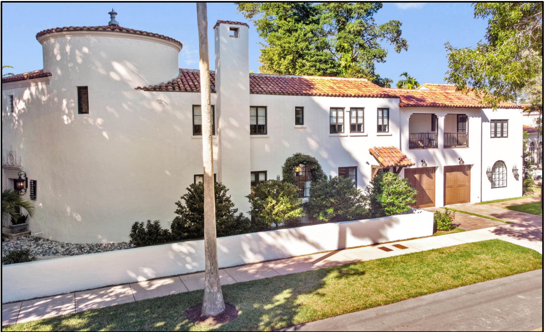
East Façade – After
