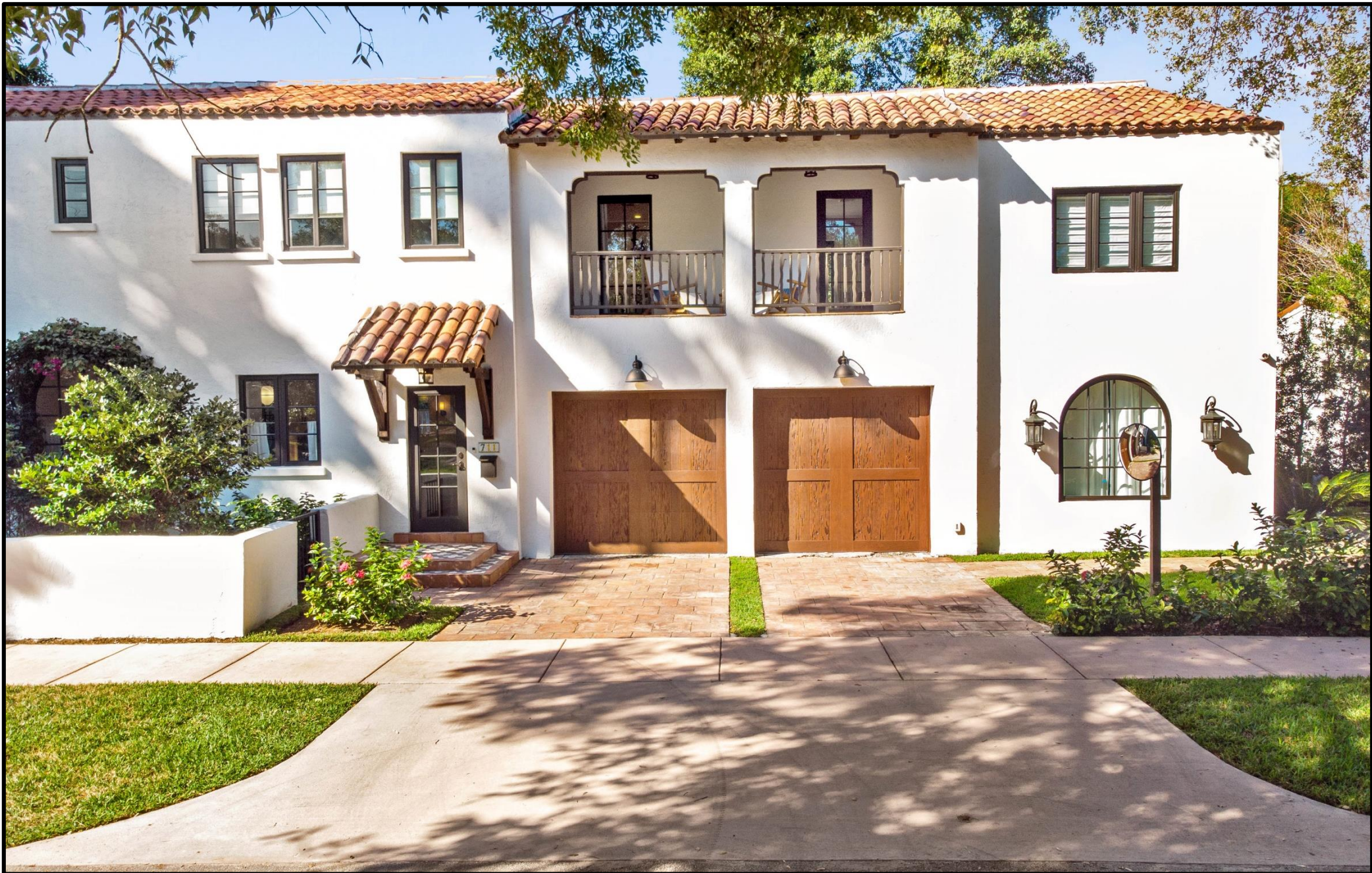
East Façade – After
