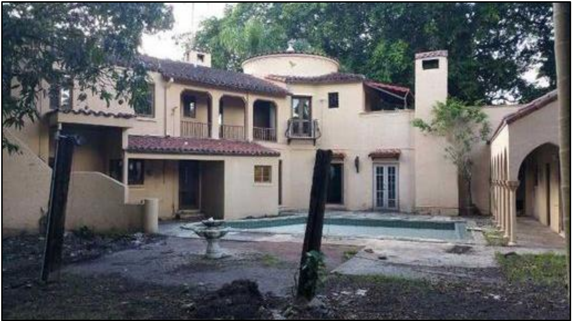
West and North (Rear) Facades – Before
