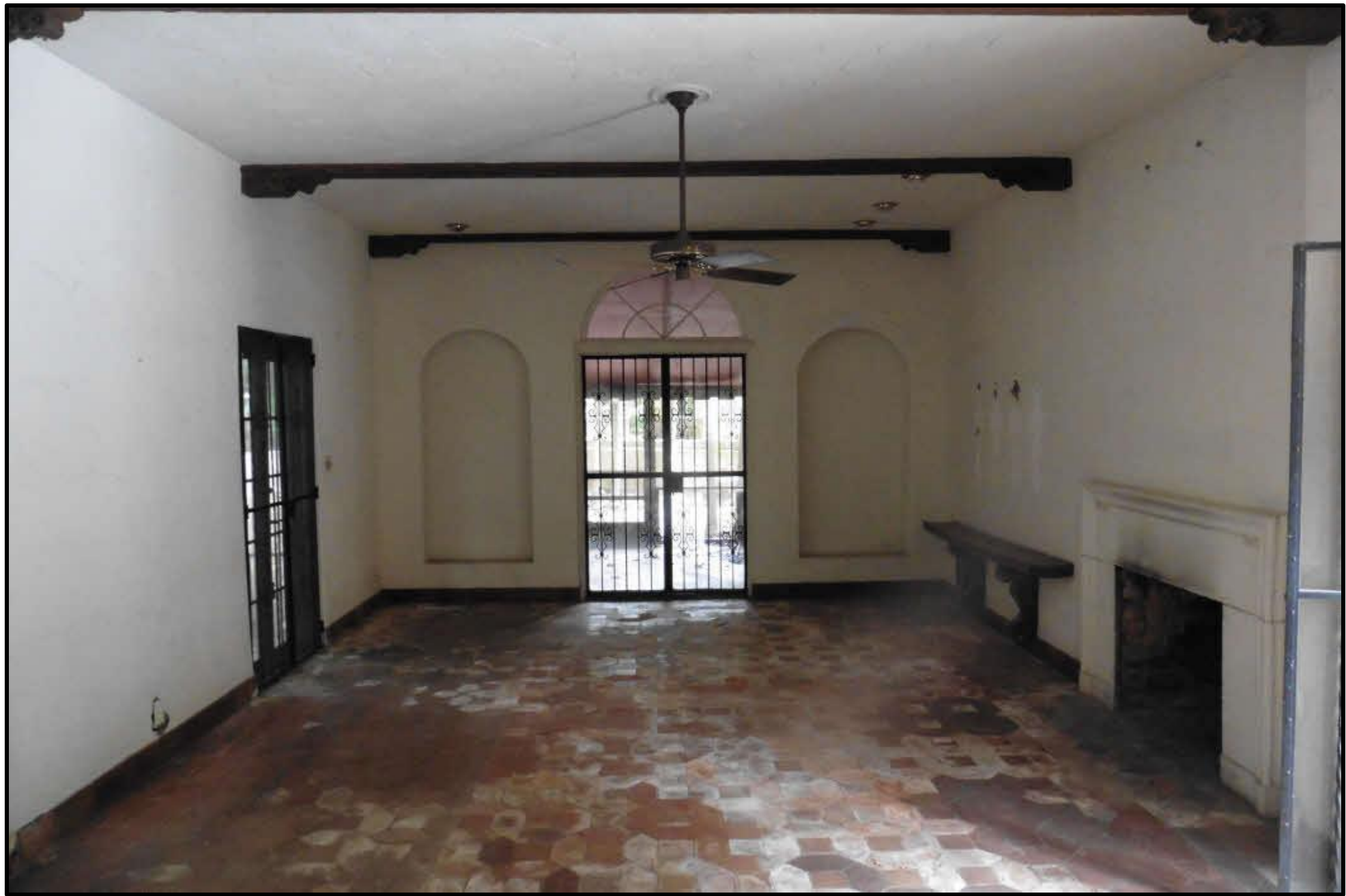
Interior – Living Room Before
