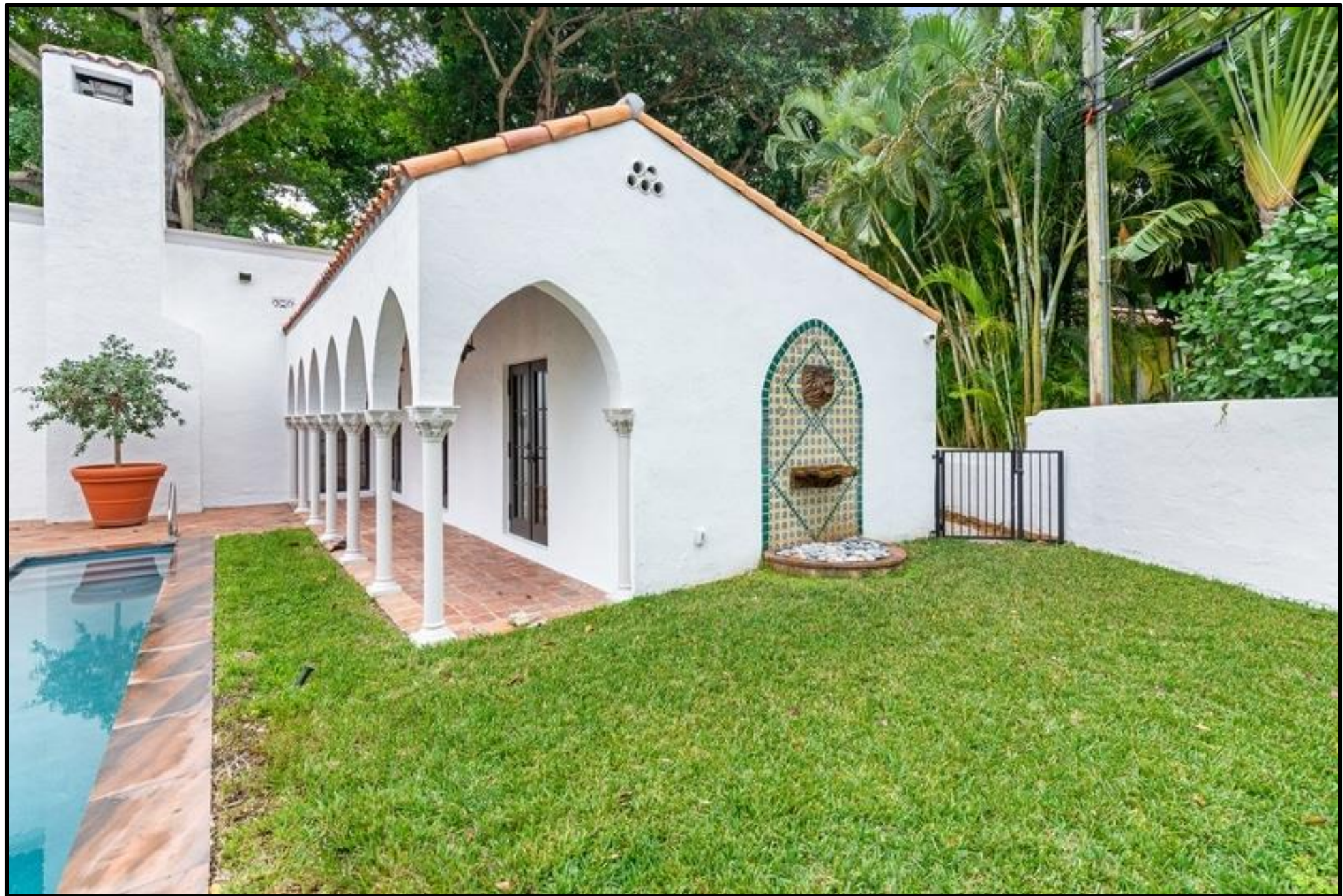
North (Rear) Façade – After
