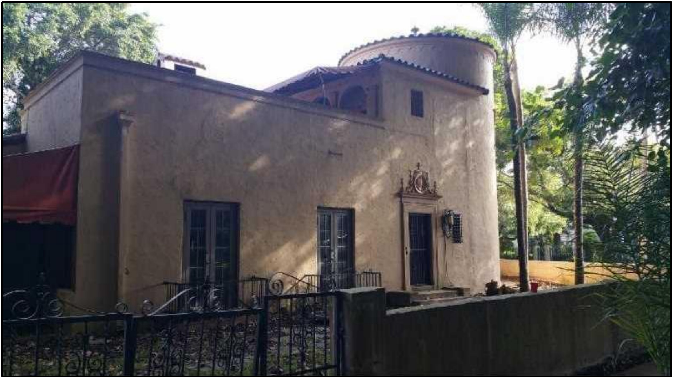
South (Front) Façade - Before
