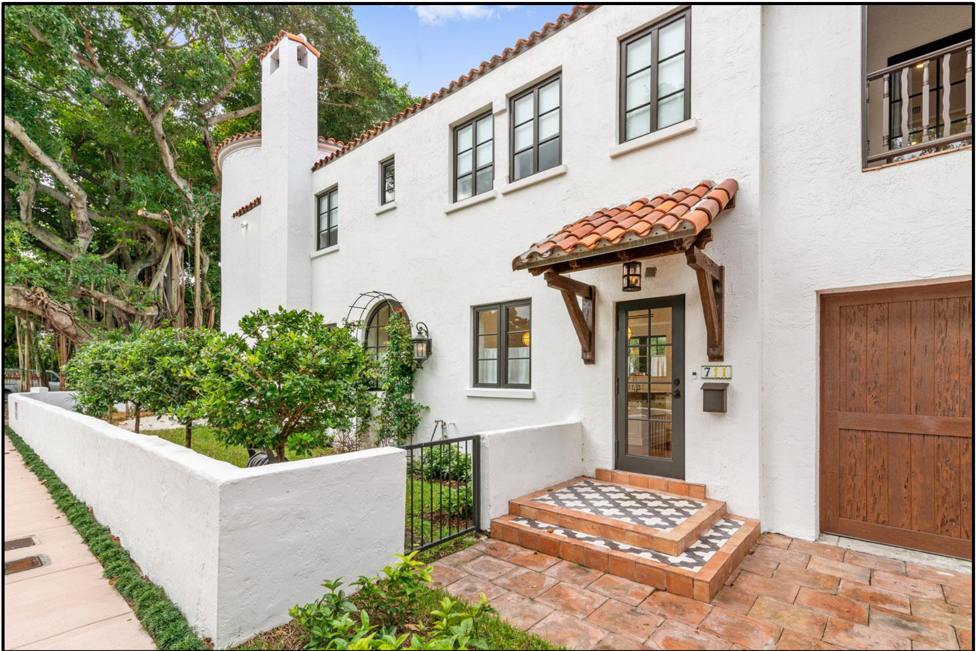
East Façade – After
