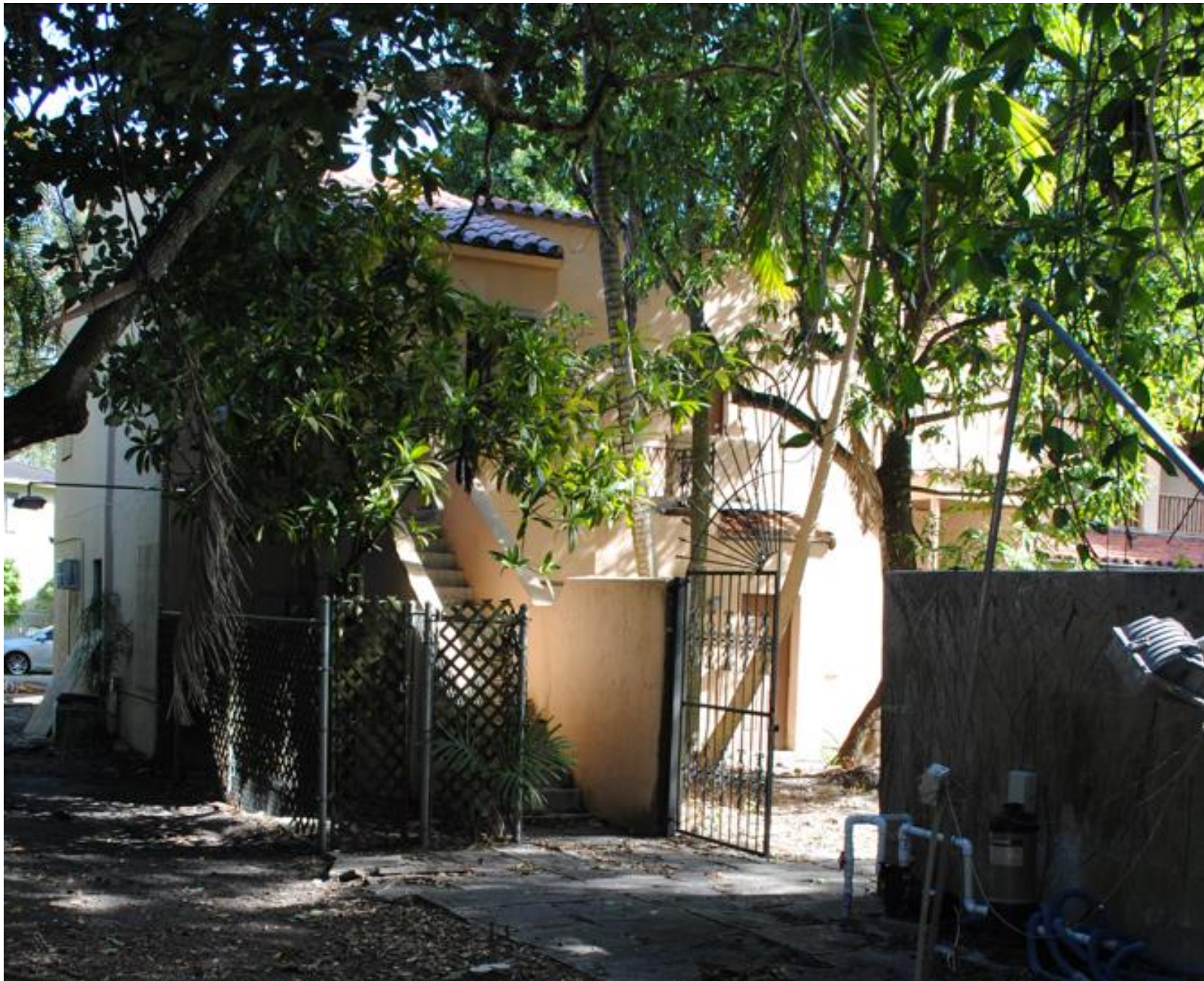
Northwest Corner – Before
