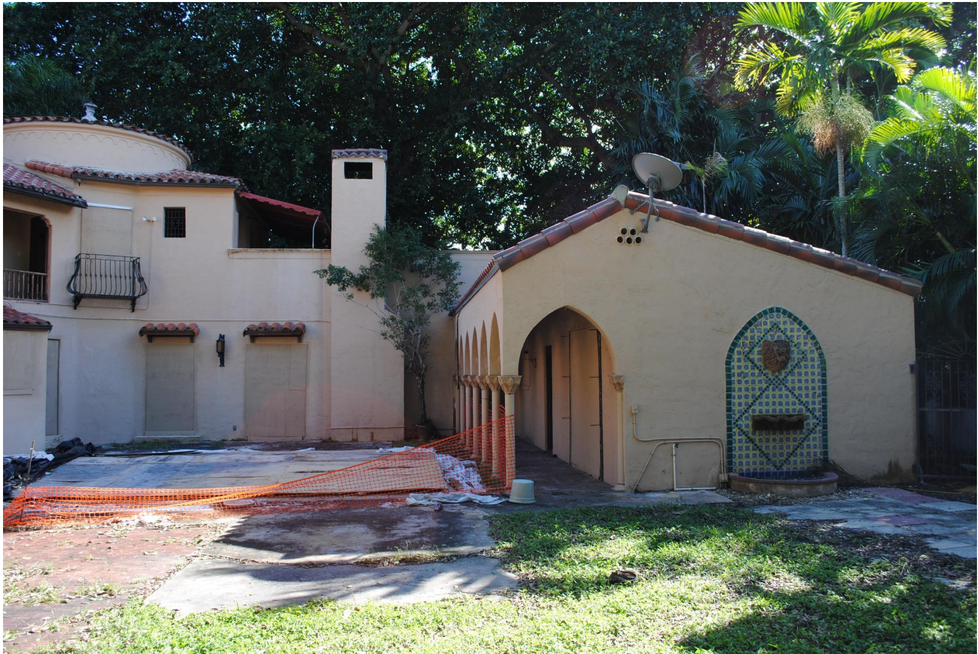
North (Rear) Façade – Before
