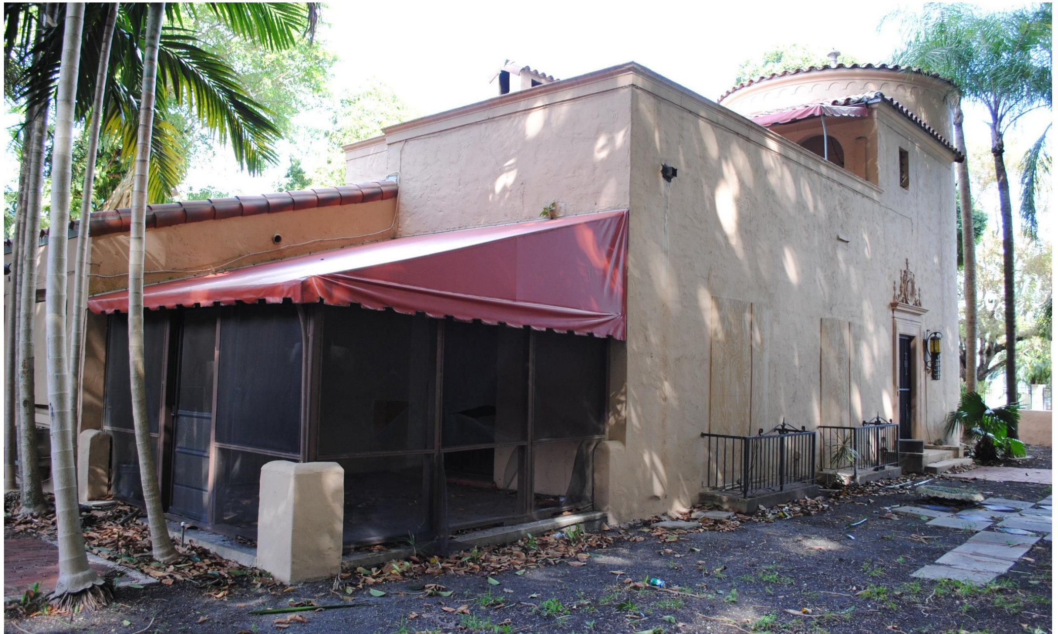
South (Front) Façade - Before
