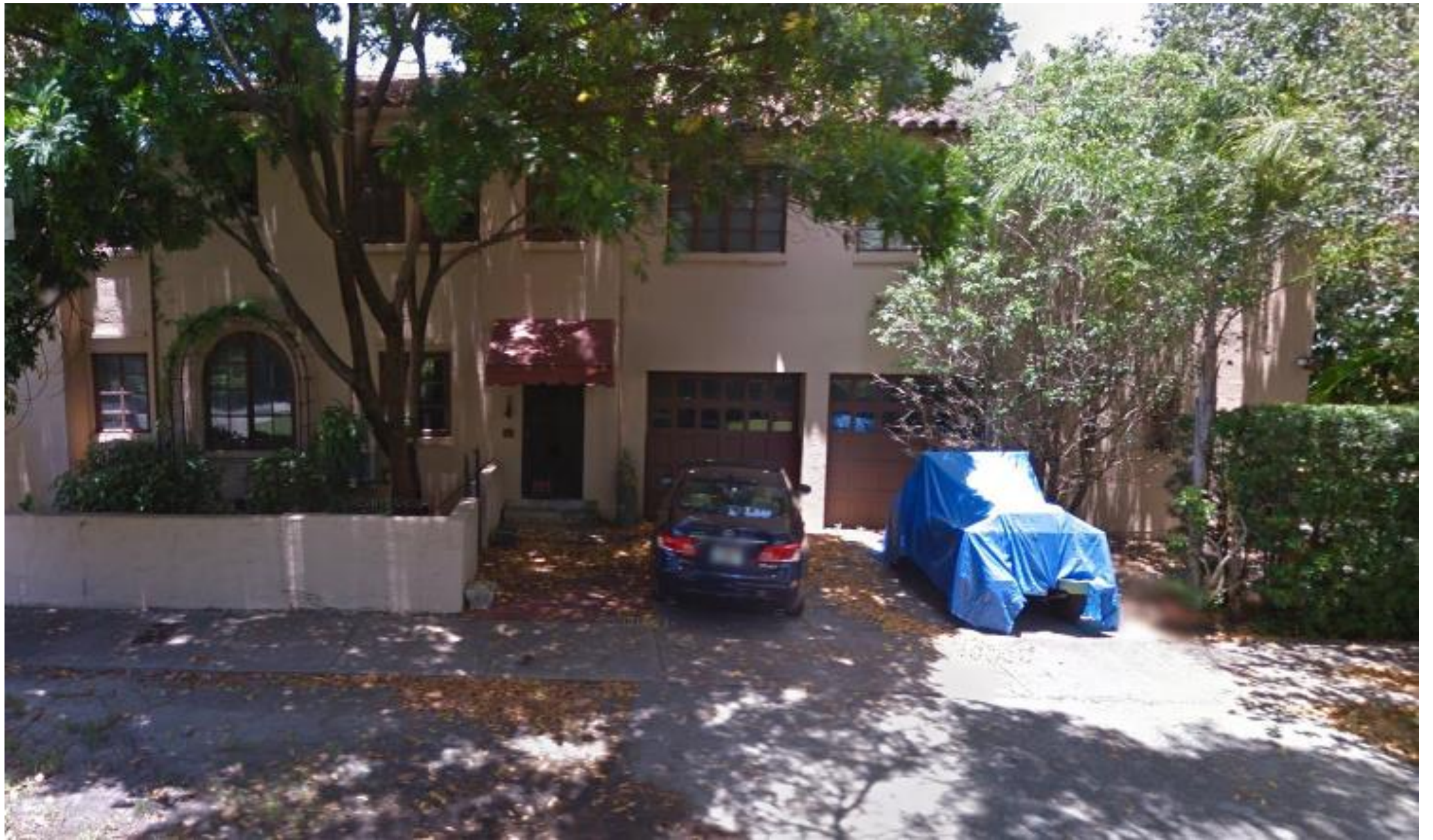
East Façade – Before
