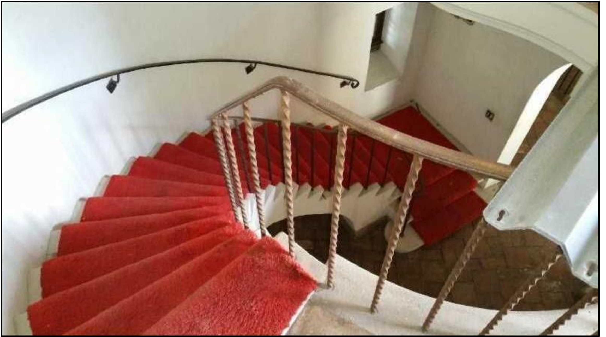
Interior –Staircase Before
