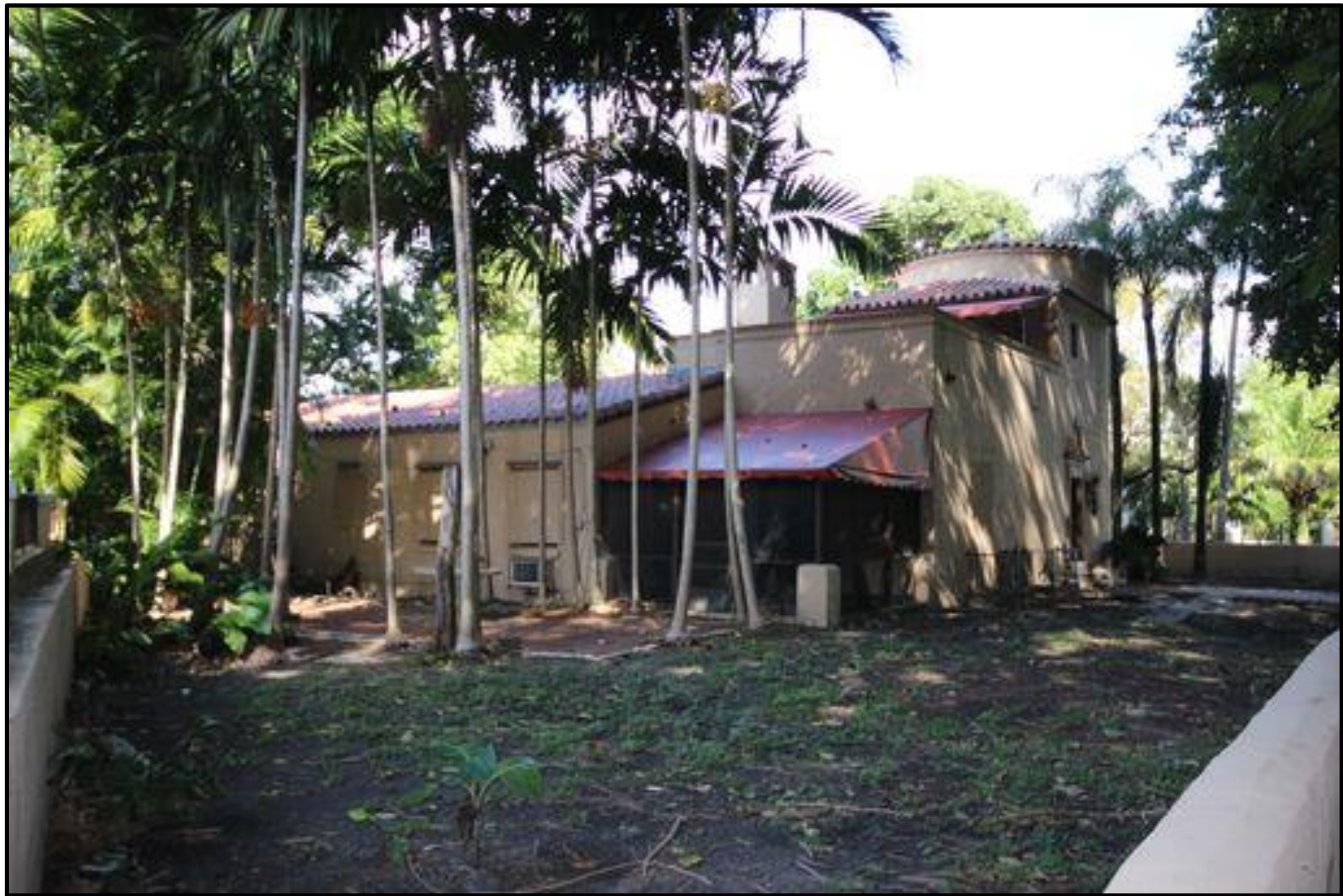
Southwest Corner (looking east) – Before
