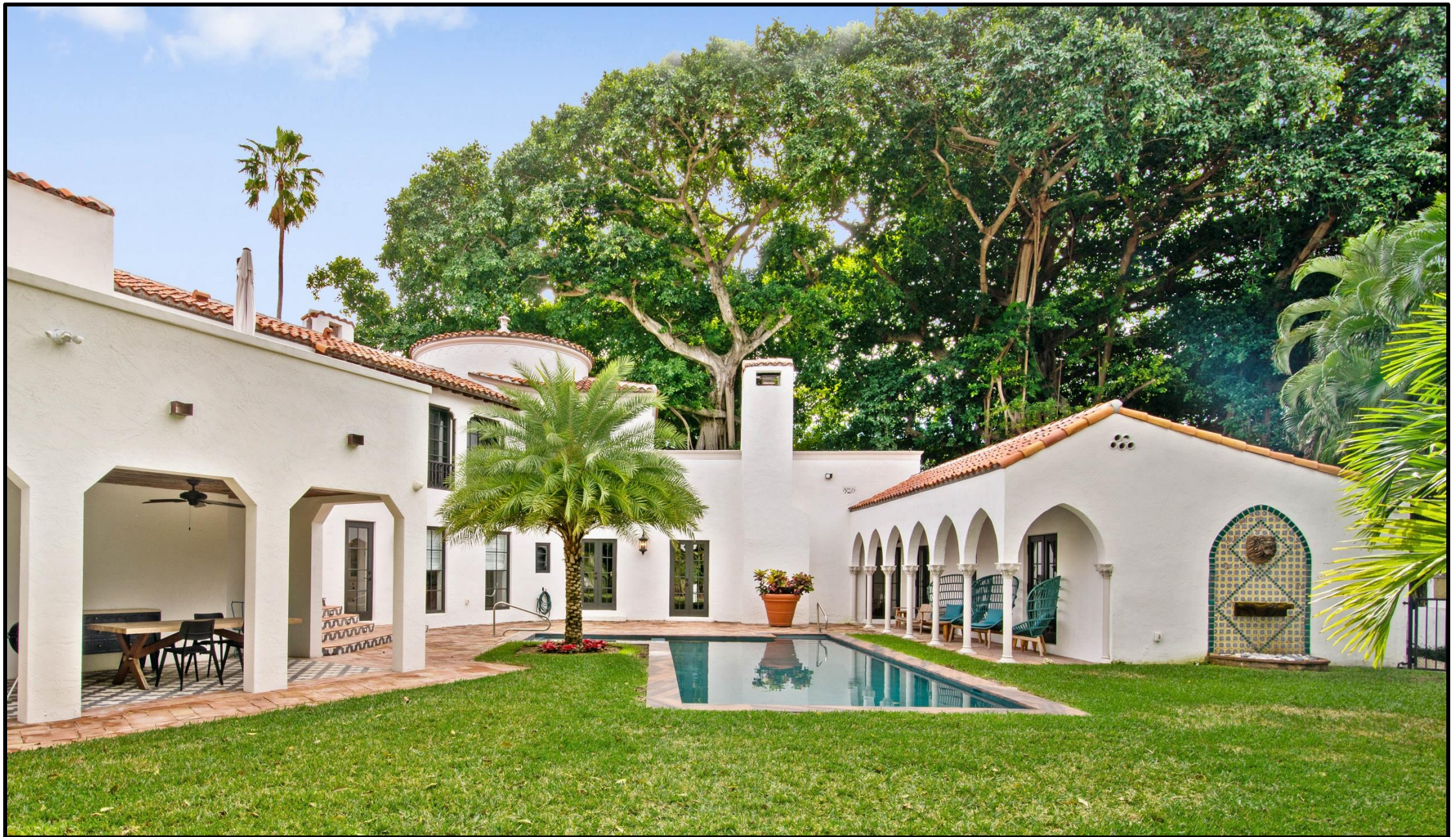
West and North (Rear) Facades – After
