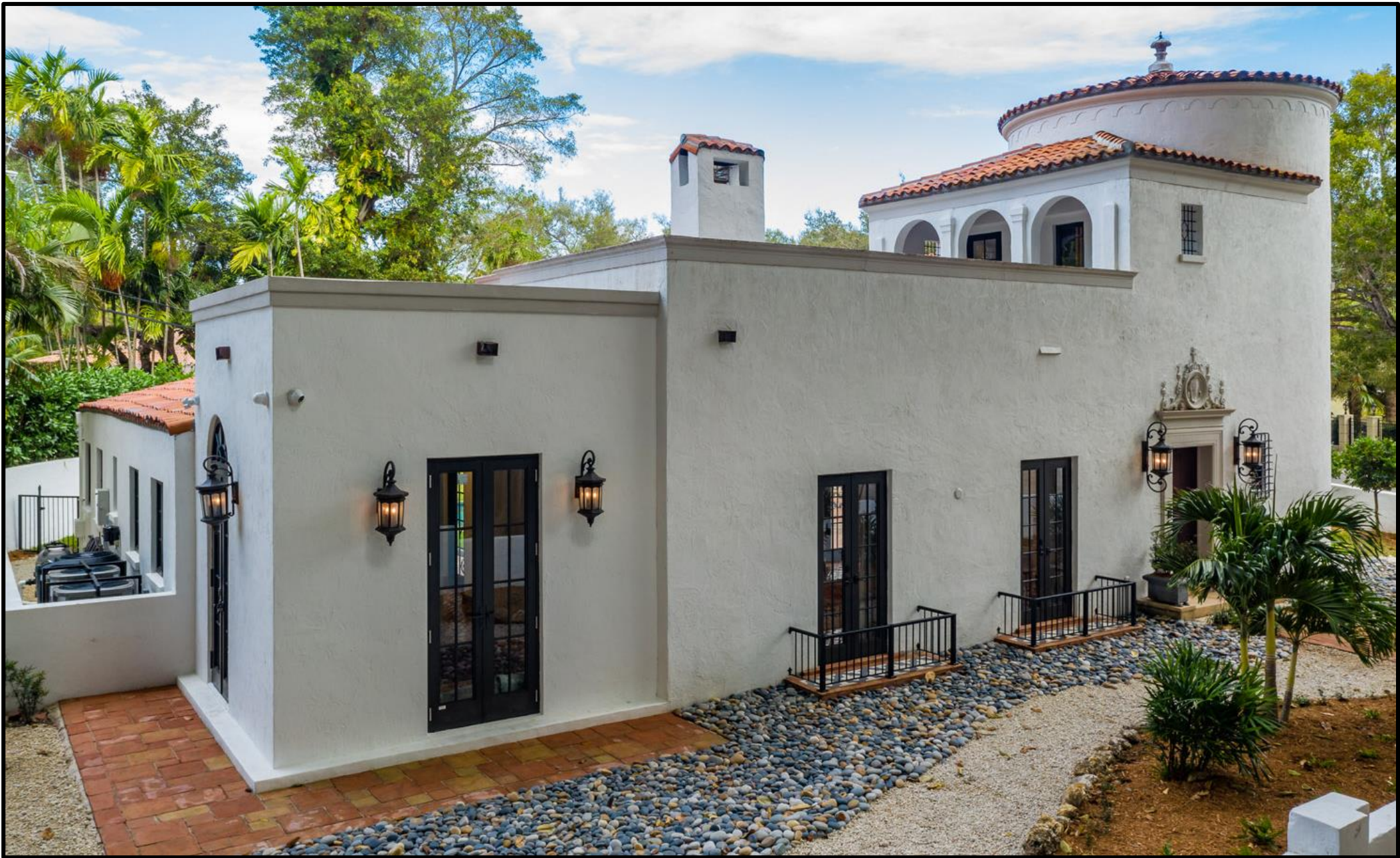
South (Front) Façade - After
