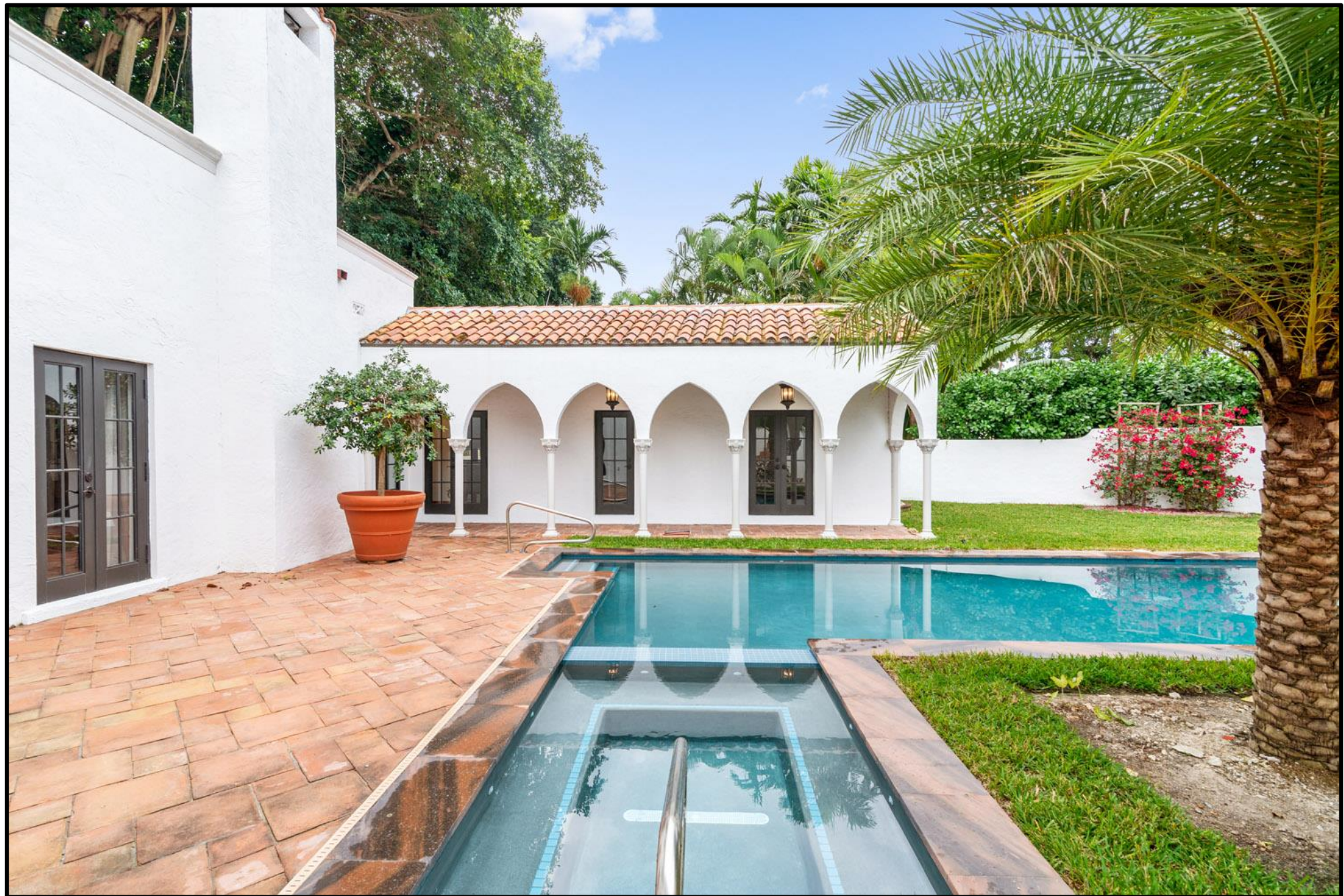
East (Rear) Façade – After
