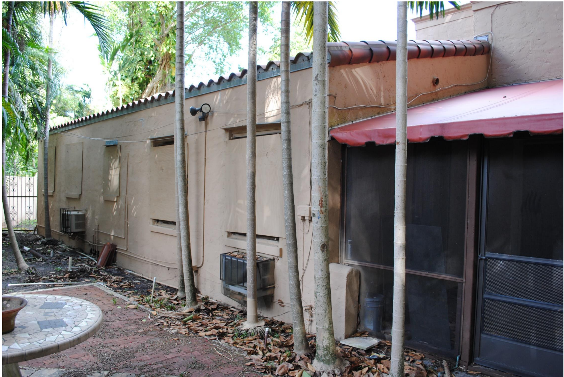
West Façade – Before
