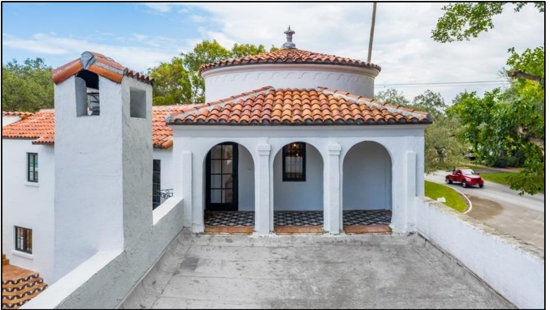
Second Floor Roof Terrace (looking east) – After
