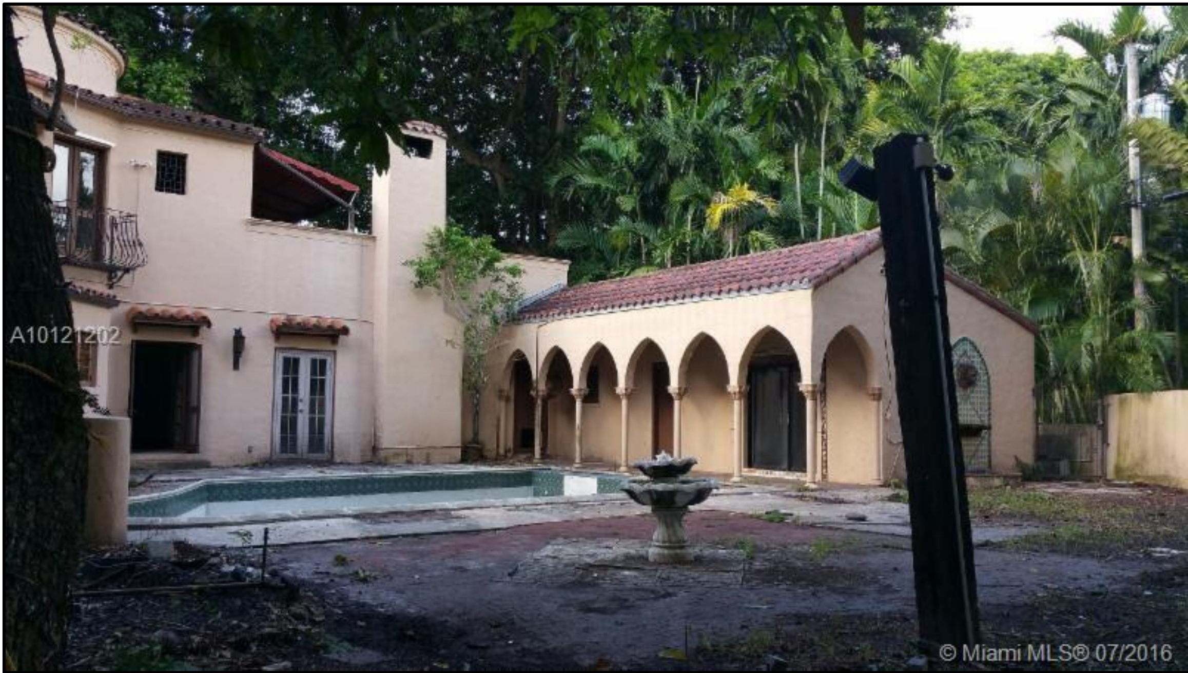
North and East (Rear) Façades – Before
