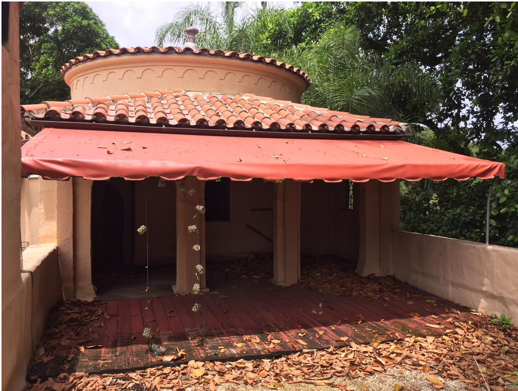
Second Floor Roof Terrace (looking east) – Before
