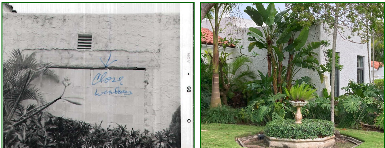
Figures 24: Removal of Window Feature: November 1968 [left]; 2025 [right] 1968 photo courtesy Miami-Dade Property Appraiser
