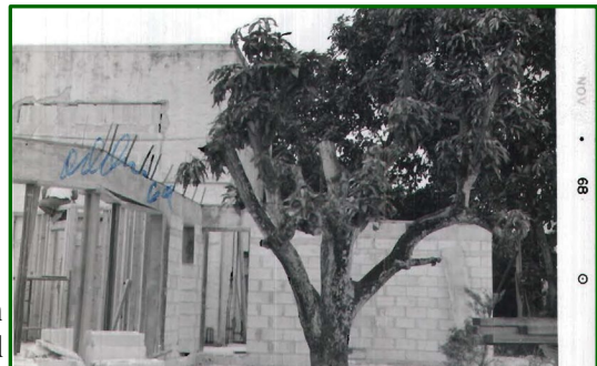
Figure 34: Addition Under Construction Note: 1923 accessory building in background
