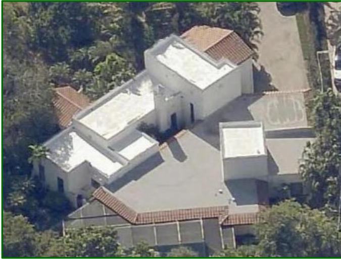
Figure 30: Aerial Photo Looking Southwest, 2024 Courtesy Miami-Dade Property Appraiser Figures 31: area at top right of photo Figure 32: area at bottom left of photo
