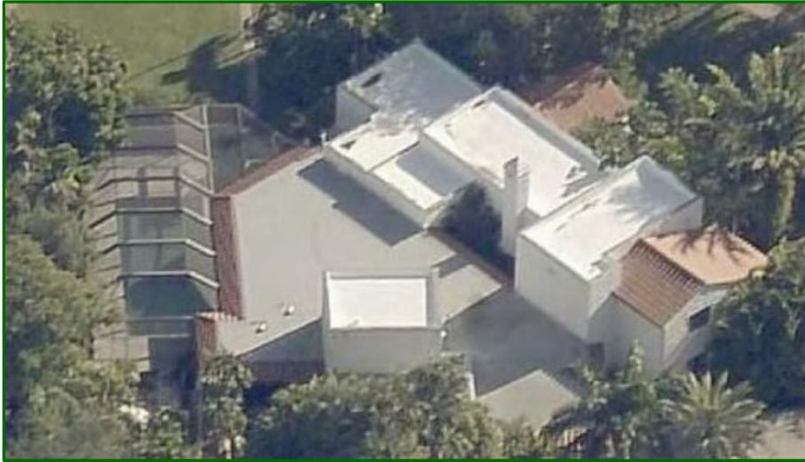
Figure 26: Aerial Photo Showing Position of 1923 Chimney, 2024
