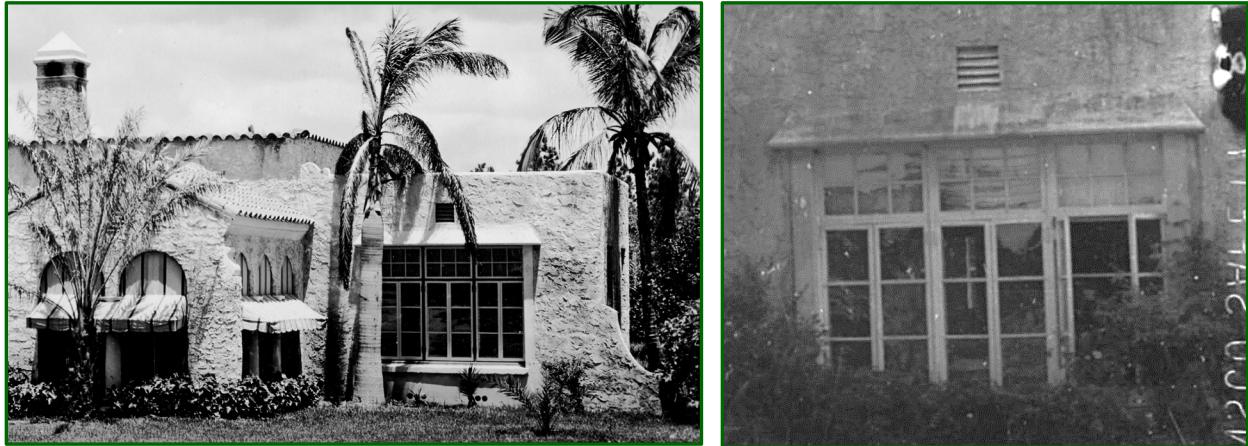
Figures 23: Eastern Bay Window Feature: 1925 [left]; c.1940 [right] Note: projecting sill & masonry frame [left] and swooped masonry hood [right]
