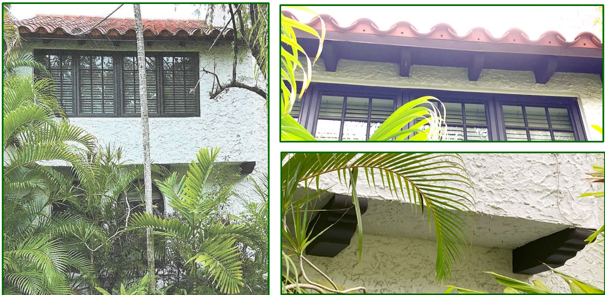
Figures 29: Southwest Corner: Arched Openings & Cantilever Addition, 2025
