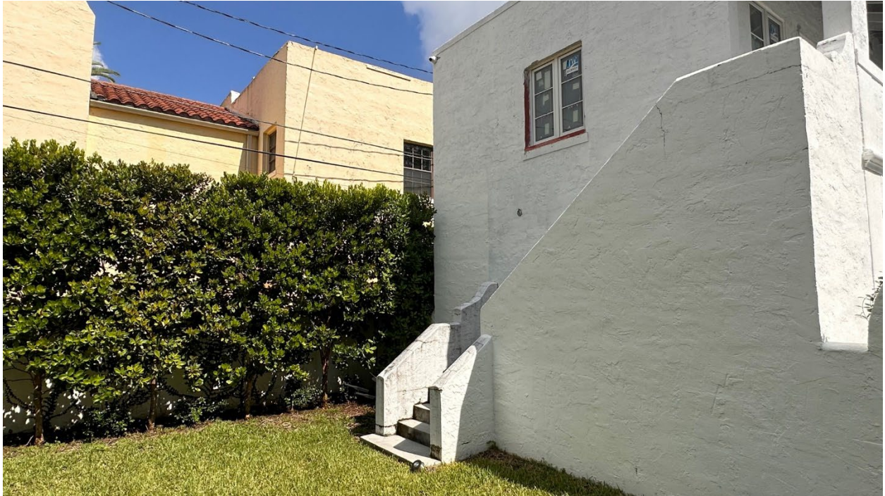
GARAGE BUILDING STAIRS
