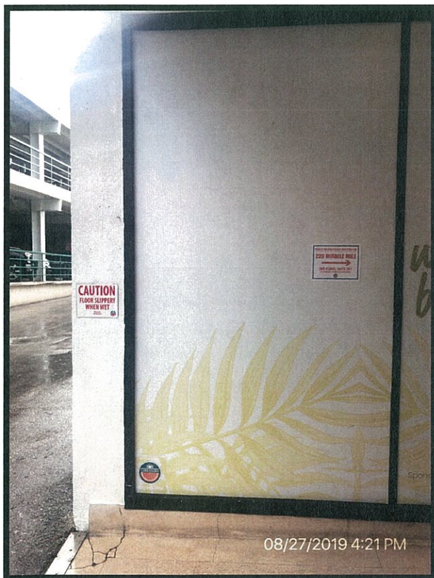
Sign located on SW wall of breezeway
