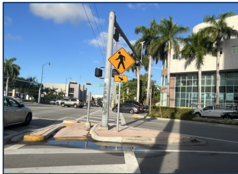
Photo 23: Issues with Orientation of W16-7P Plaque
