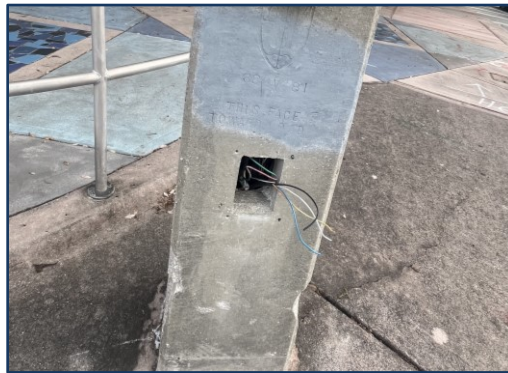
Photo 5: Exposed Wires (Upright NE Corner)
