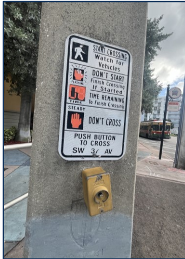
Photo 4: Pushbutton tilted and Sign faded (NE corner)
