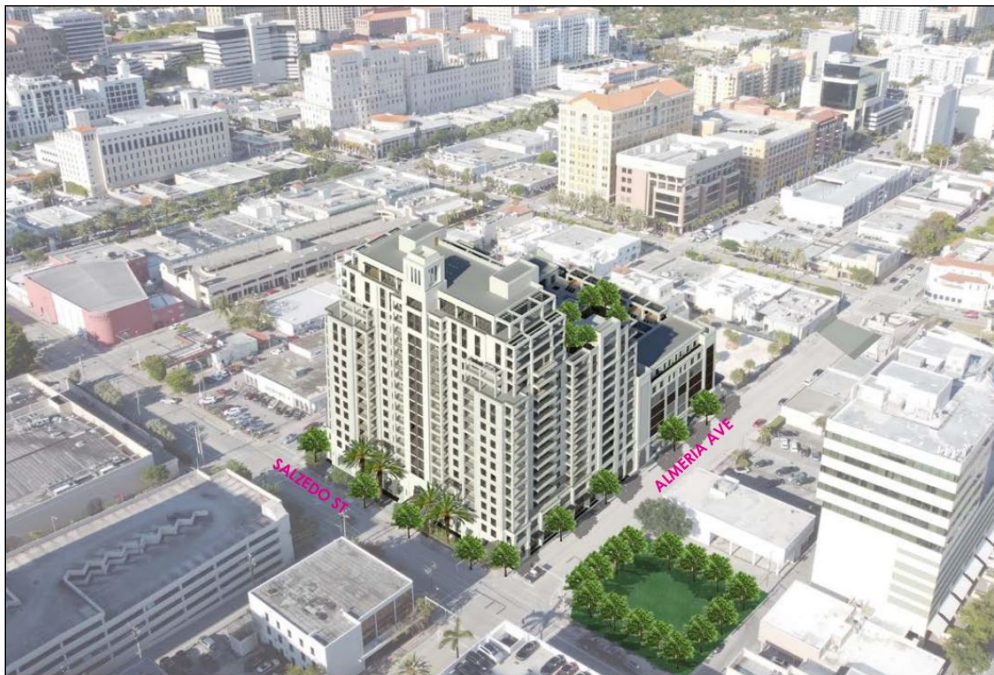
Proposed project and existing conditions
