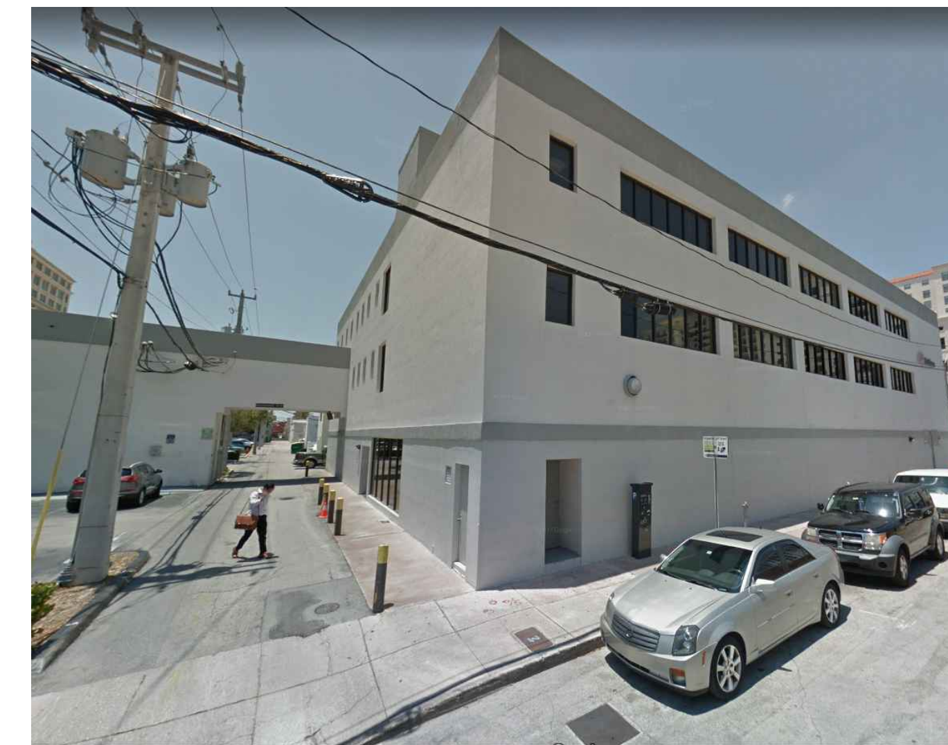
3. EXISTING BANK BUILDING - FROM GALIANO
