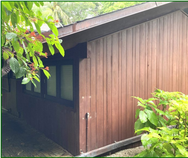
Designed Wood Features: Random Width Vertical Cypress Siding [left]. Craftsman Features such as rafter tails with detailed ends [right], craftsman knee braces, projecting beams, cedar roof shingles
