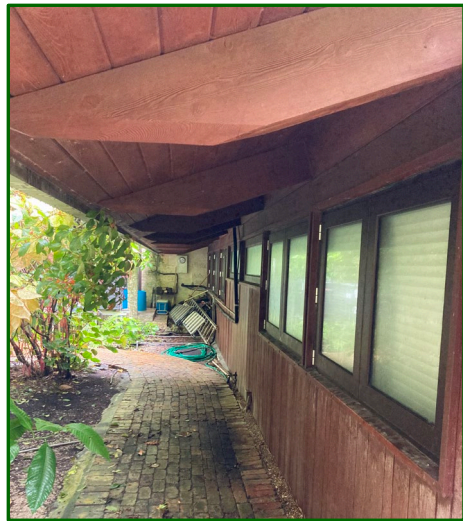
Designed Wood Features: Random Width Vertical Cypress Siding [left]. Craftsman Features such as rafter tails with detailed ends [right], craftsman knee braces, projecting beams, cedar roof shingles
