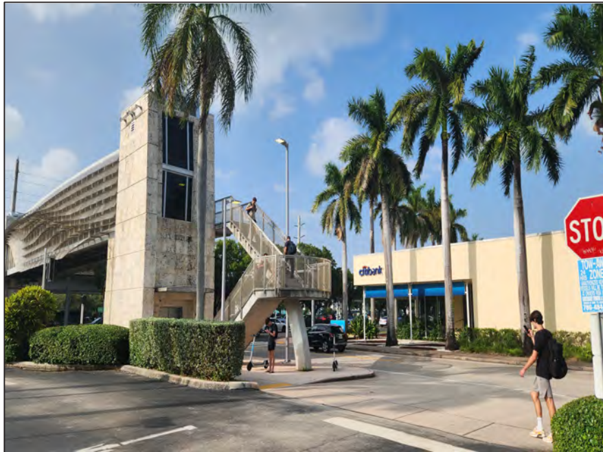
US-1/South Dixie Highway at Mariposa Court, South Leg (Facing North): Moderate to high pedestrian activity was observed at the pedestrian bridge.
