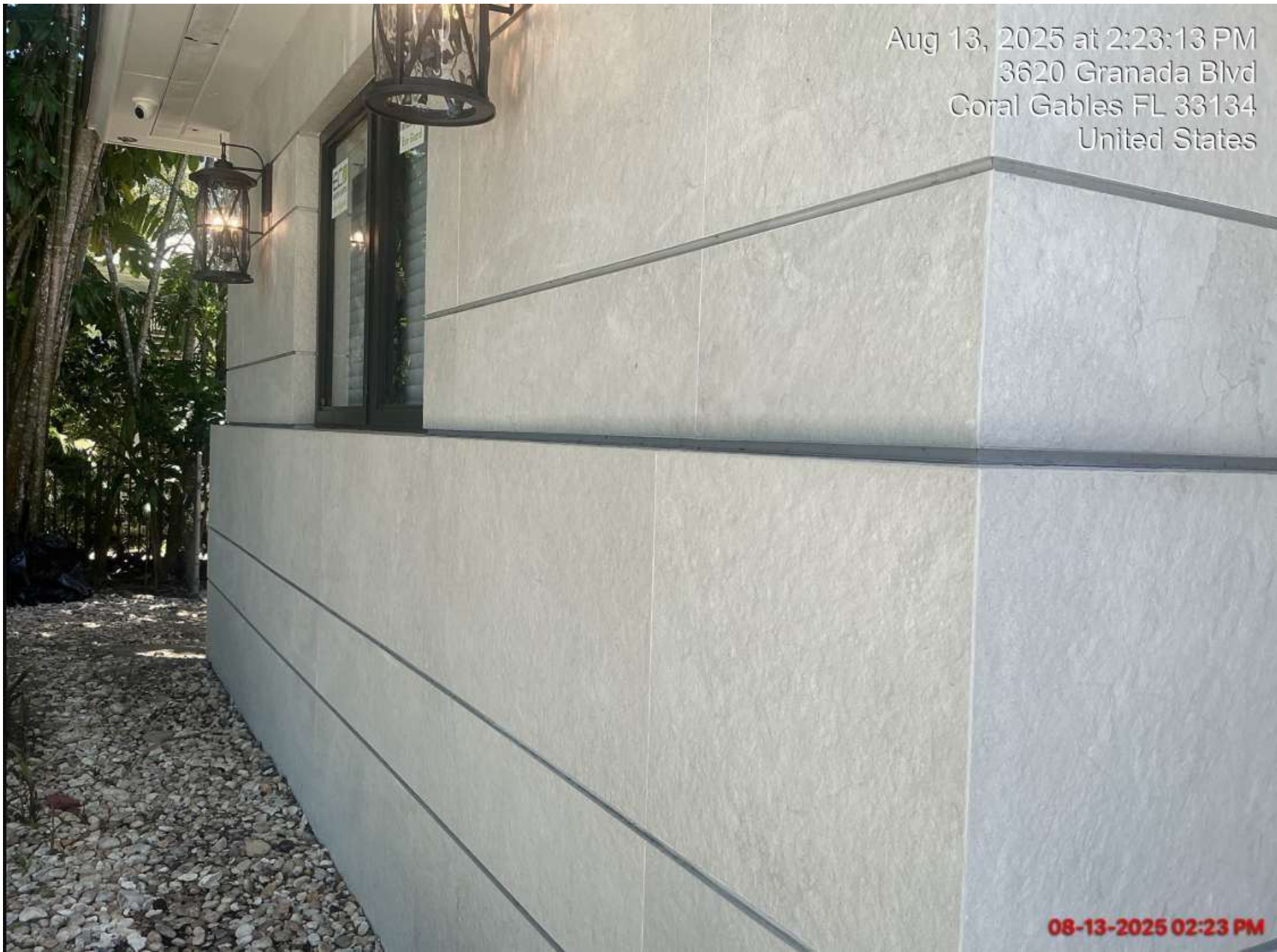
FRONT FAÇADE WALL ALTERED W/ STONE TILE CLADDING
