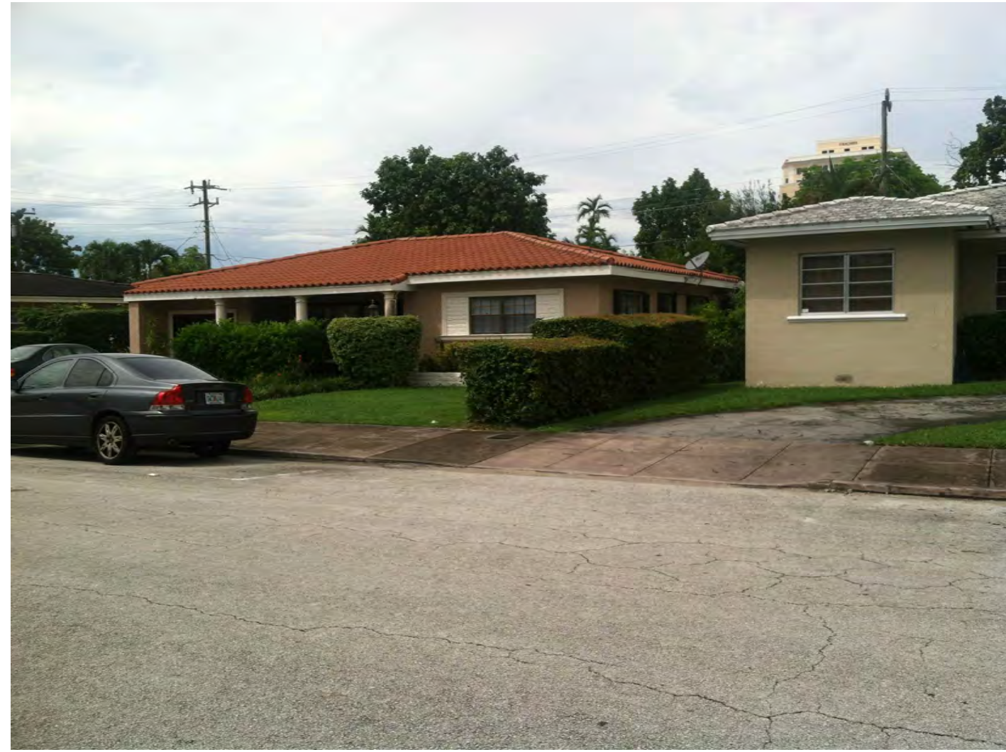
VIEW OF NEIGHBOR TO THE WEST
