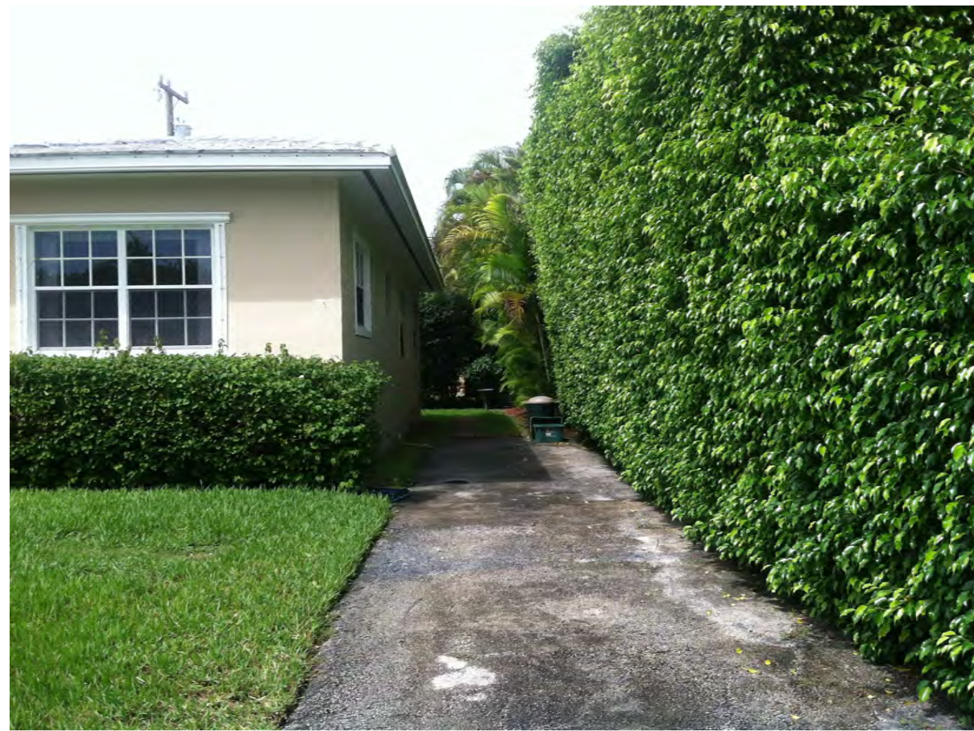
311 SANTANDER - VIEW OF EAST SETBACK FROM FRONT OF PROPERTY
