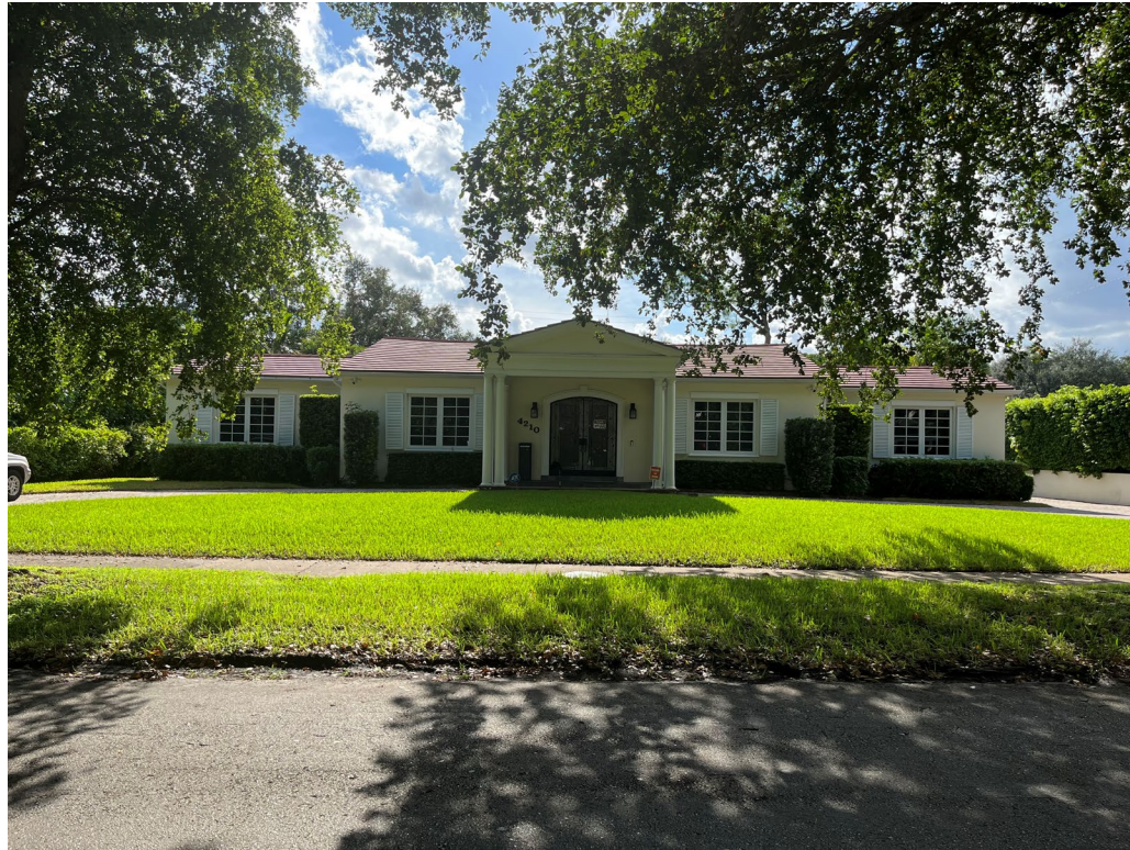
Existing House. Front view.
