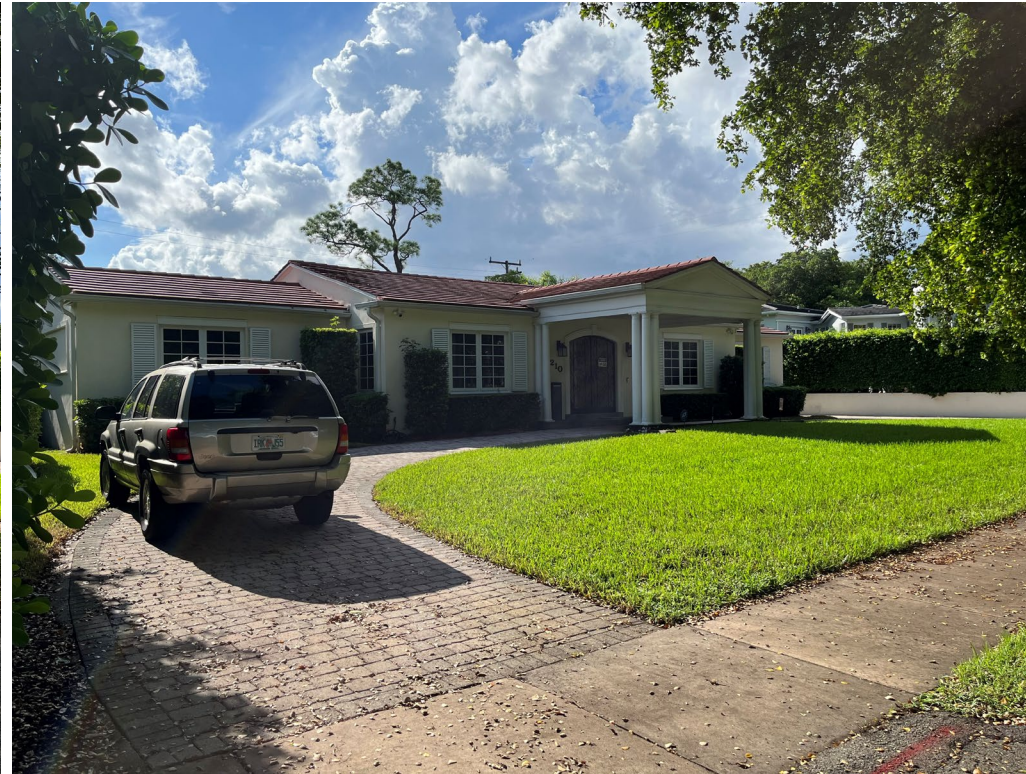
Existing House. Front view.
