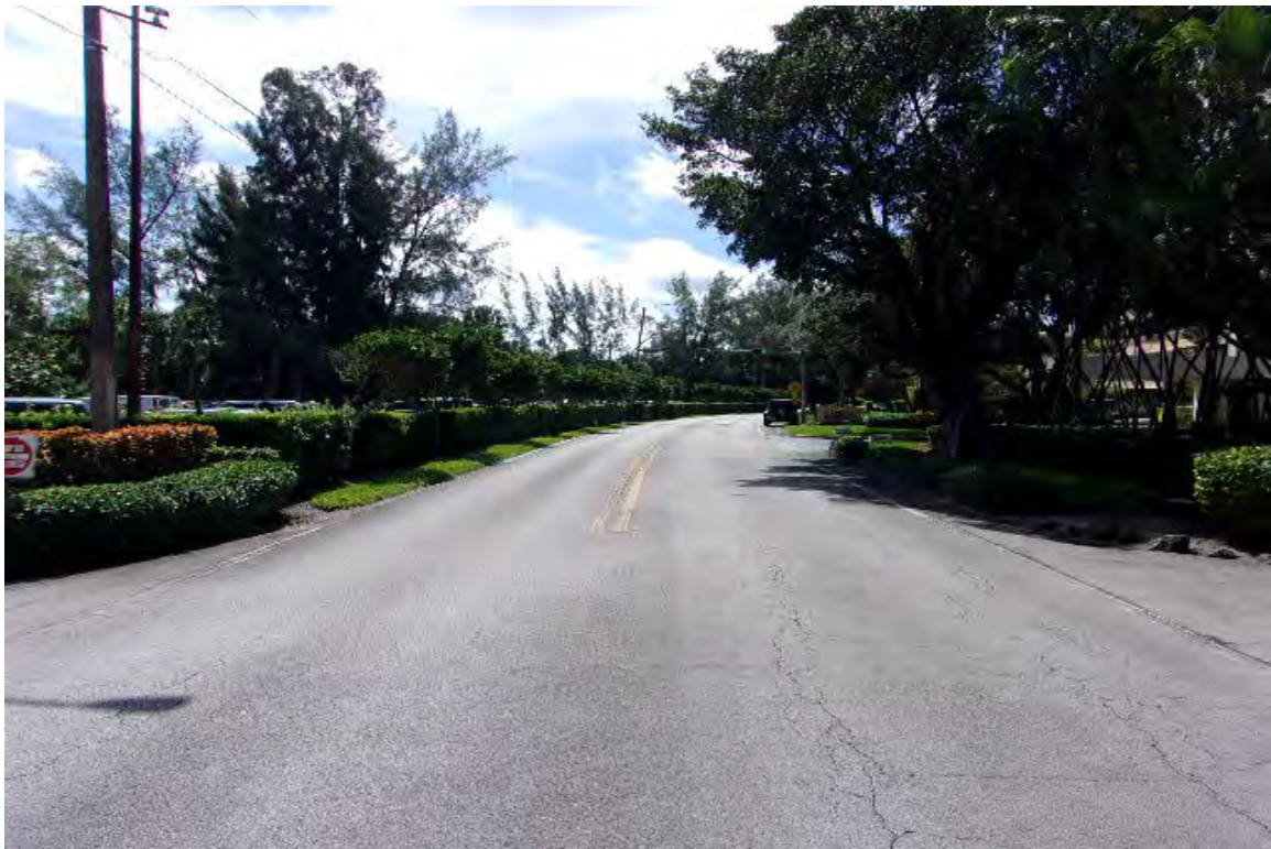
LOOKING SOUTHERLY ON UNIVERSITY DRIVE– SUBJECT TO LEFT
