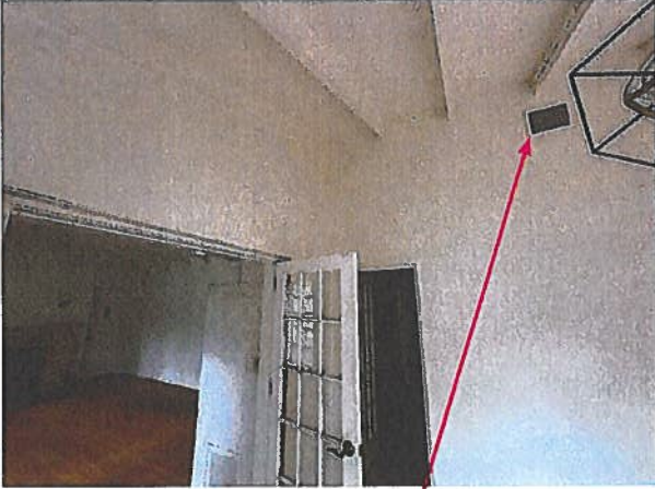
Air vents added when porch enclosed.
