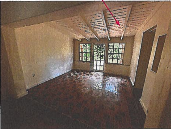
Rear courtyard originally screened in, and now opened into the home. New tile looks laid, and AC added in room.
