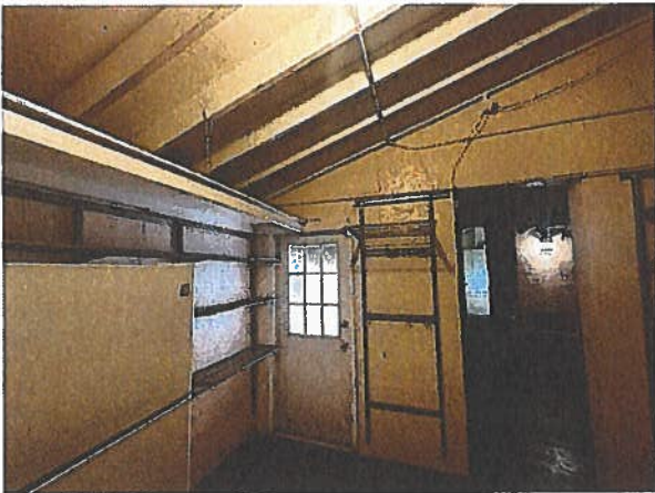
Rear of new garage extension.
