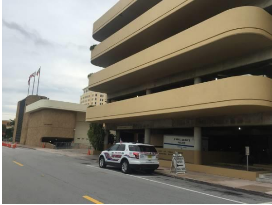
Looking northwest along south elevation.
