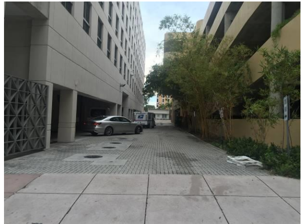
Looking south along east elevation and alley between Sevilla Avenue and Palermo Avenue.
