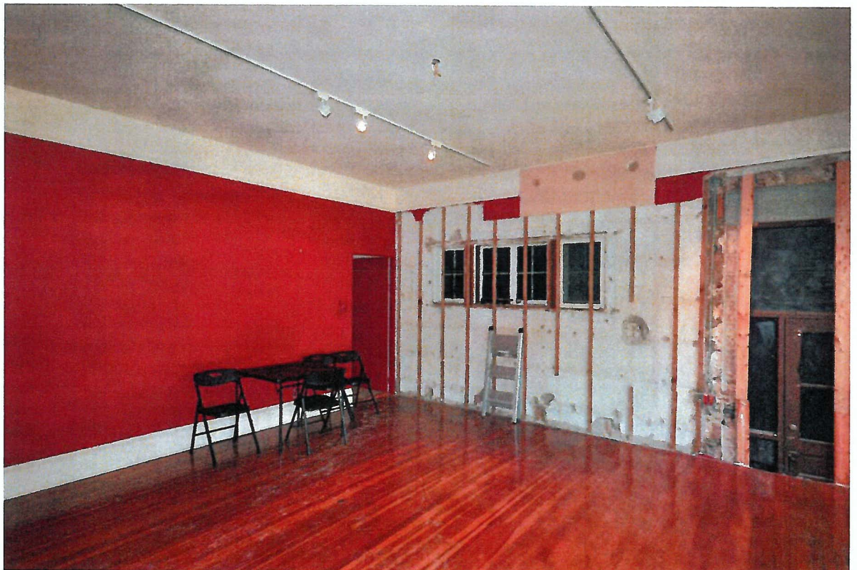
20. Dining Room Looking Southwest
