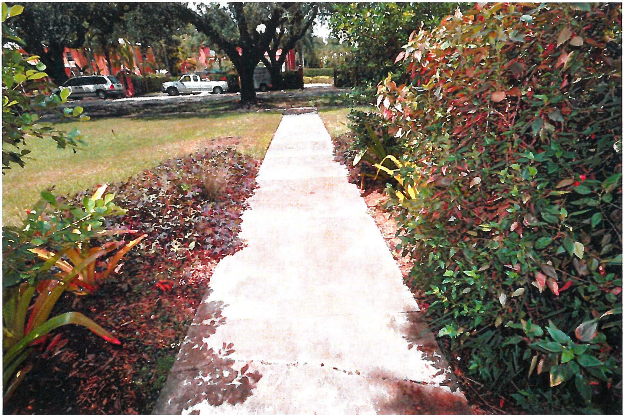
46. Existing Front Sidewalk
