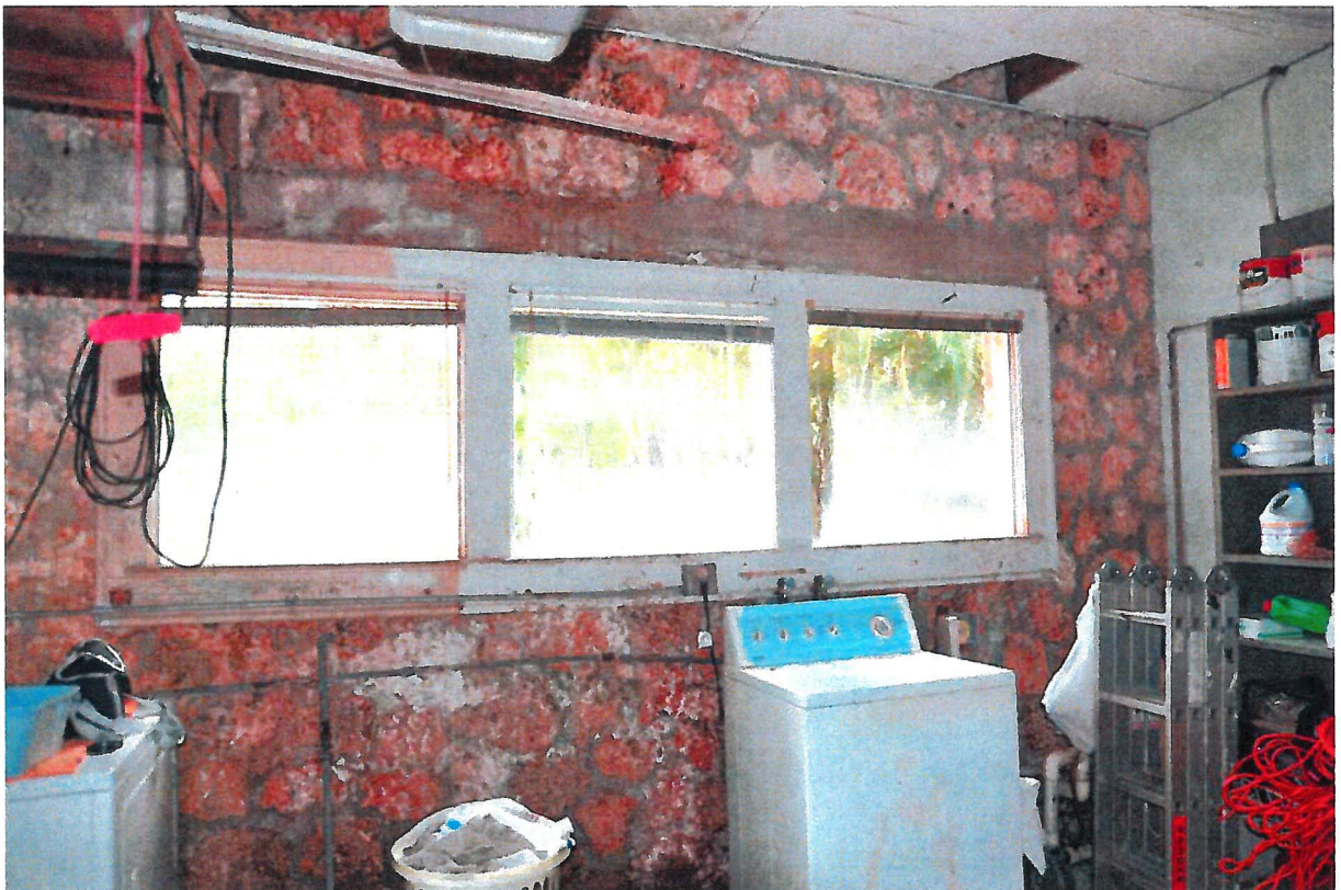
42. Garage Interior Looking East
