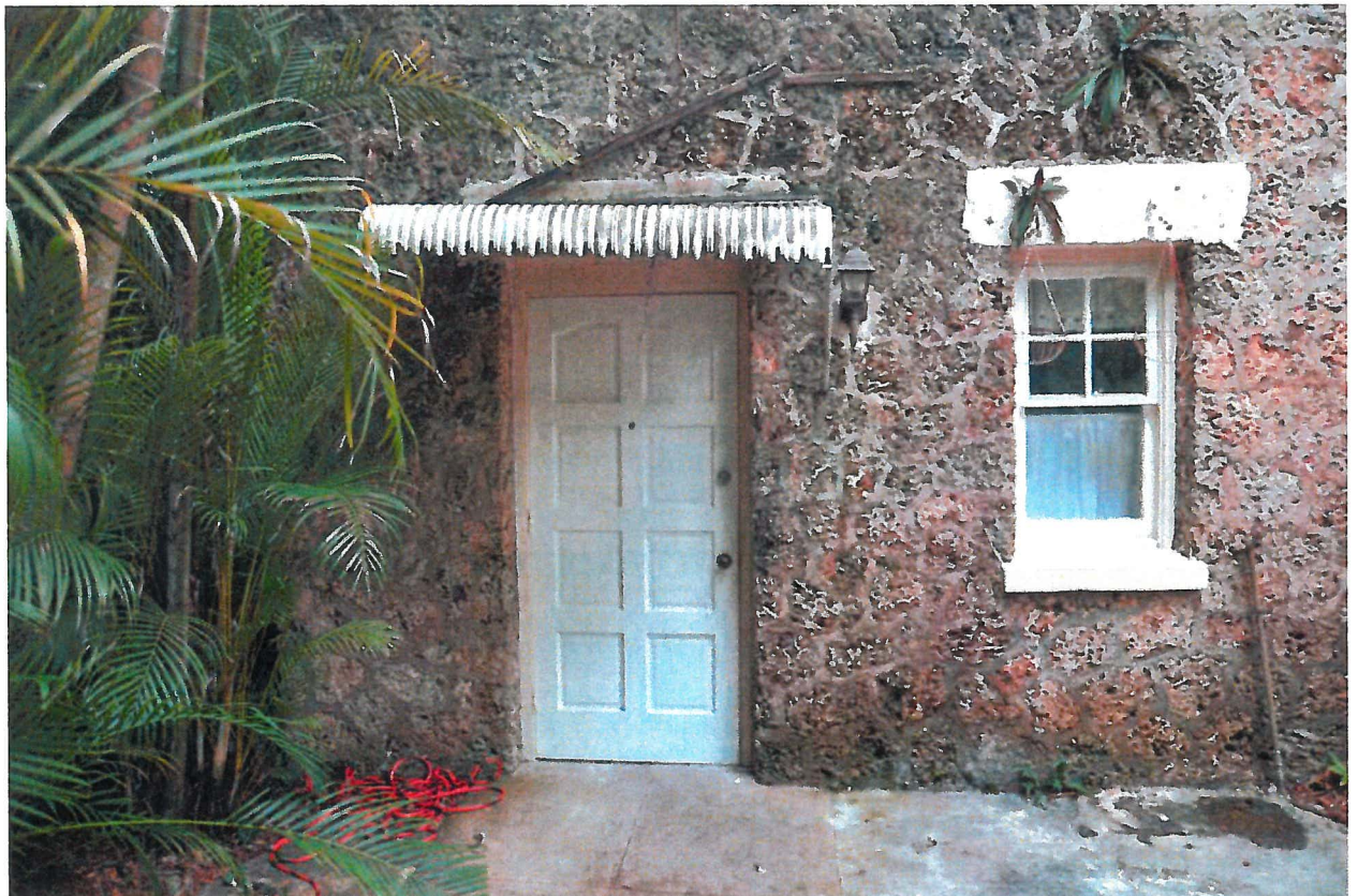
6. East Façade of Existing Garage Detail
