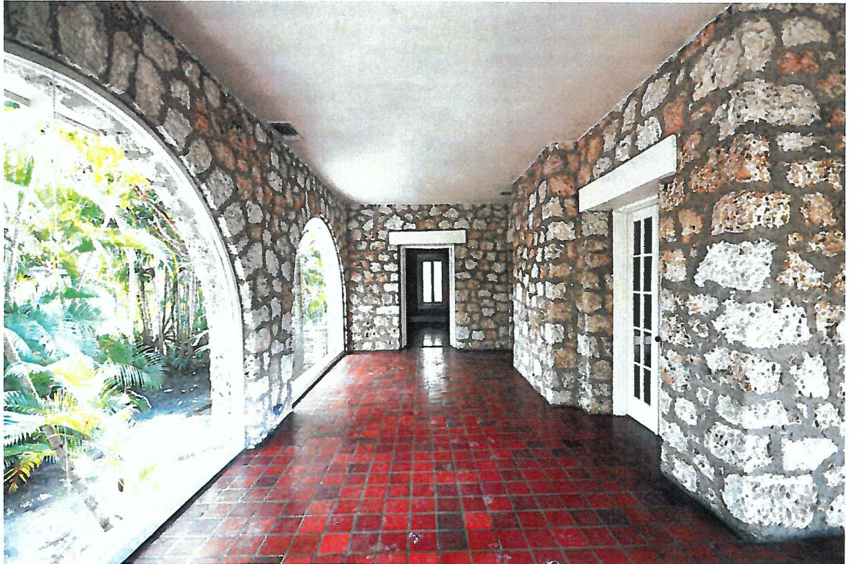
24. Northwest Florida Room (Looking Southeast)
