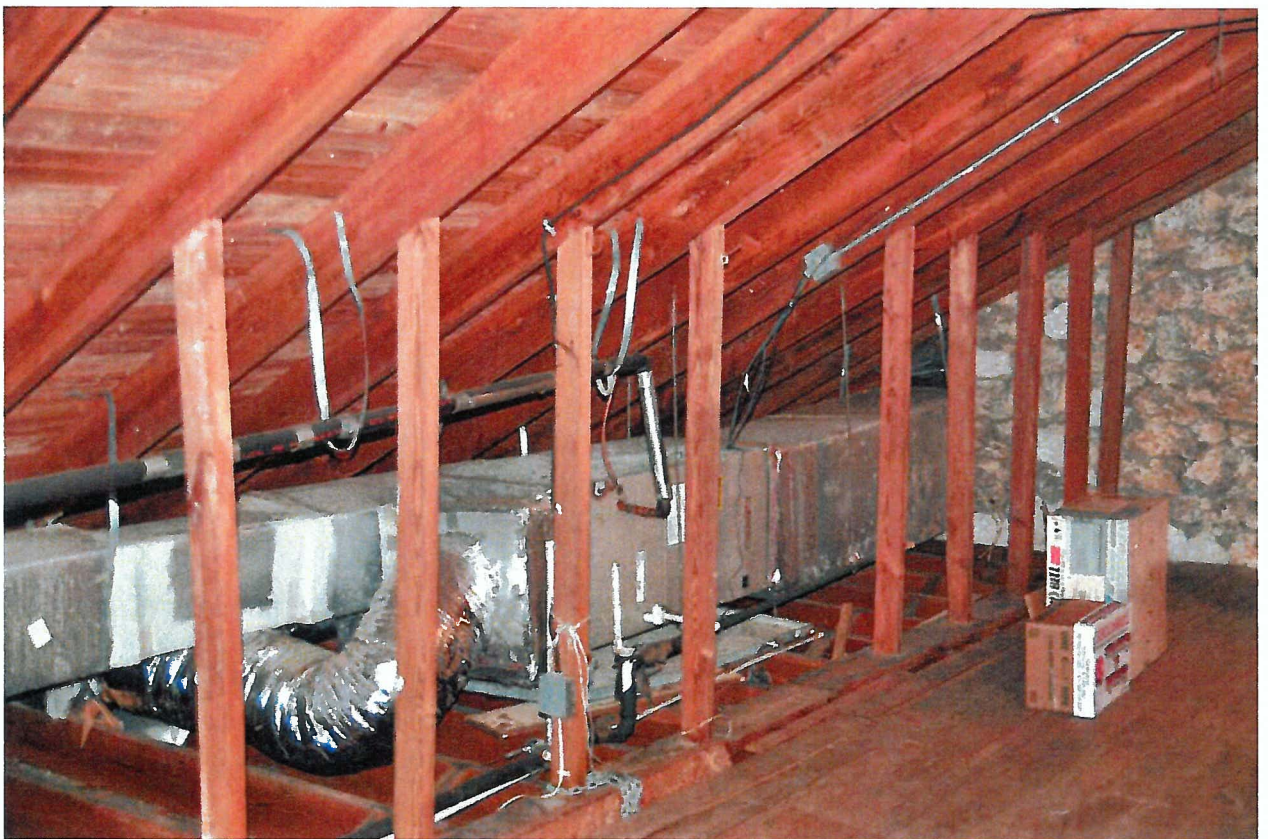
40. Attic Looking North
