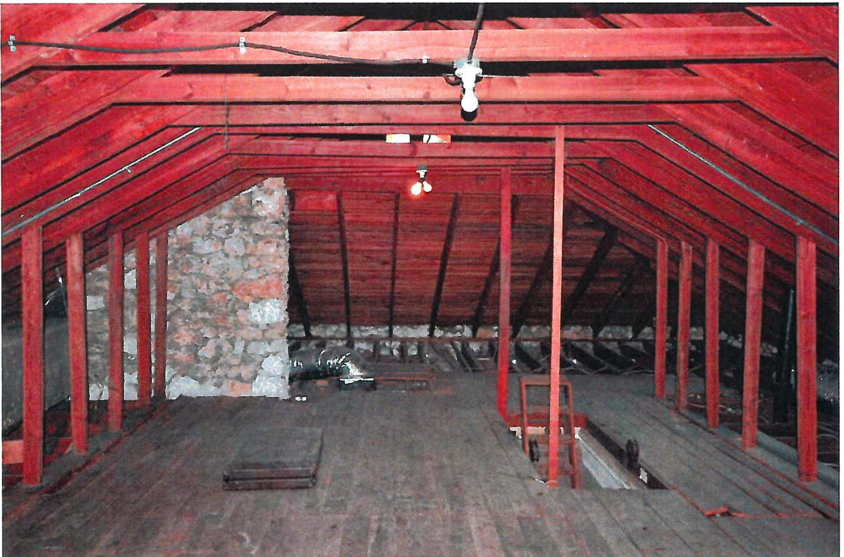
38. Attic Looking East
