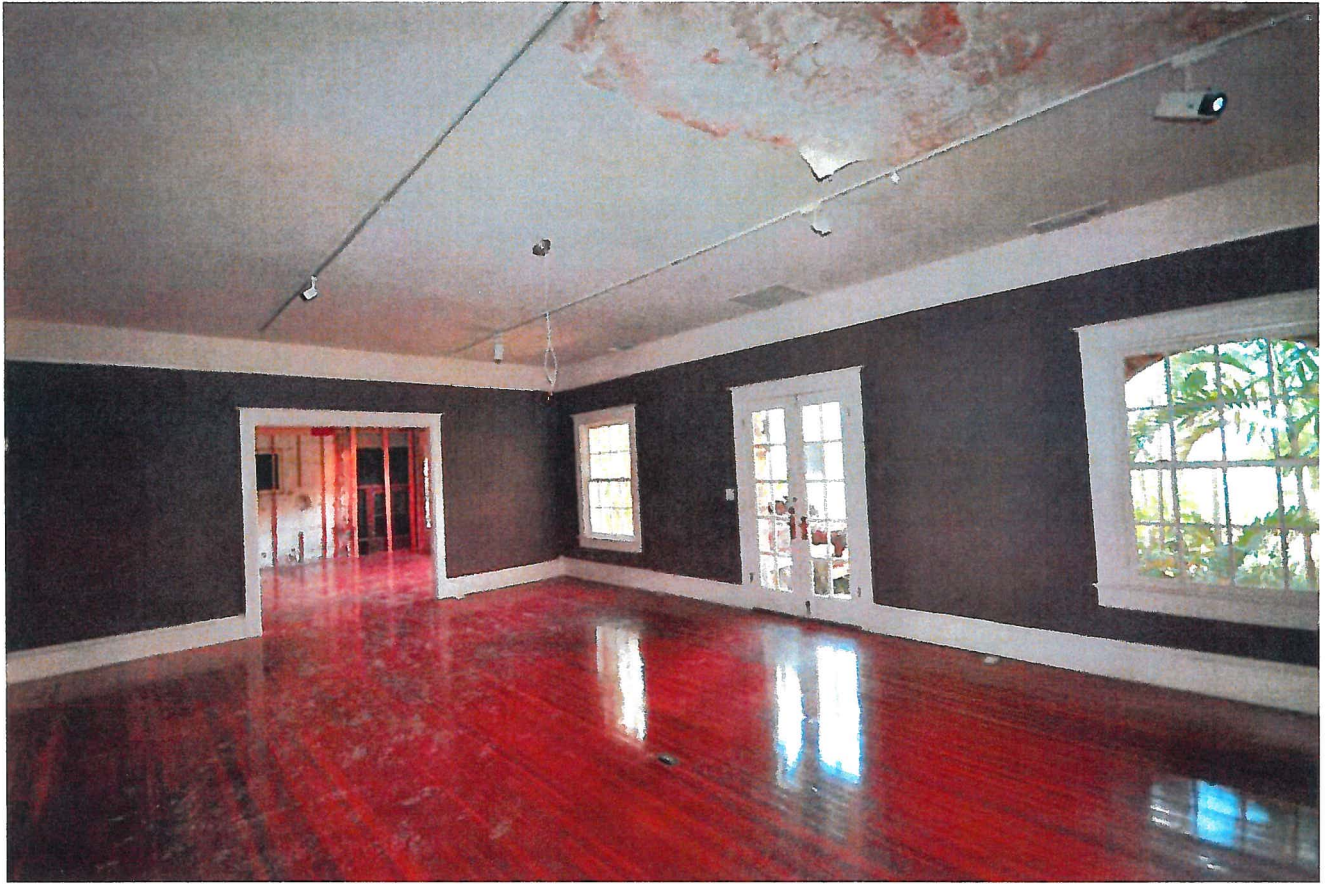
17. Living Room Looking Northwest
