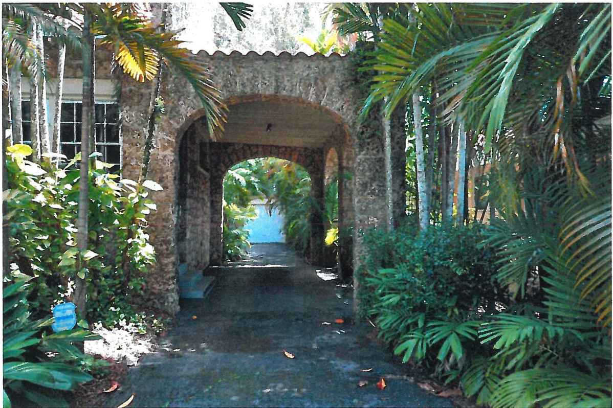
2. North Façade - Carport
