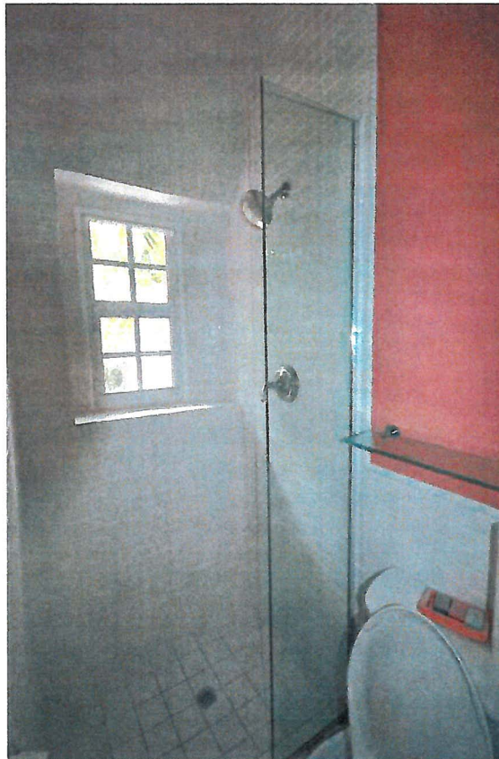
34. Southwest Bathroom Looking Southwest
