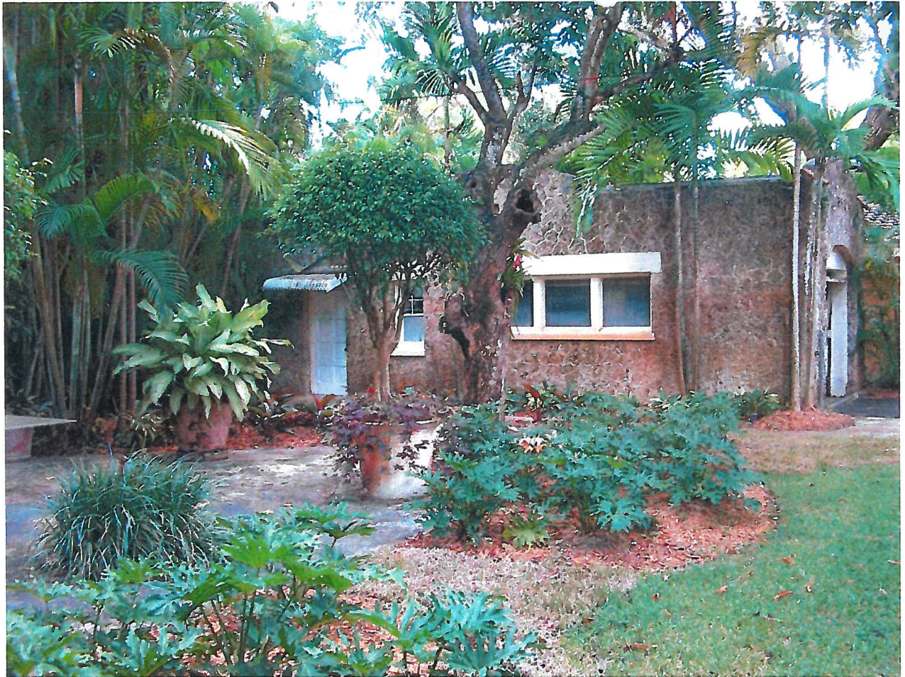
5. East Façade of Existing Garage
