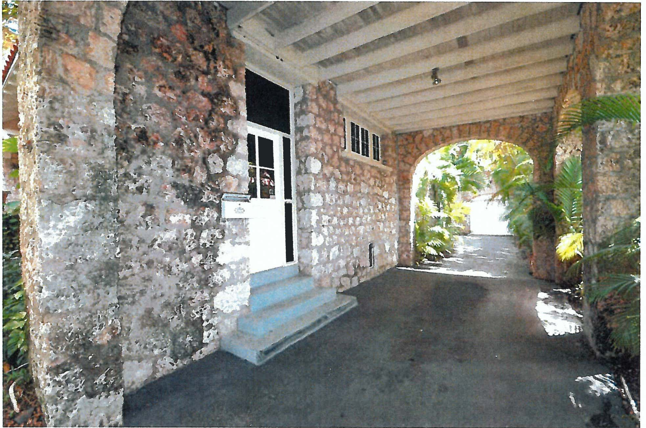
11. Exterior Carport at West
