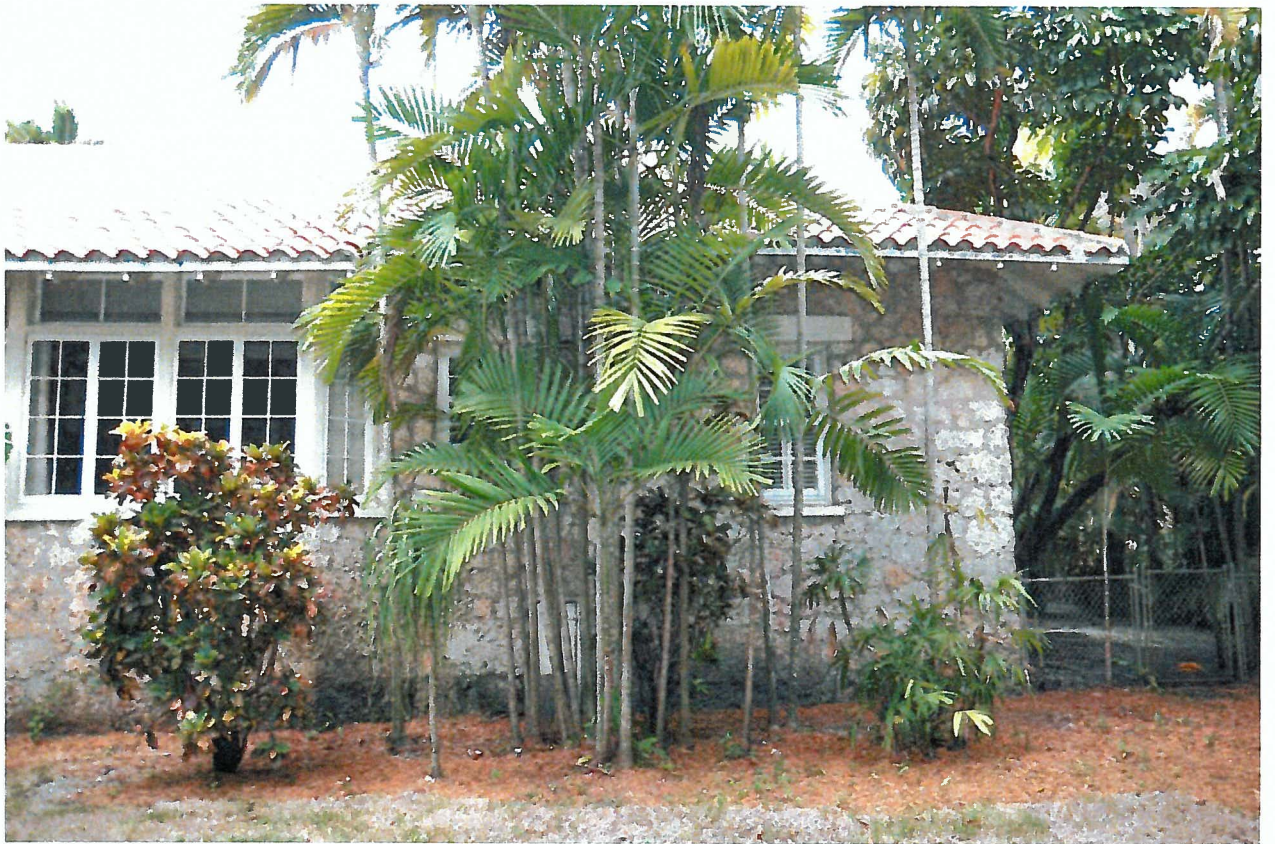
8. Southeast corner of Existing Residence
