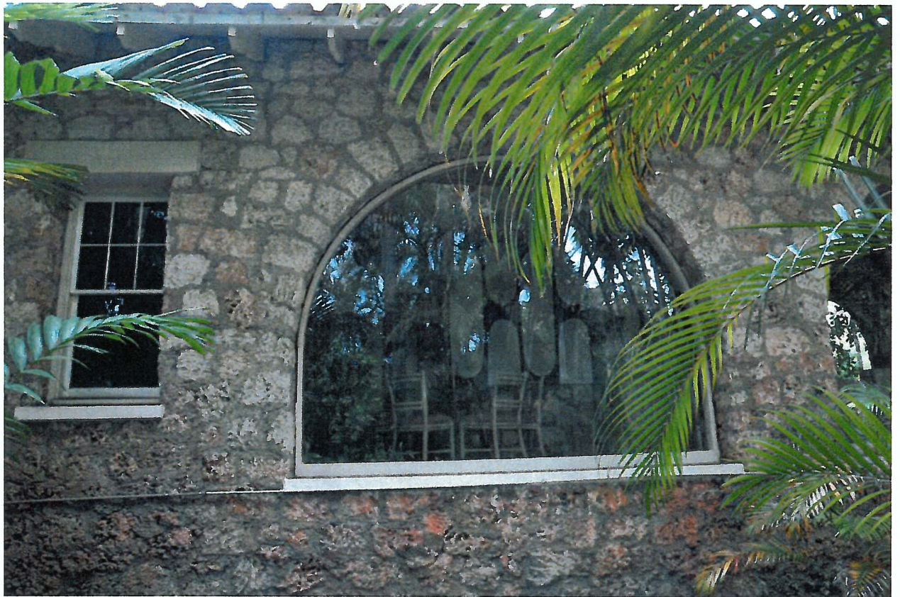
4. East Façade Detail of Existing Windows
