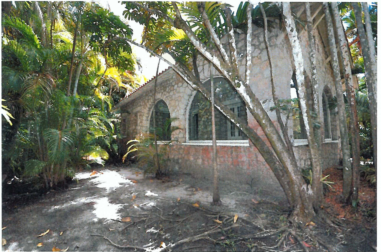
3. East Façade of Existing Residence
