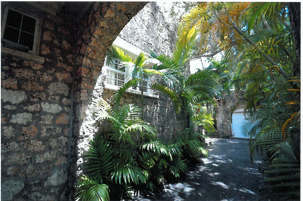
12. West Elevation Beyond Carport
