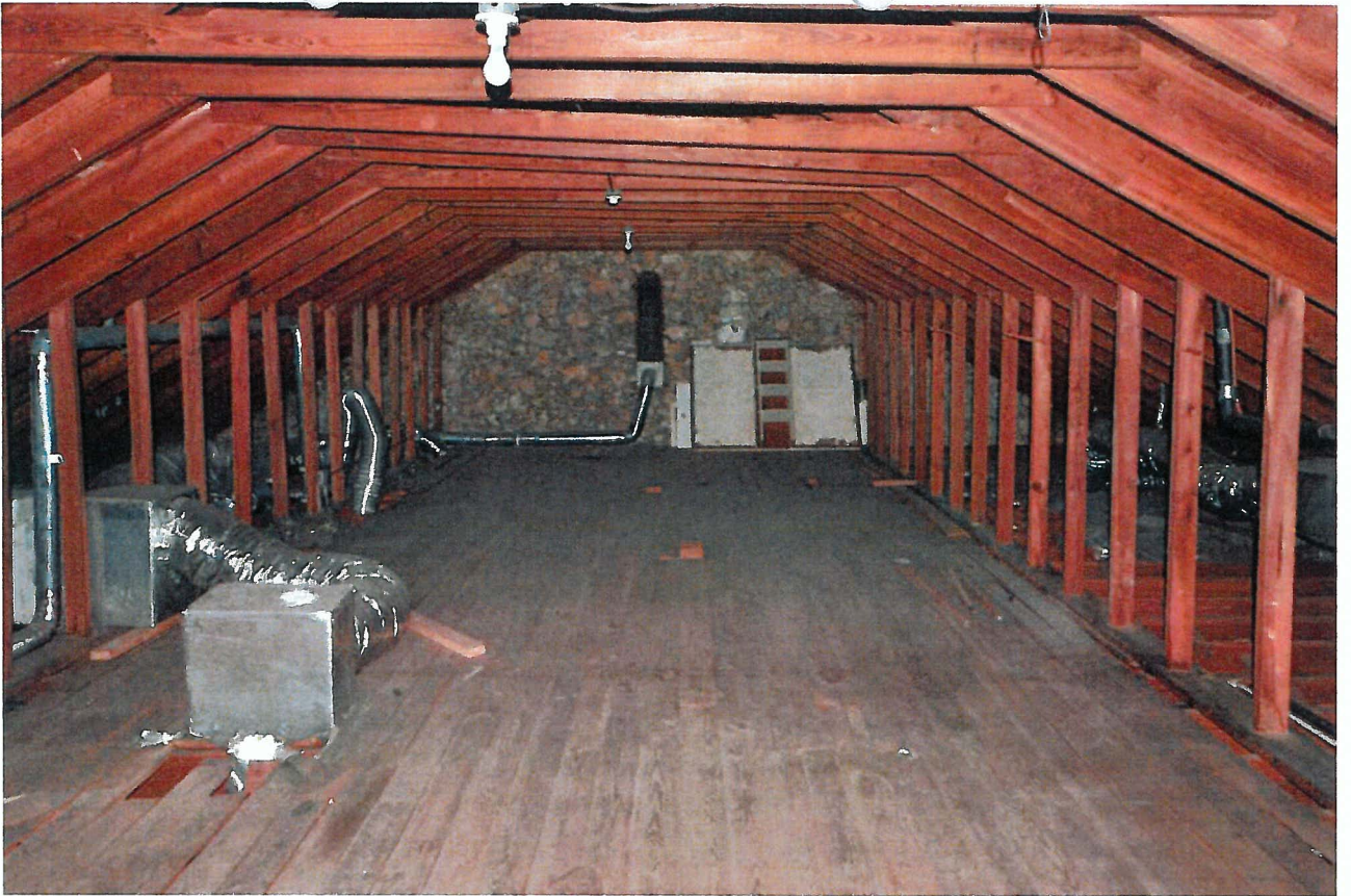
39. Attic Looking West
