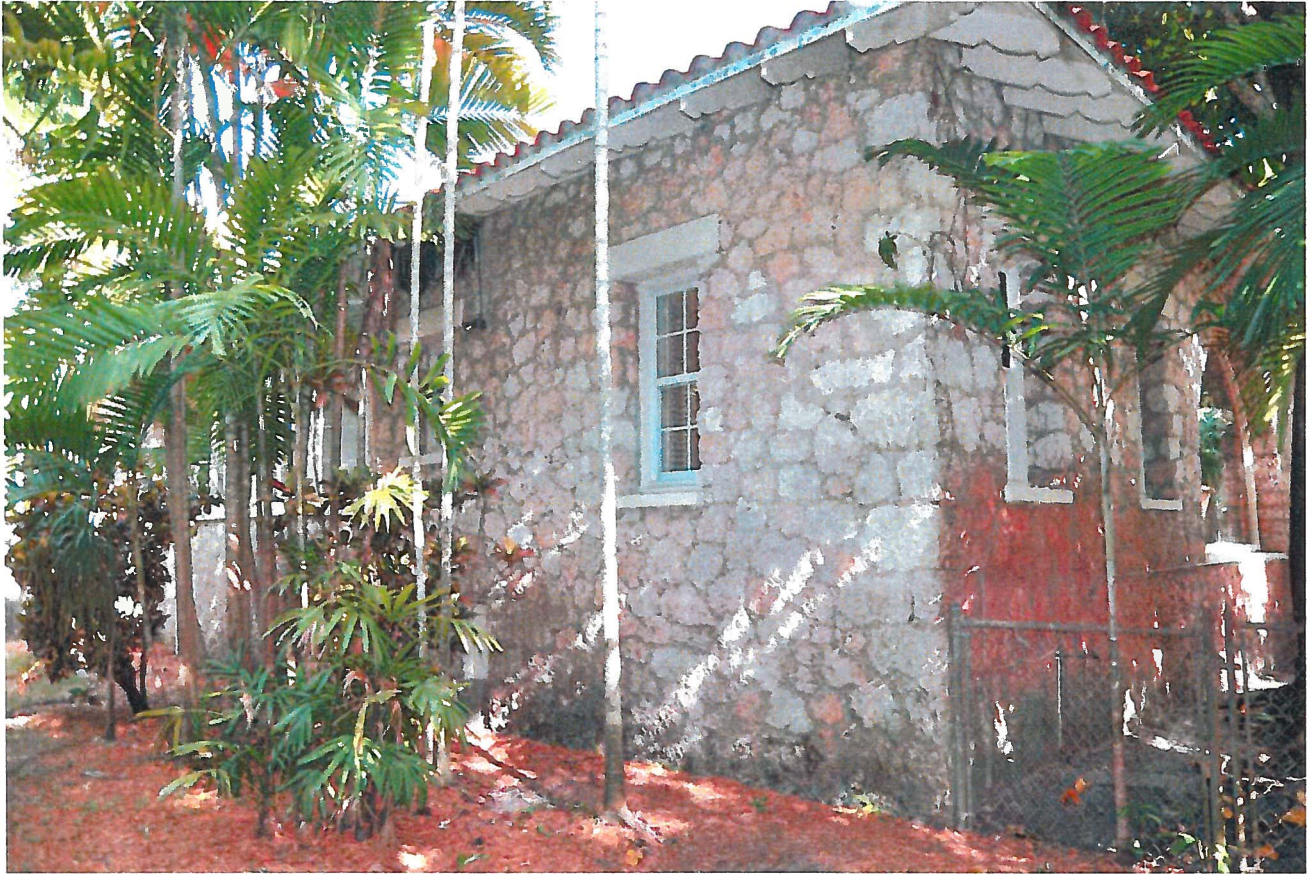
9. Existing Southeast Corner
