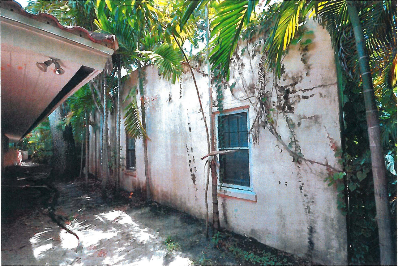
13. West Elevation of Existing Garage
