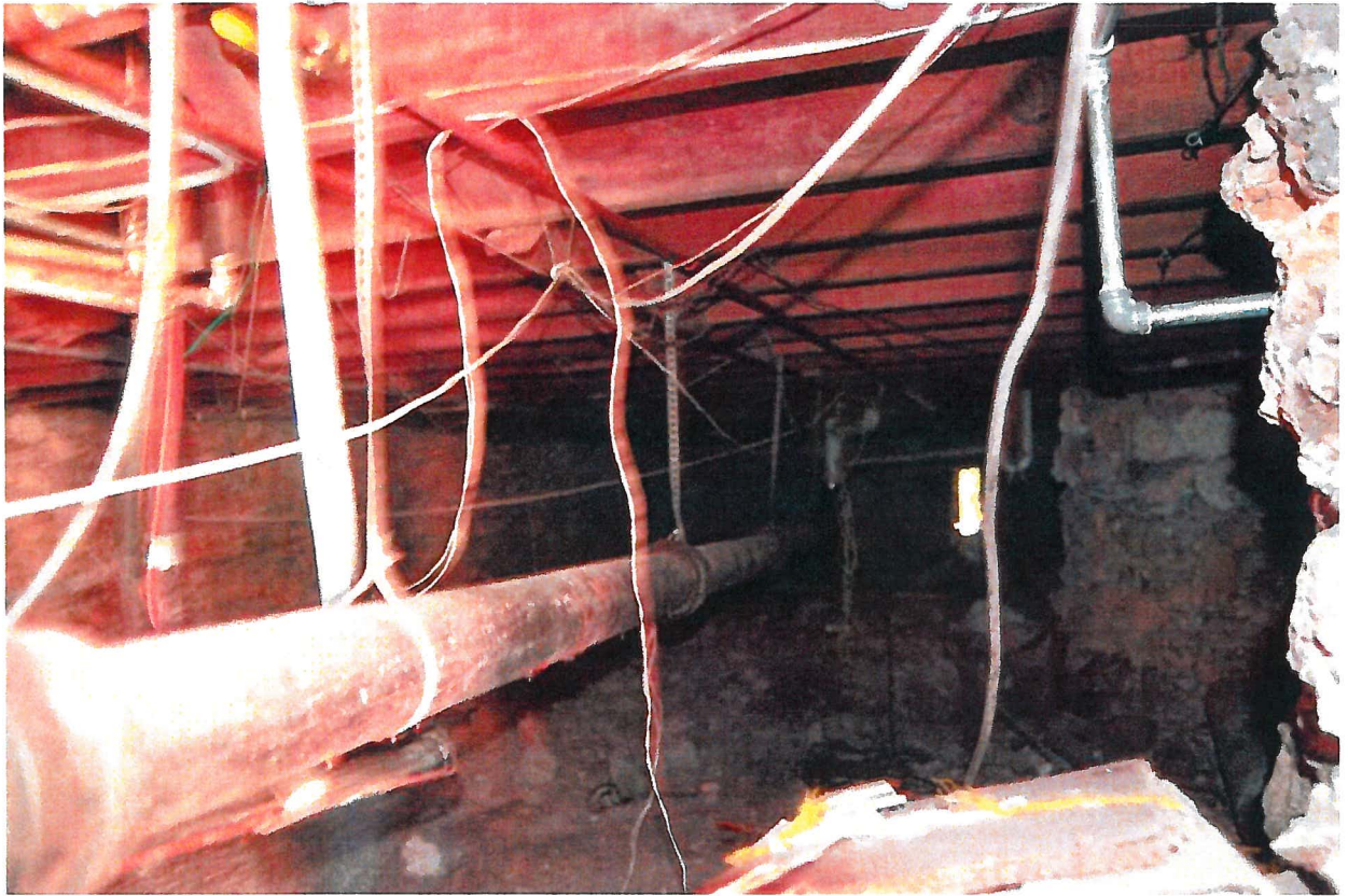
41. Existing Crawl Space
