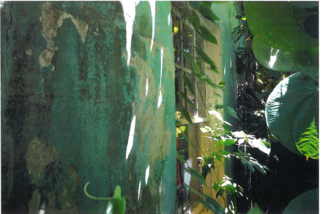
10. South Façade of Existing Building
