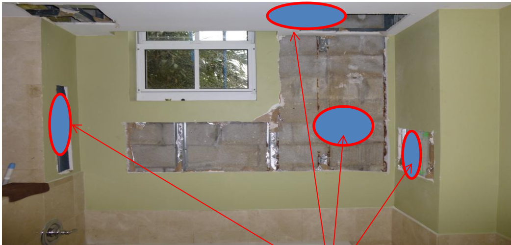
60% Moisture on Concrete block Wall
