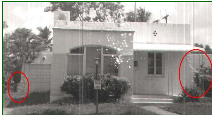
Figure 23: Historic Photo, 1967 Red circles: Wing Walls
