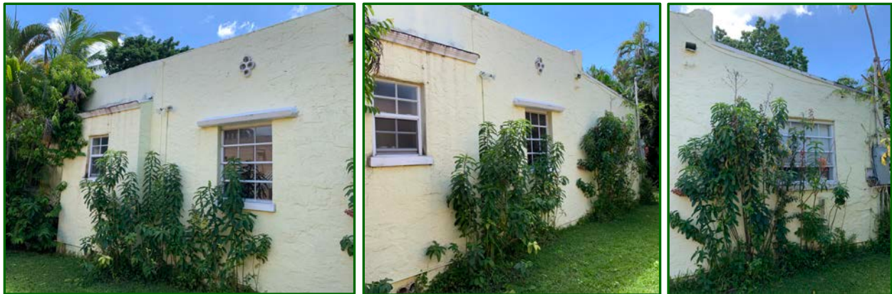
Figures 28: East Façade: Permit #402, 1923 [top] 2022 [bottom] Looking South: Southern section [left] Looking North: Center portion [center]; North (Rear) end -- enclosed sleeping porch [right]
