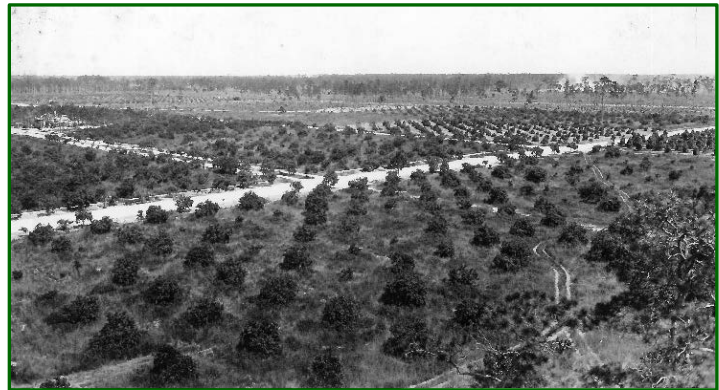
Figure 1: Streets in Coral Gables Under Construction, July 22, 1922
