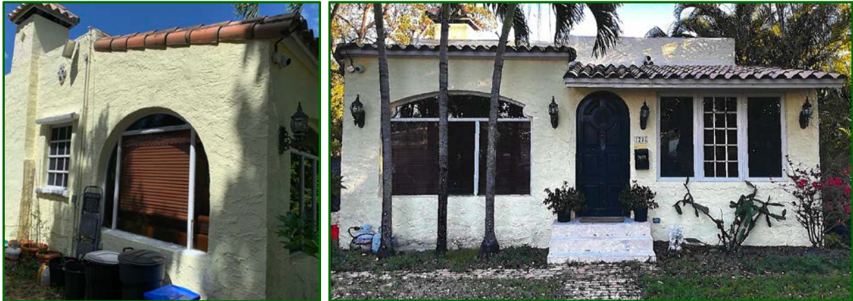
Figures 21: Front (South) Façade [right] Courtesy of Owner Note: porch enclosure extends beyond the east façade of the original home Southwest Corner, Arched Opening of Original Screened Porch, 2022 [left]
