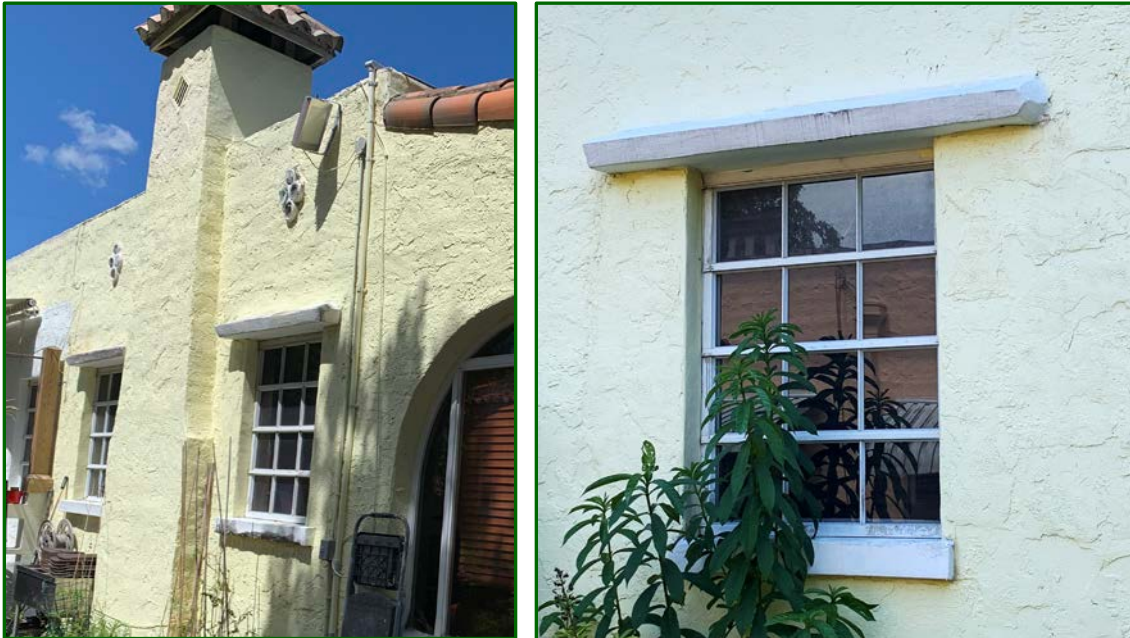
Figures 25: Flared Hoods Feature Over Windows, 2022 West Façade [left]; Lintel Detail, East Façade [right]
