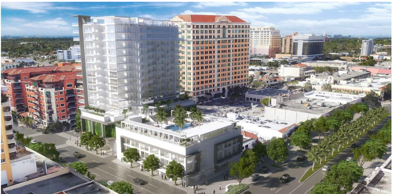
Proposed project and existing conditions
